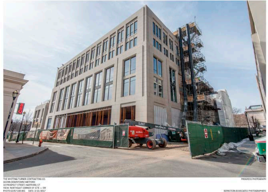
Construction on the Hartford Times Building looking northwest up Arch Street
