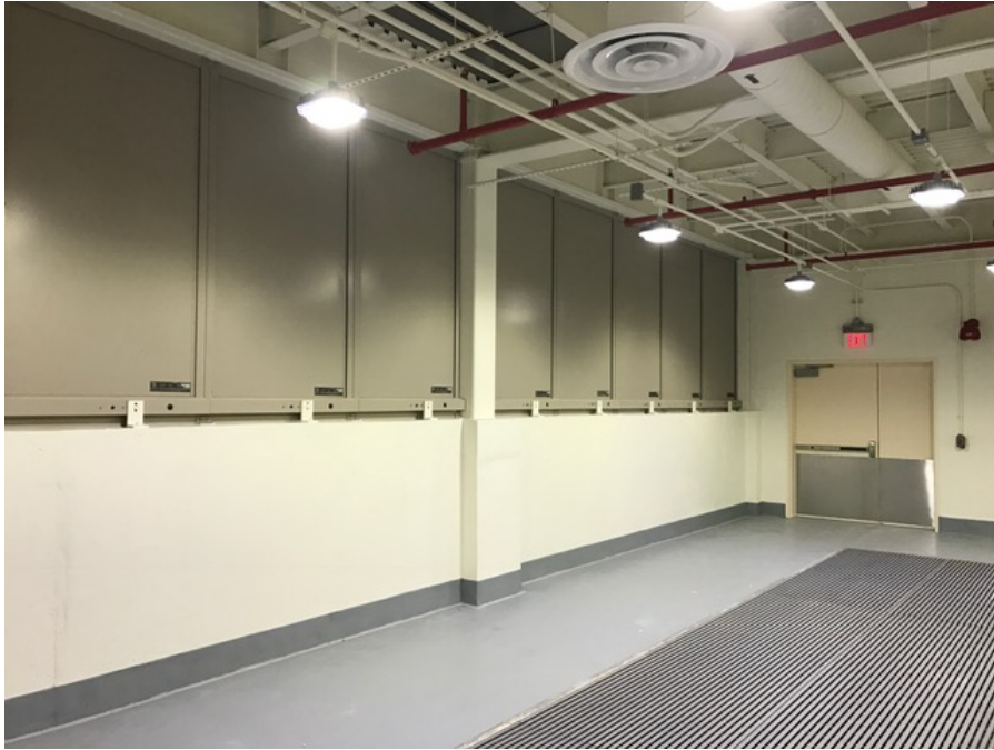
Chemical Storage Room with Blast Panels on Exterior Wall
