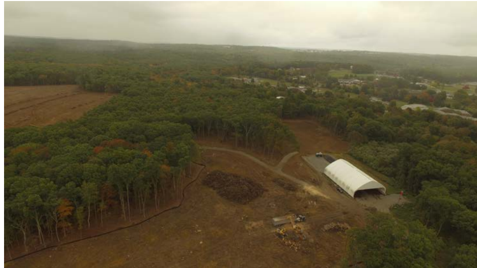
Farmland Restoration in Progress
