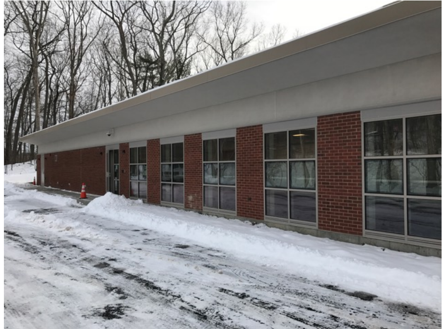
East Elevation View of MAA Facility
