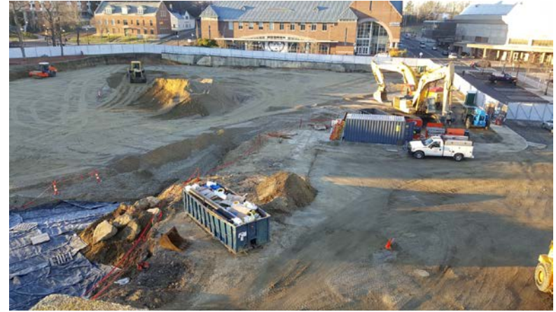
Site Prep for Upcoming Building Project
