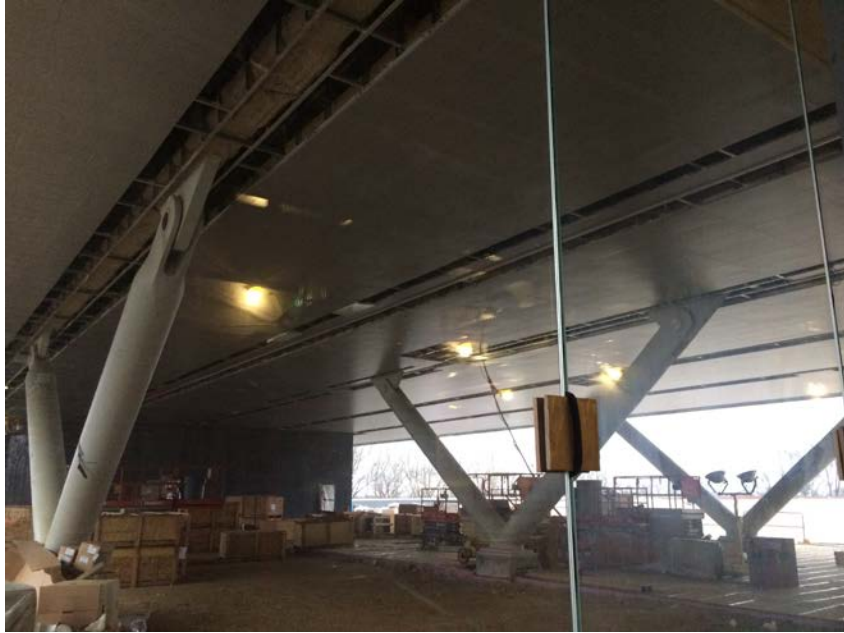
Ceiling View of Terrace Area Below Lab Bar
