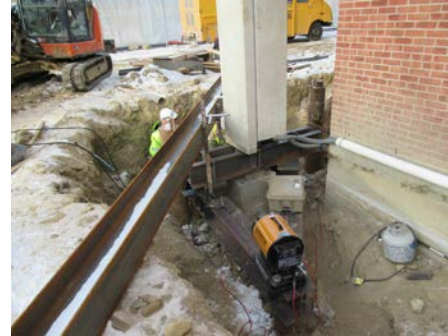
Caisson Repair – UTEB Building
