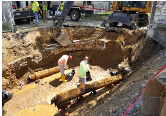
Abatement and removal of existing failed utilities
