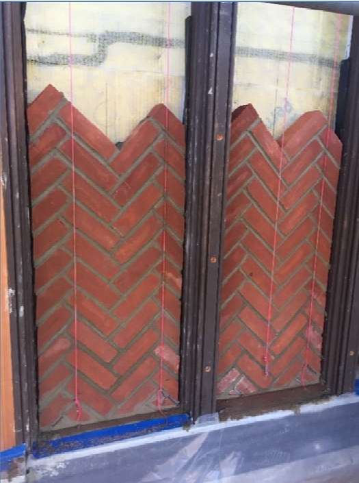
Herringbone Brick on North Elevation
