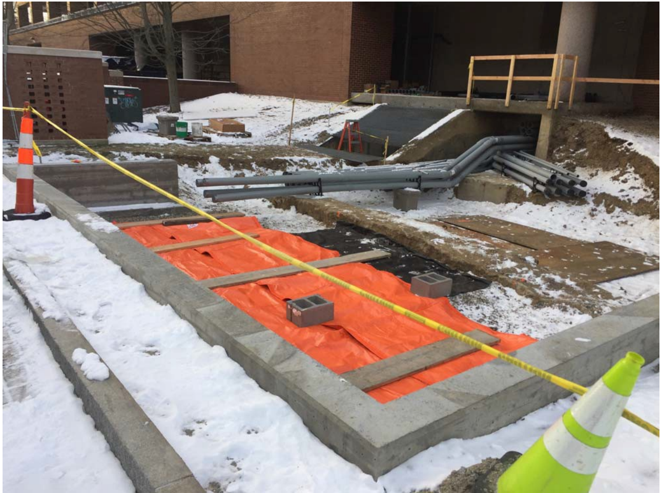
Babbidge Exterior Transformer Locations
