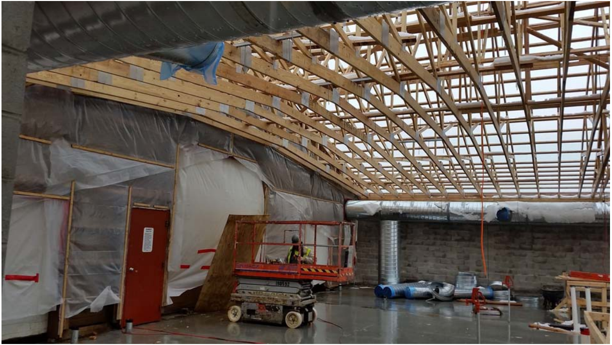
Trusses in new barn addition
