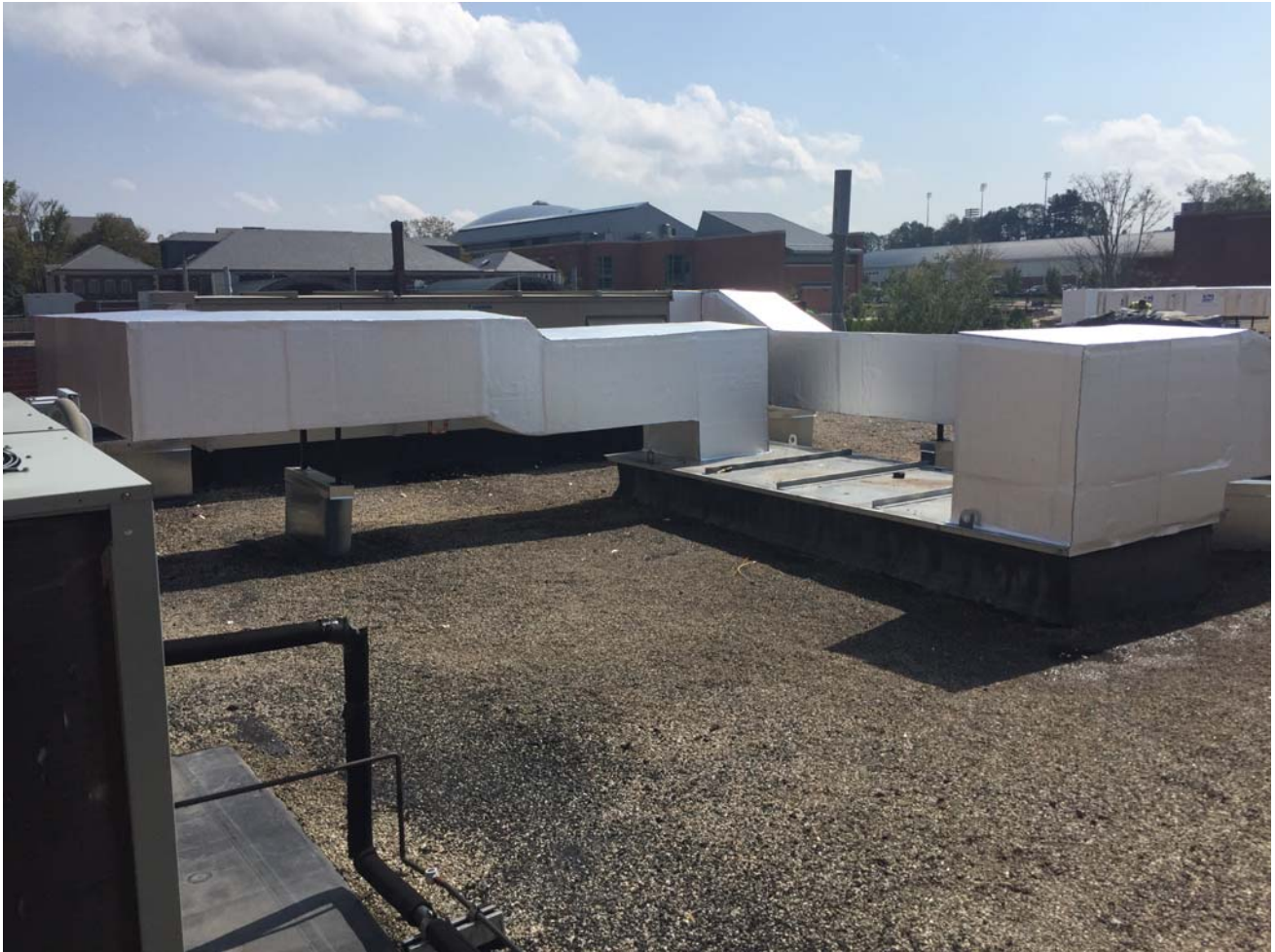
E-2 Rooftop Units
