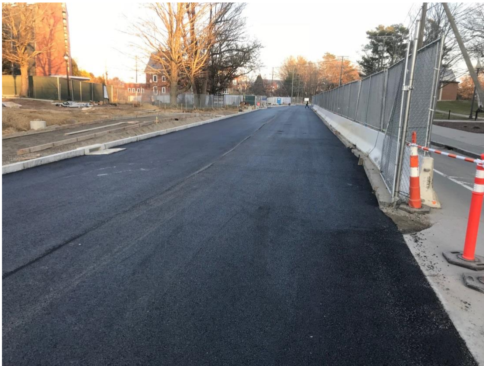
Binder Course of Pavement in front of St. Thomas Chapel
