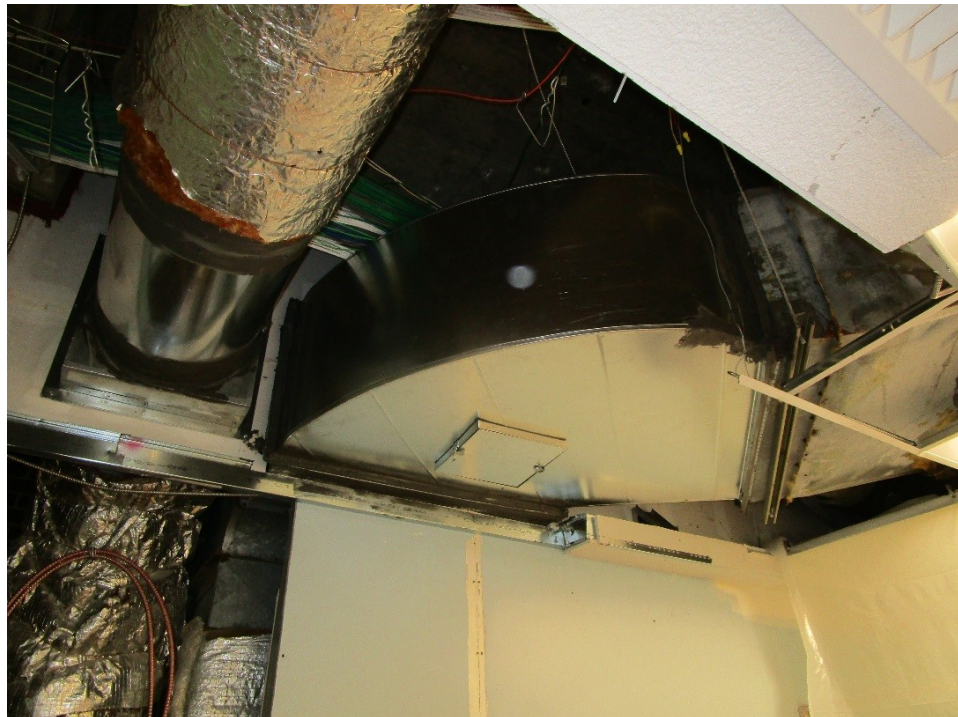
New Fire Dampers in Duct Work
