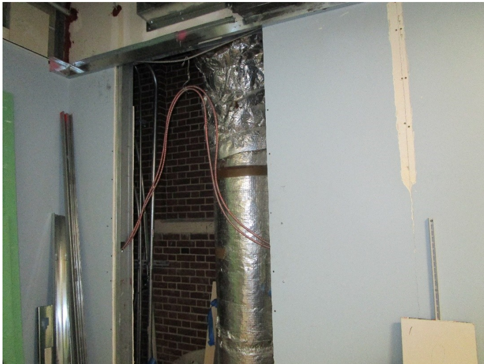
New Fire Rated Shaft Wall
