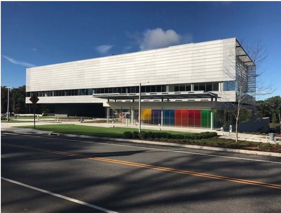
East Elevation View
