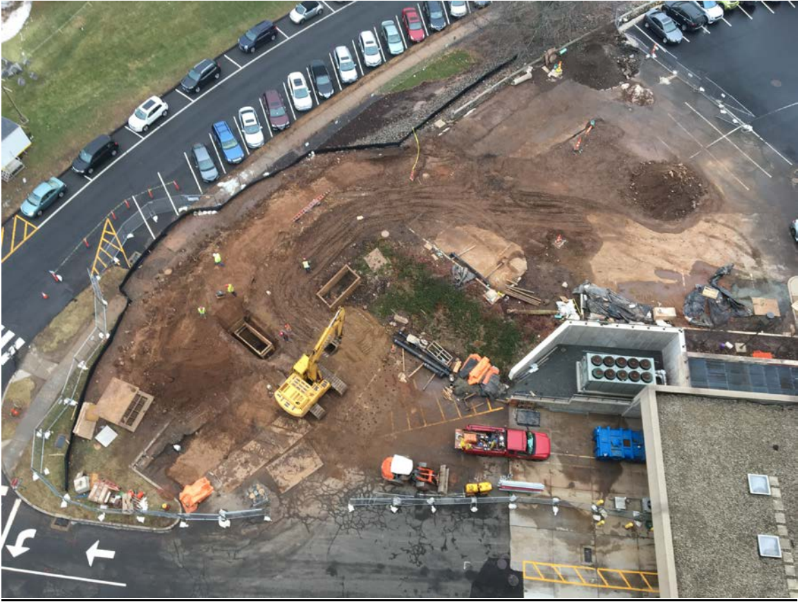
Relocation of water main nearing completion.
