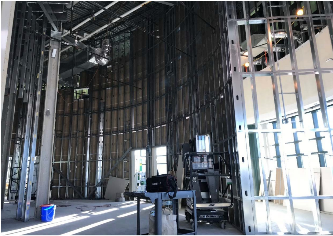
Dry wall framing in progress on the second floor
