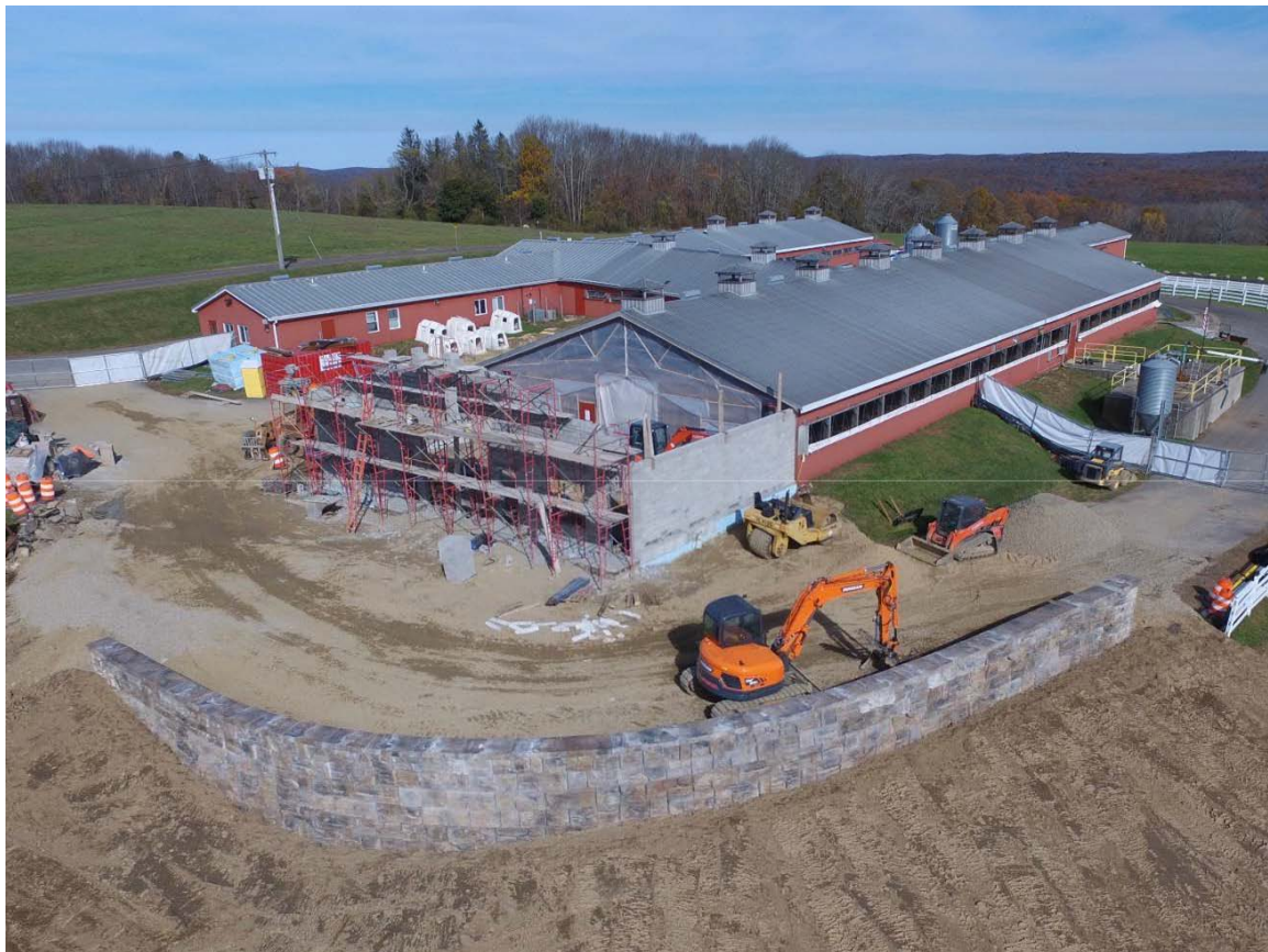
Kellogg Dairy Center – Aerial view of new retaining wall November 2017
