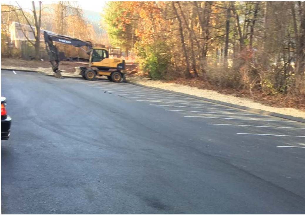
Sidewalk Site Beyond Excavator
