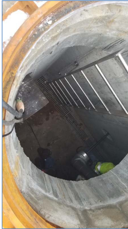
Crews providing temporary connections inside vault to Burton Family Complex
