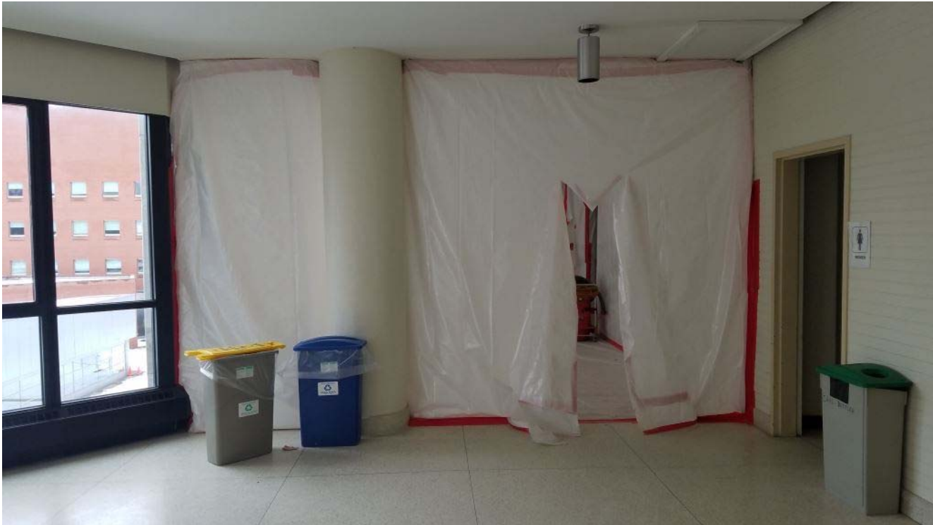
PCB Abatement Work and Containment
