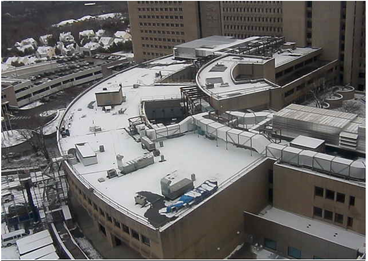
New Roof Substantially Complete
