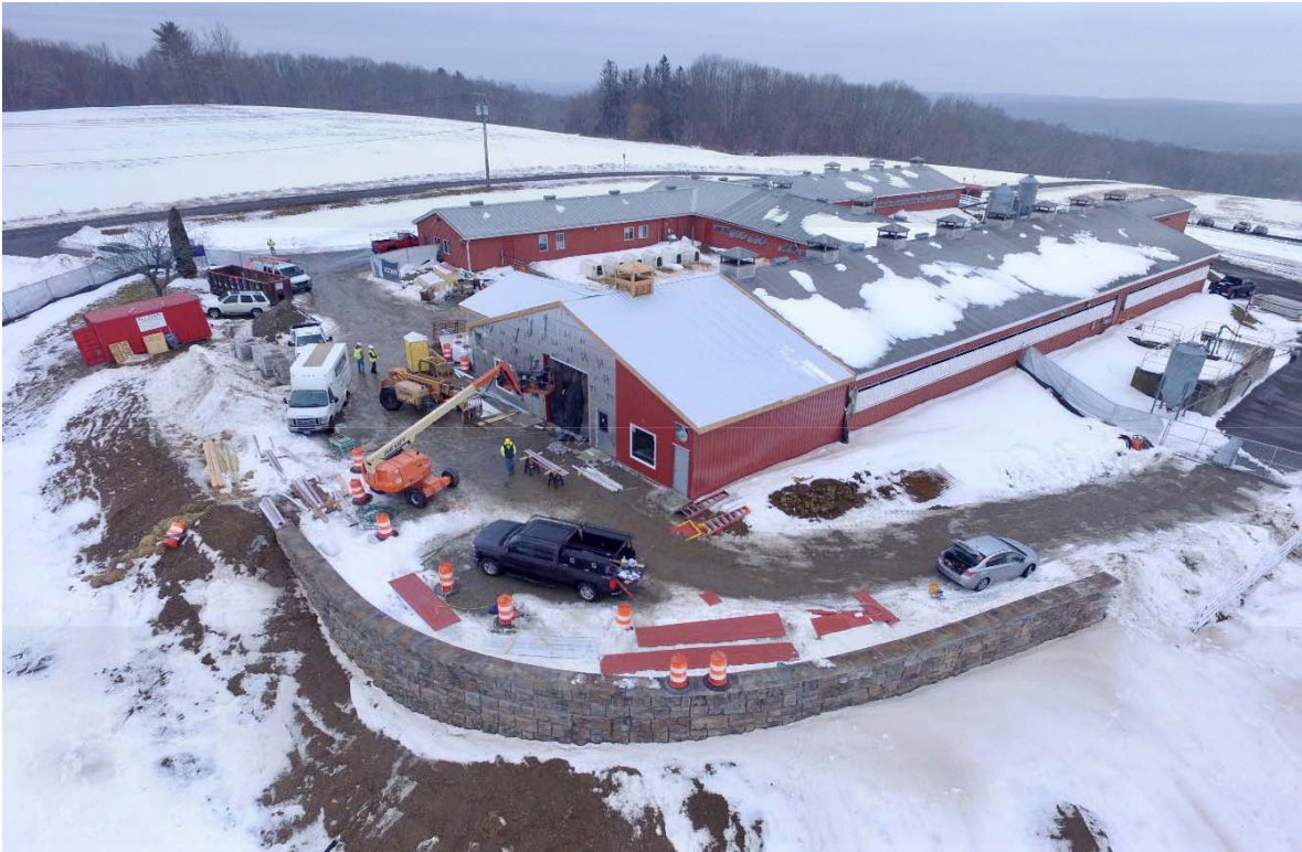
Kellogg Dairy Center – Aerial view of the site January 2018 (Photos by M. Levin- Levin Aerial Works)
