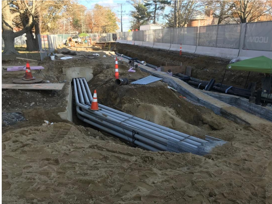
Underground Utilities in front of St. Thomas Chapel
