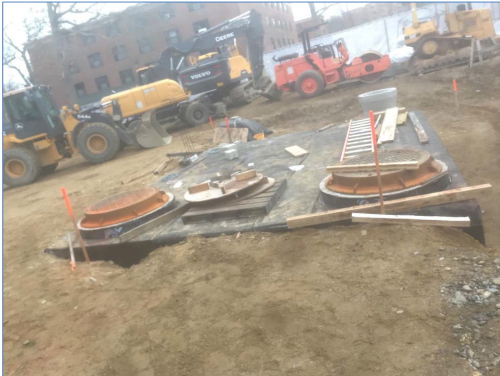
Vault D-7 waterproofed and ready for backfill
