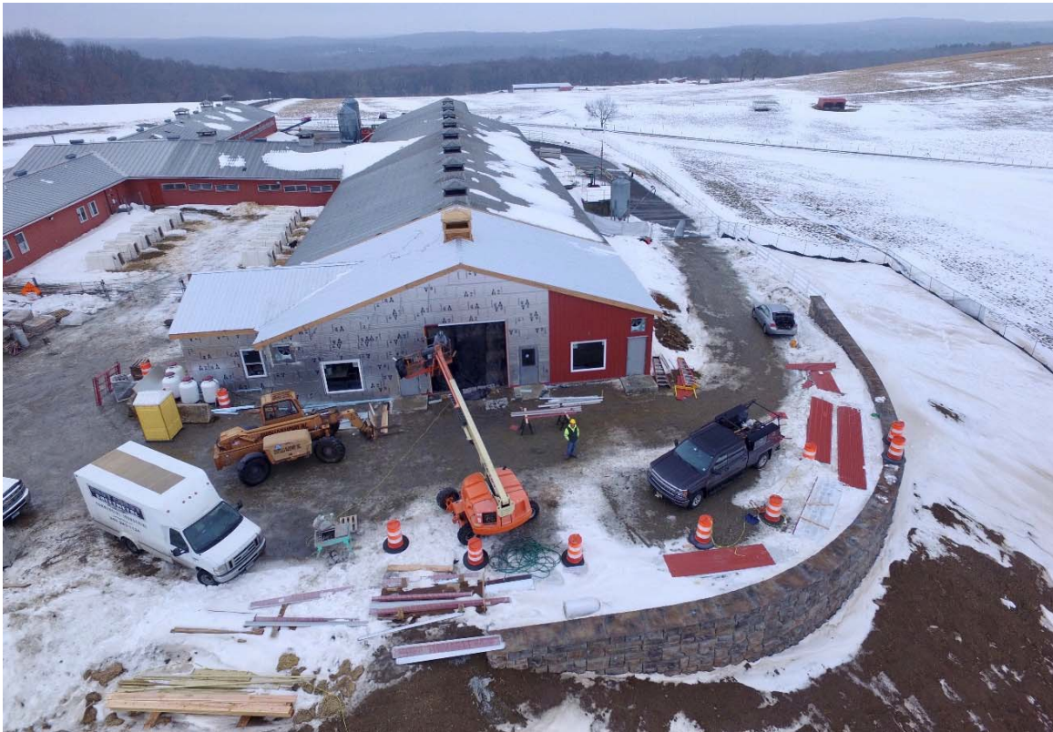
Kellogg Dairy Center – Aerial view of the site January 2018
