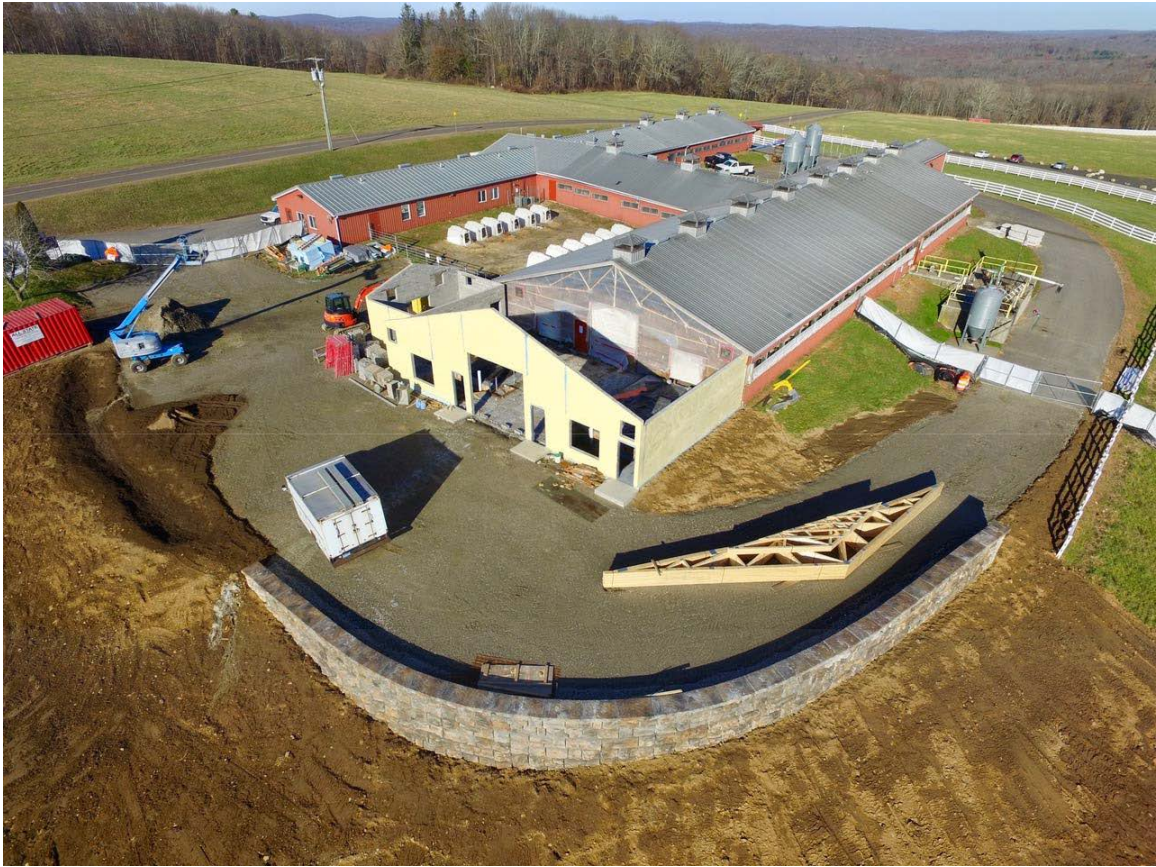
Kellogg Dairy Center – Aerial view of the site December 2017
