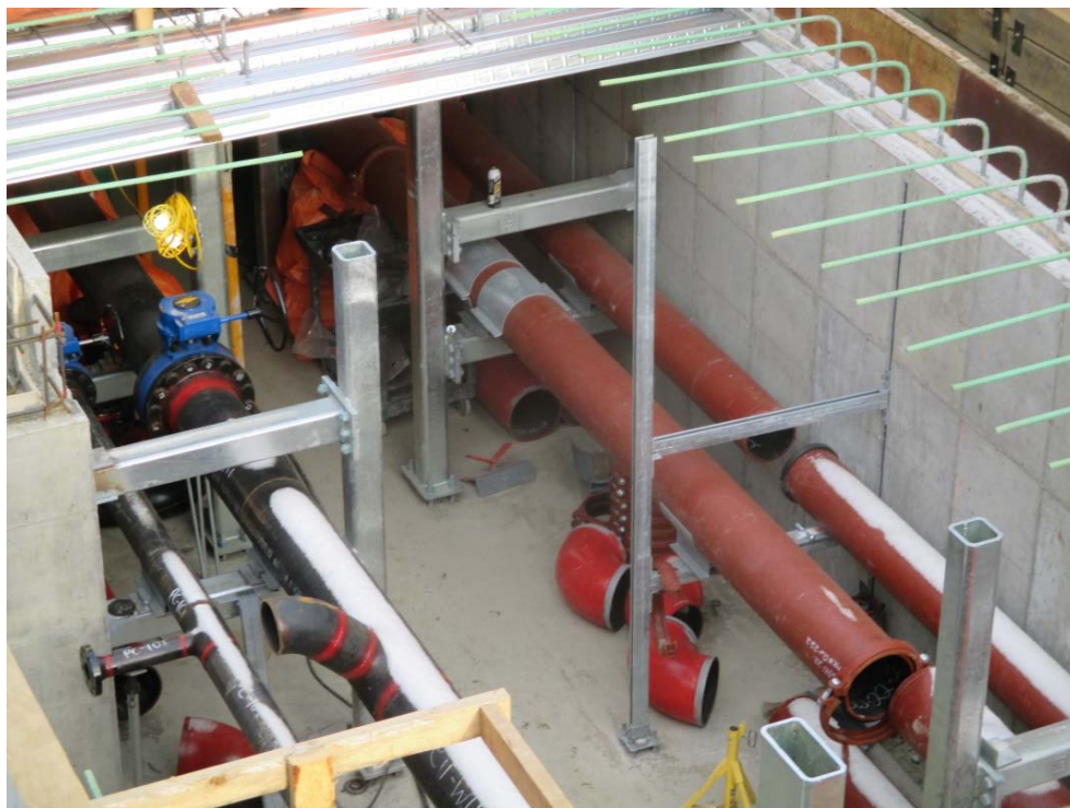
Installation of Tunnel Utility Piping
