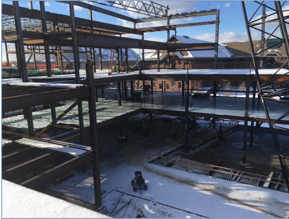
Elevated steel decks are underway, and steel is on schedule.
