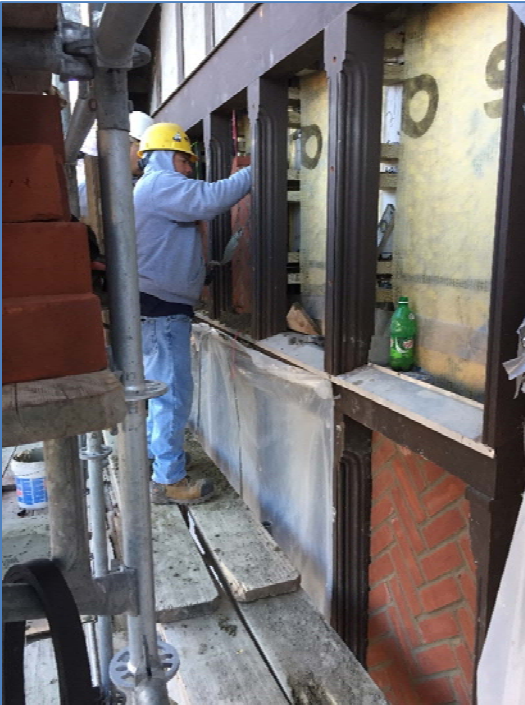
New wood columns
