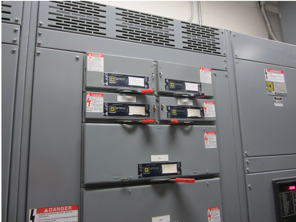
New Electrical Equipment
