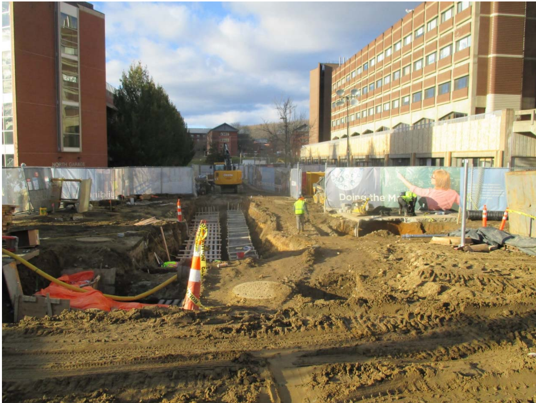
Tunnel Backfill and Electrical Ductbank Replacement
