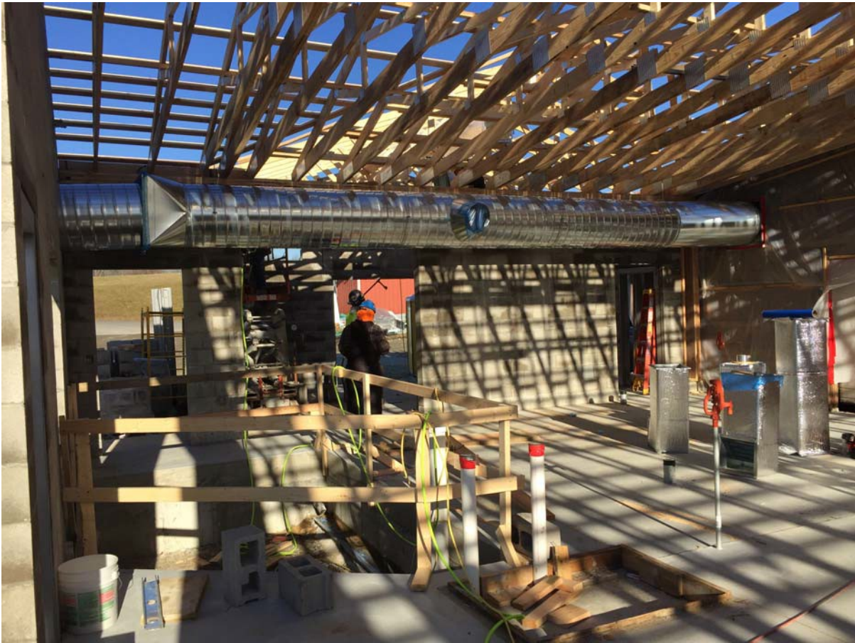
Mechanical ductwork in new barn addition
