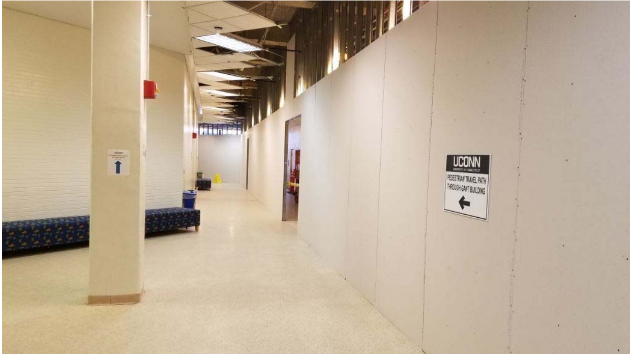
Installation of Temporary Interior Partition Walls and Directional Signage
