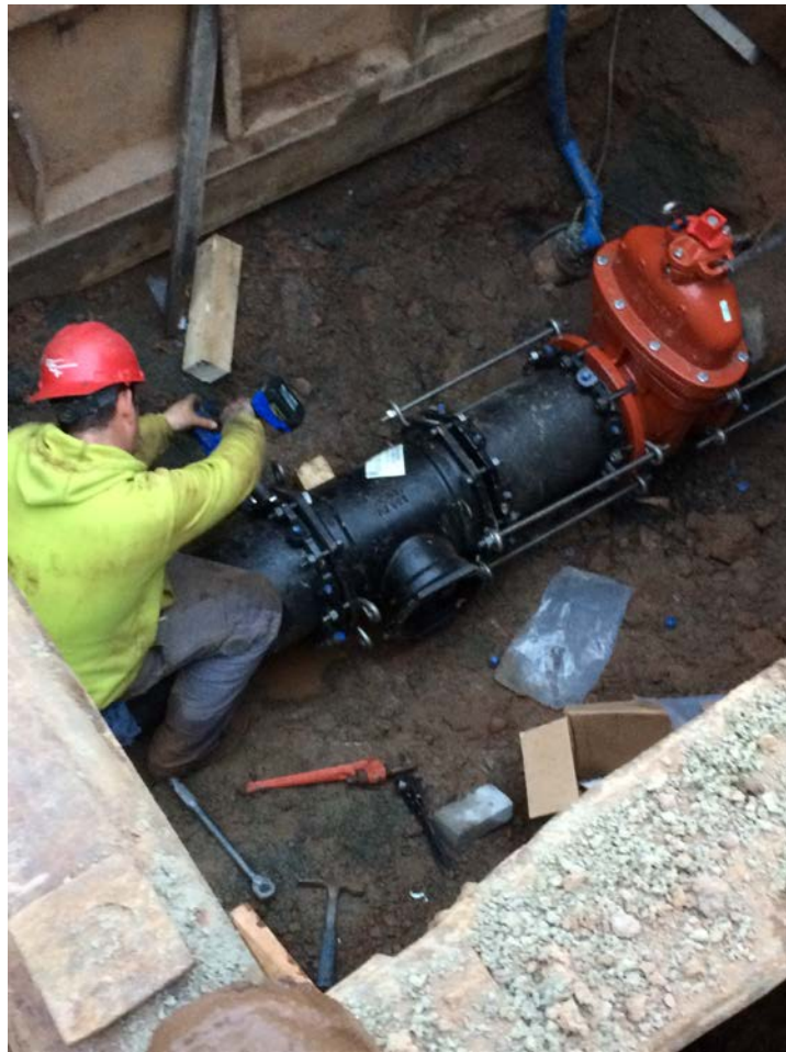
Water main gate valve, restraints and blow off installation
