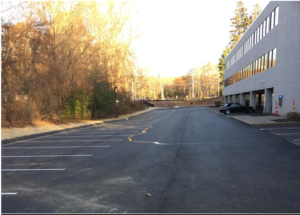
Finished Parking Lot West side
