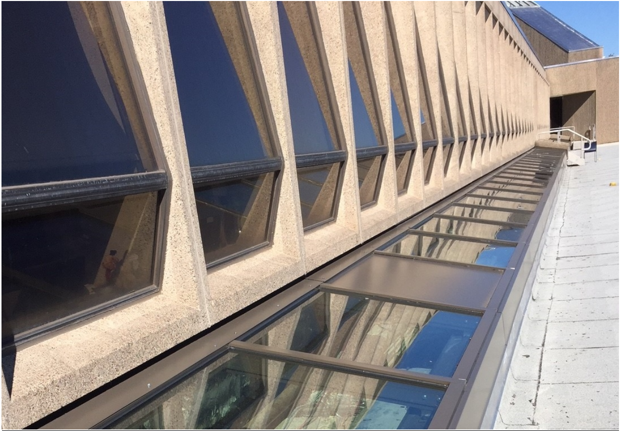
Completed Skylight Section
