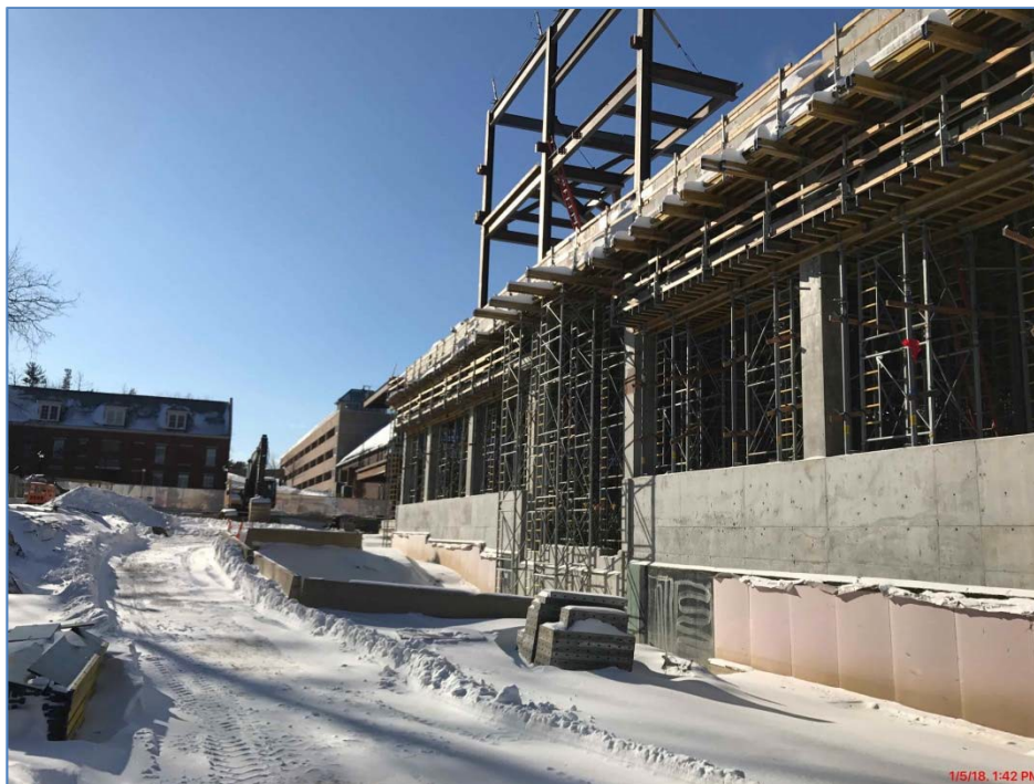
South building elevation outside of the pool structure. The start of the elevated track can be seen at the top of the photo.
