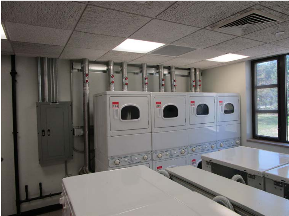
New Venting at Laundry Facility
