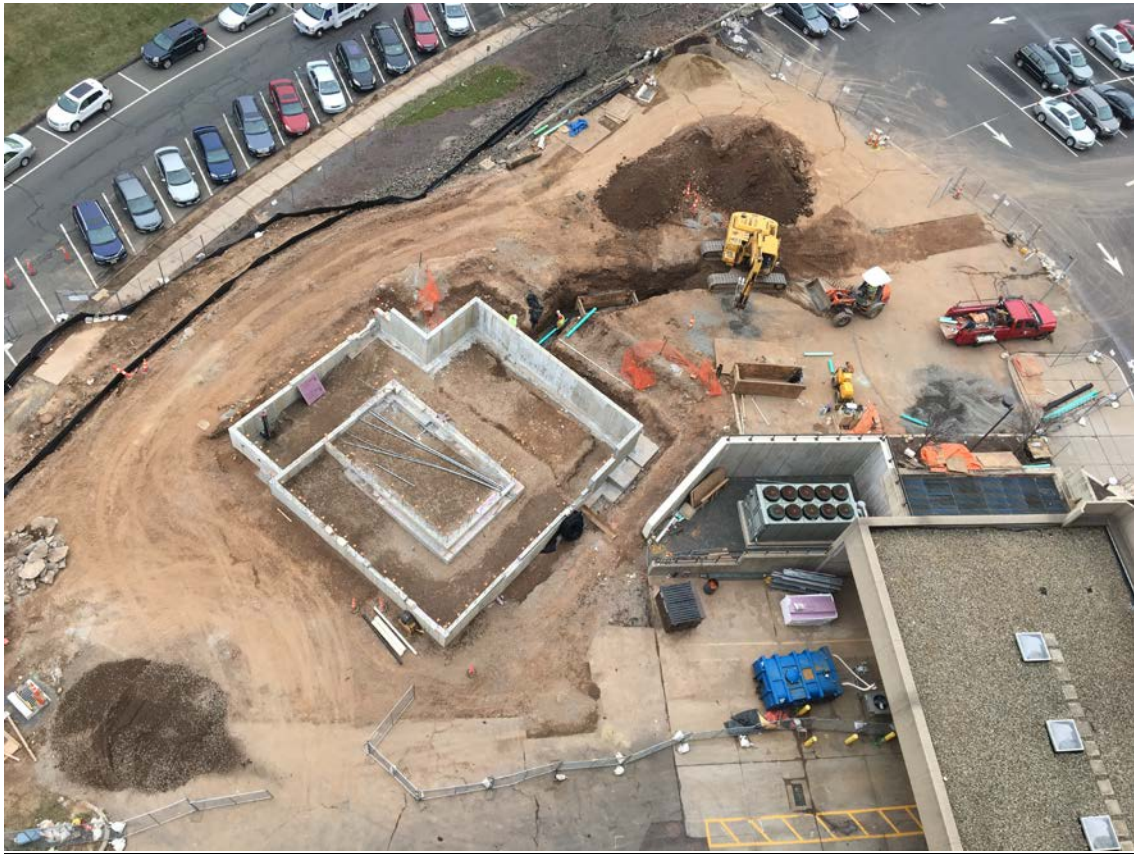
Building foundation and installation of sewer line.
