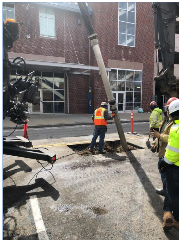
Vacuum truck utilized to limit test pit impacts
