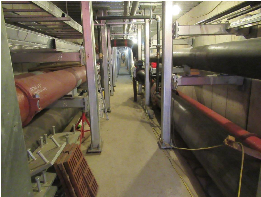
Installation of Tunnel Pipe and Support System
