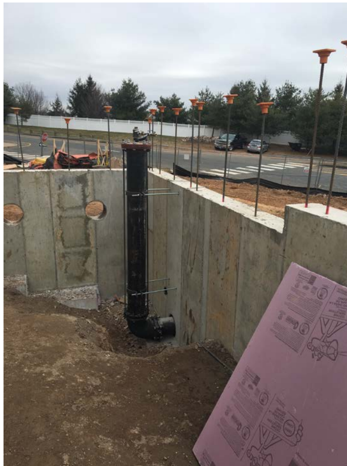
Sprinkler main entering the building
