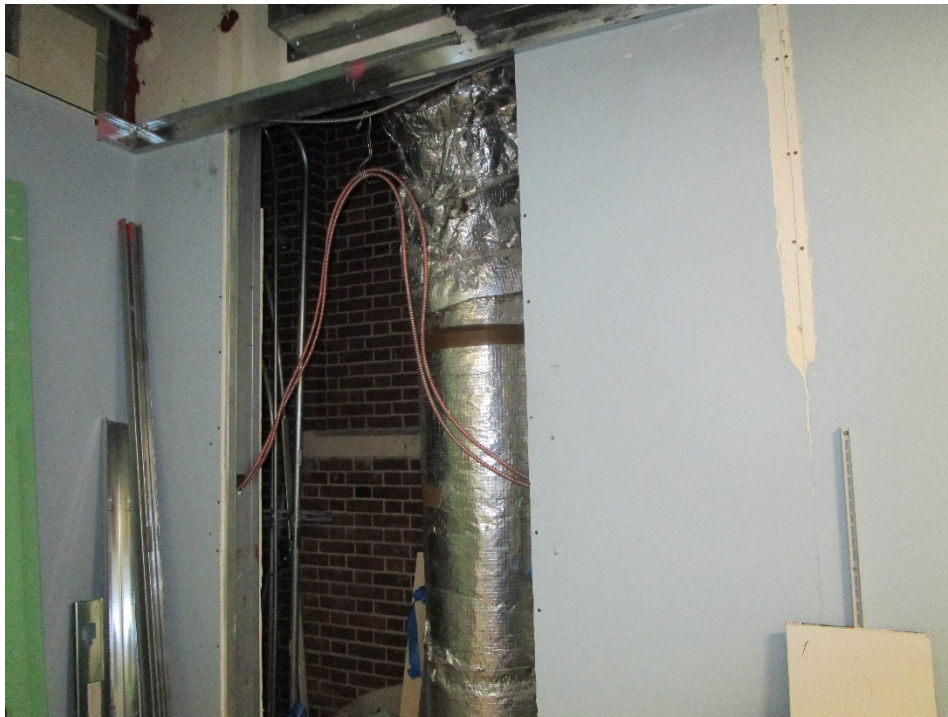
New Fire Rated Shaft Wall
