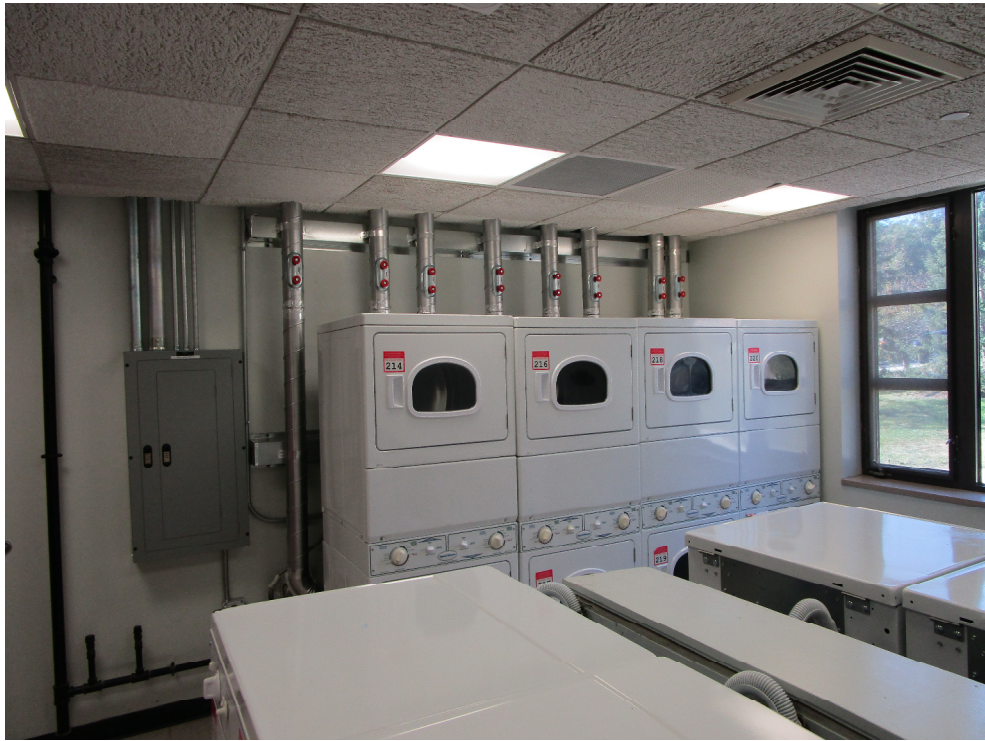
New Venting at Laundry Facility
