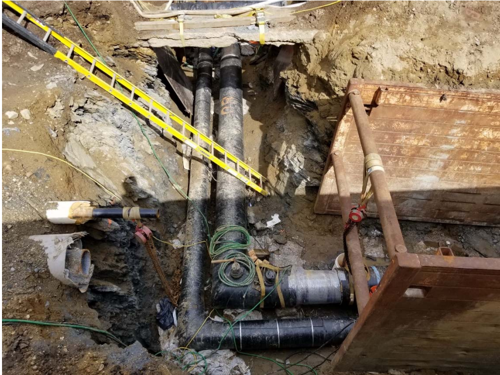
New Steam Lines From North to Atwater
