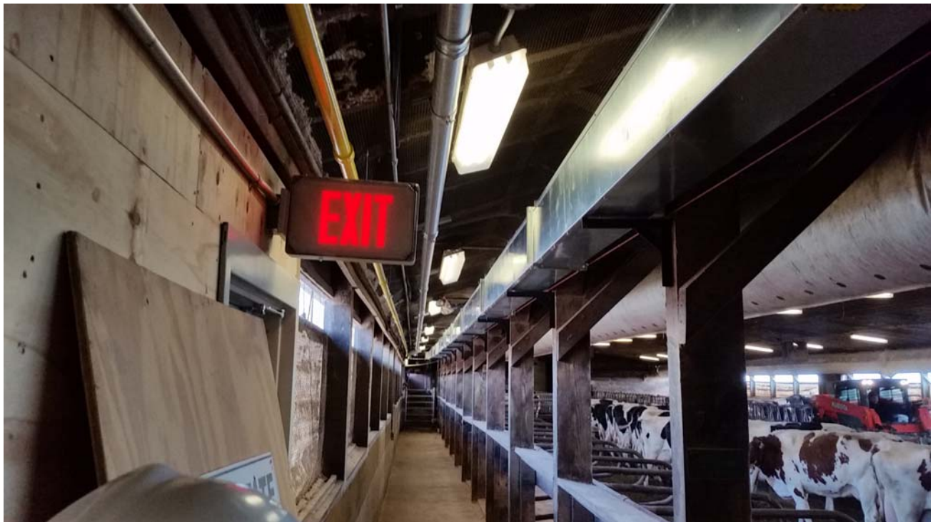
Kellogg Dairy Center – pedestrian aisle in existing barn with new trough for milk lines
