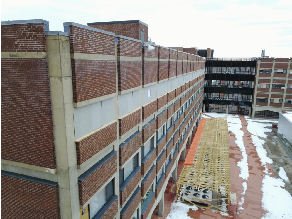
Installation of Temporary Protection for Data Center HVAC Condensers
