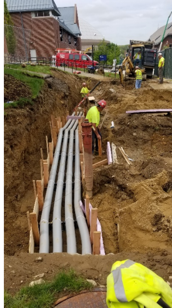
Duct Bank Installation
