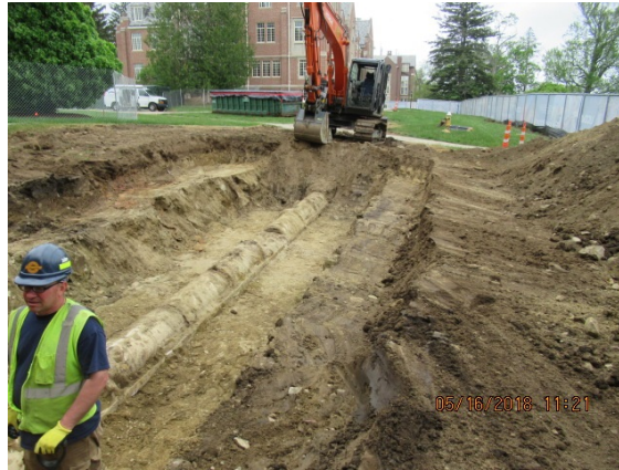
Excavation of existing steam line
