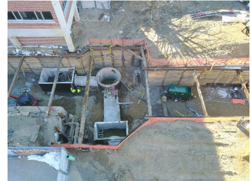
48 inch diameter storm drain relocation at tunnel intersection
