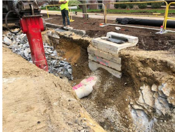
Ledge excavation for new water line installation adjacent to existing storm drain and catch basin
