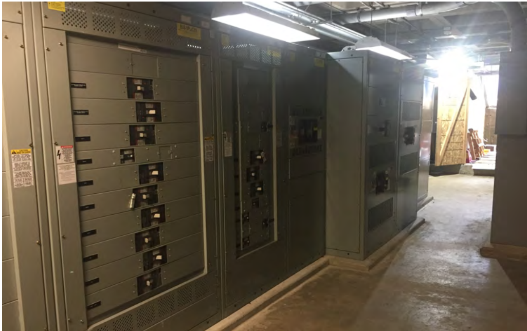
New switchgear in place
