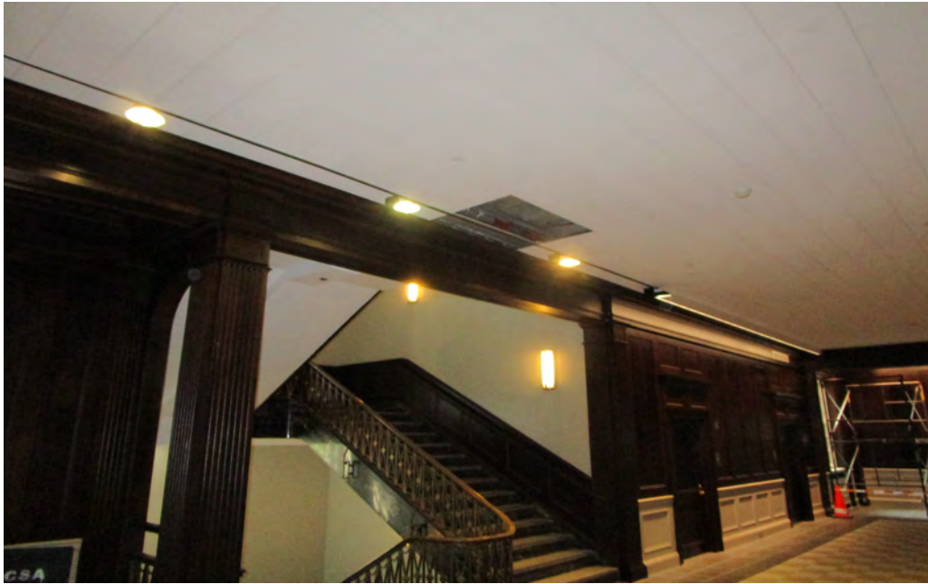
Installation of Smoke Curtain and Sprinklers
