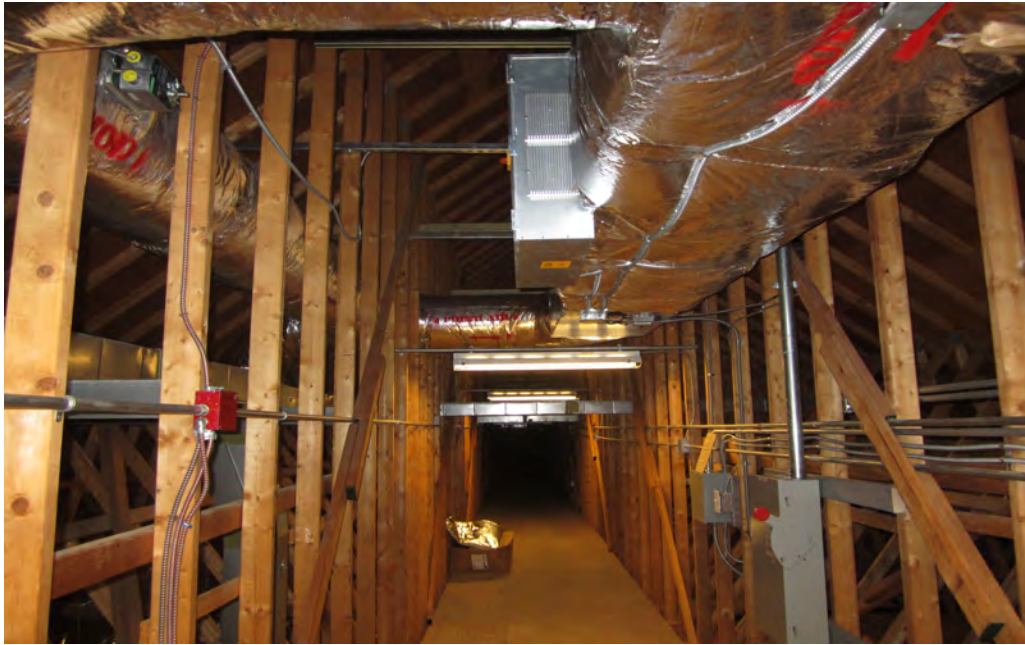
New Mechanical Equipment in Attic
