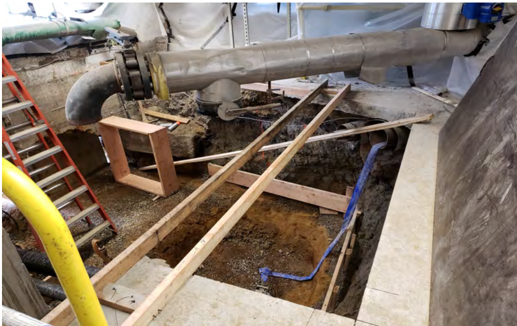
CUP Building- interior protection & floor trench/pit
