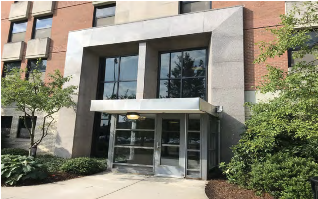
Re-anchored granite at Eddy Hall
