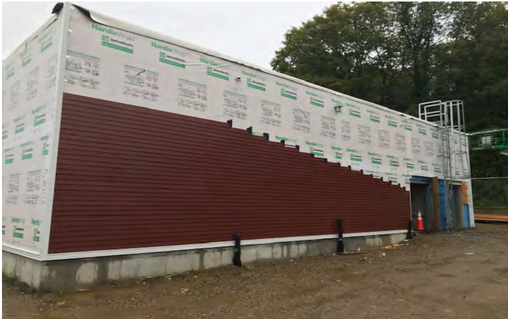
East Exterior Side of Building
