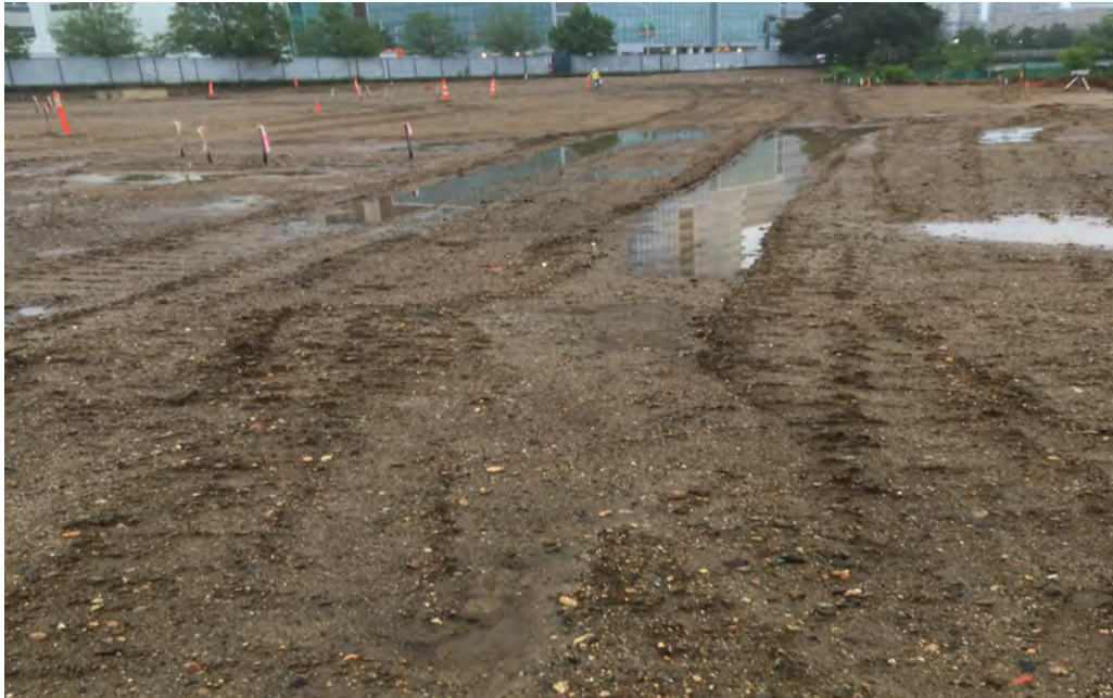
Phase 1 site area cleared and contaminated soils removed.
