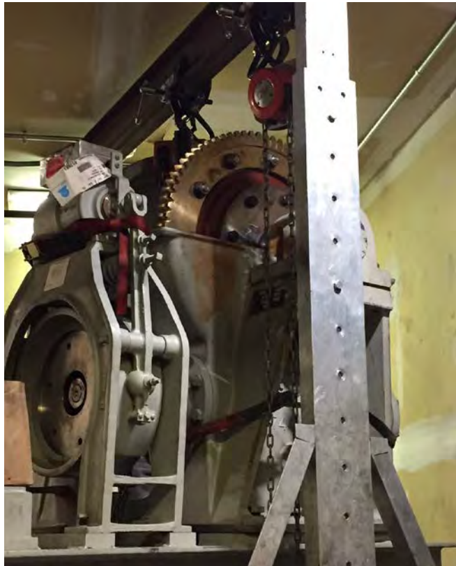
New motor being assembled in the elevator Machine room
