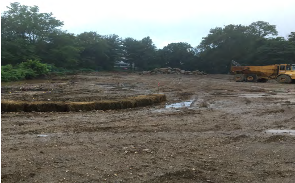
Rough Grading in preparation for Surface Lot
