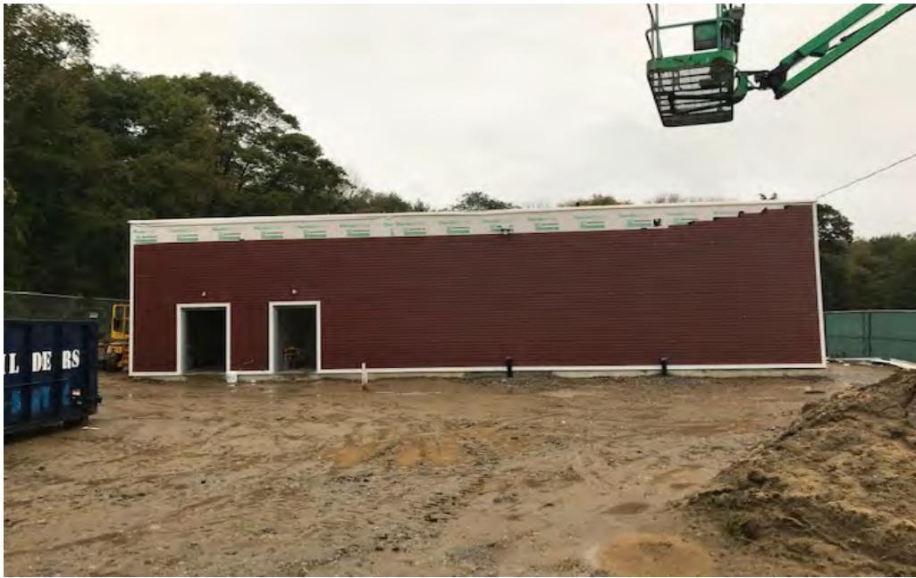
West Exterior Side of Building
