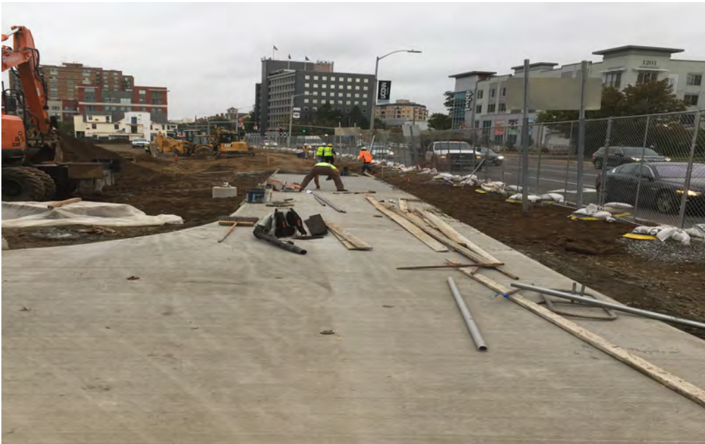
Washington Blvd Sidewalk Replacement
