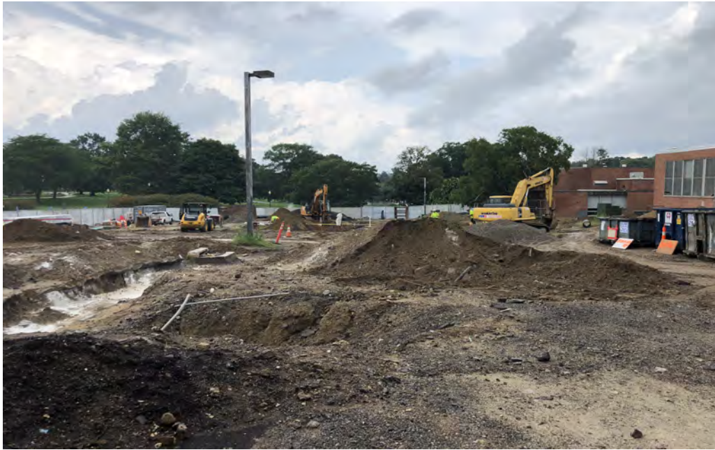
Site excavation/installation of site utilities
