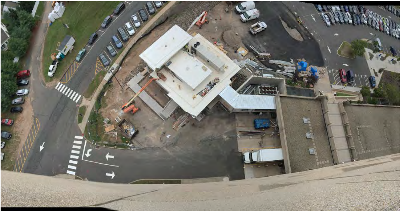
Ariel view of building
