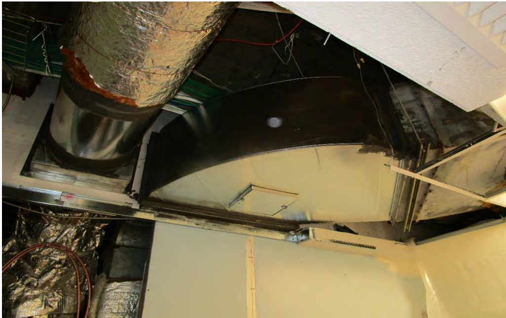
New Fire Damper in Duct Work
