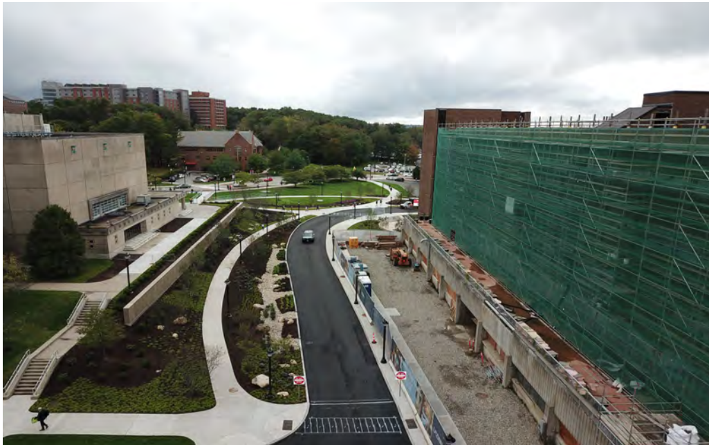
Completion of Final Landscape - Viewing West
