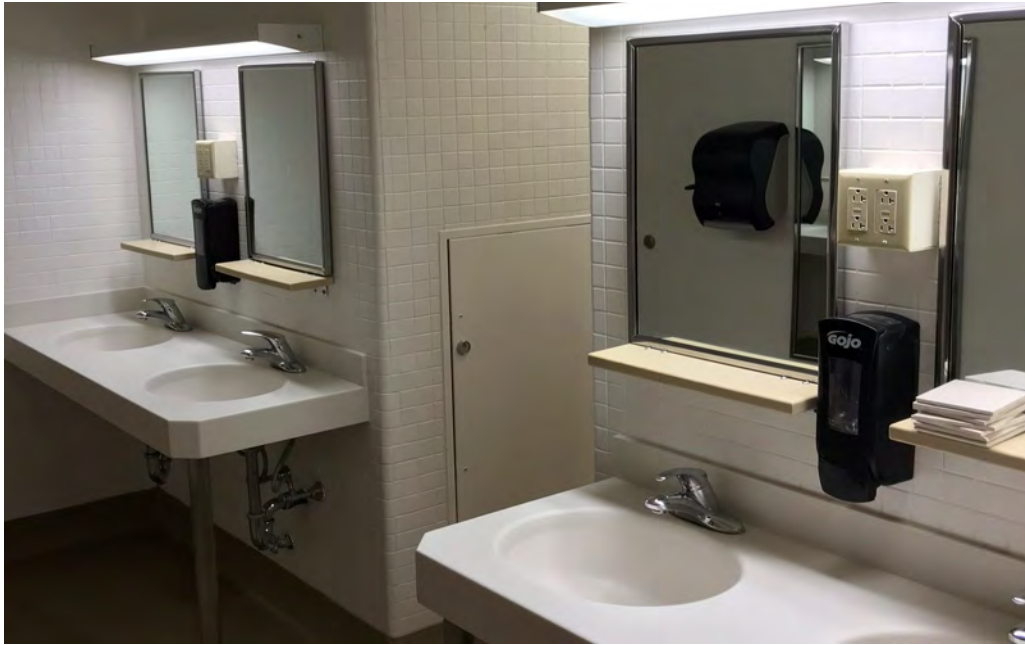
Sink Area Completed
