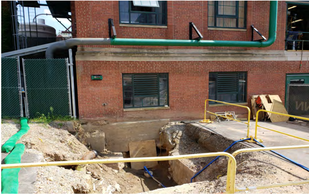
Central Utility Plant - Exterior VAULT 304 pit
