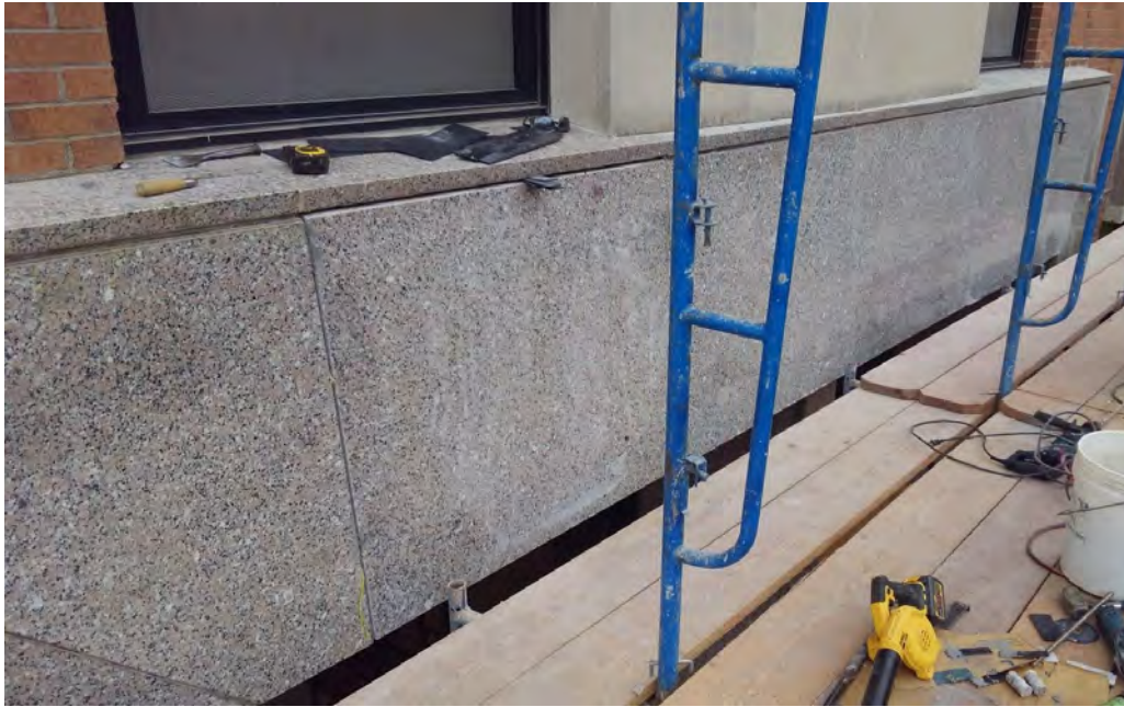
Granite panel installation
