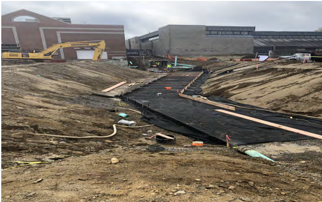
Construction of new tunnel
