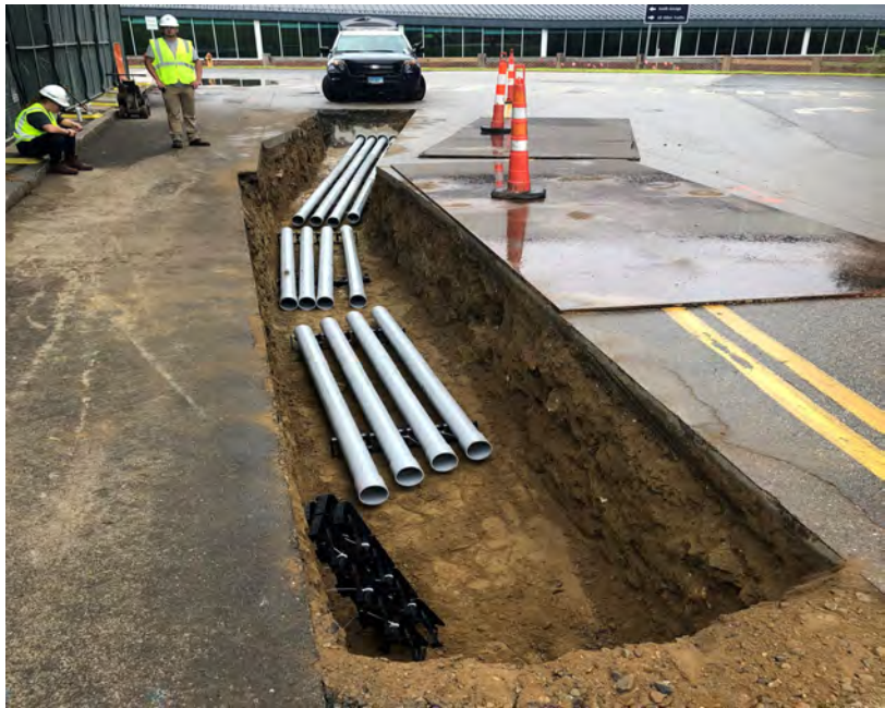
Alumni Drive - Electric Ductbank Installation
