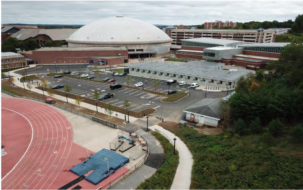
Overall View of Parking Lot - Looking South
