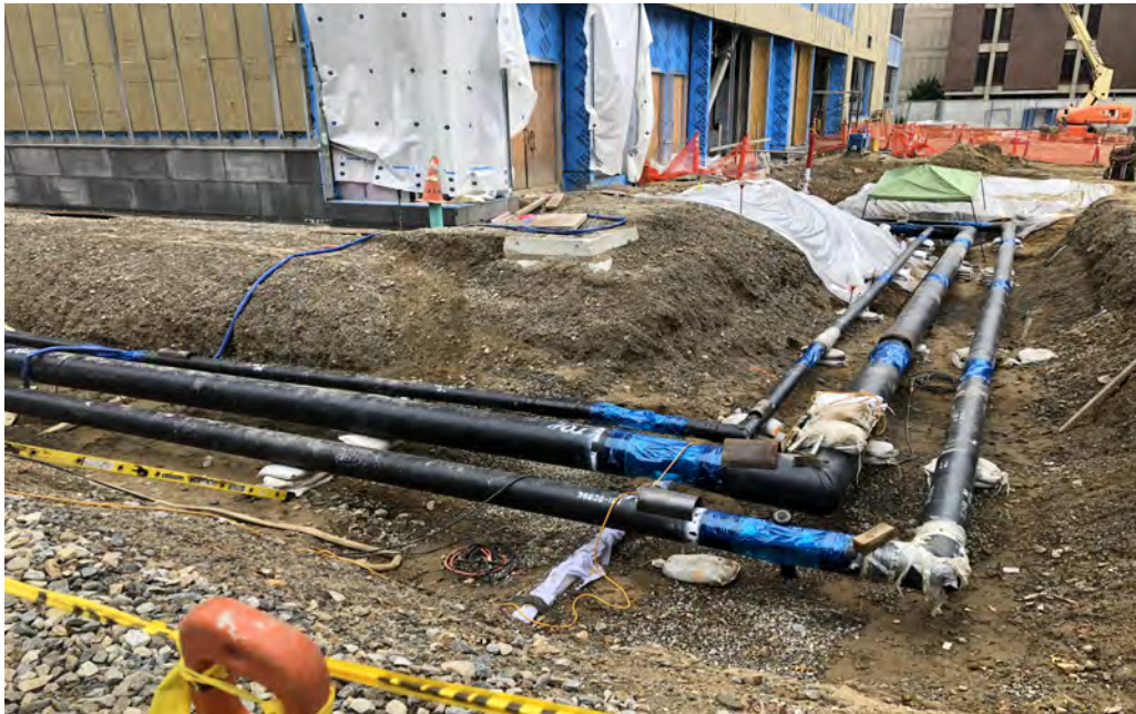
Last sections of Phase 2 Steam piping
