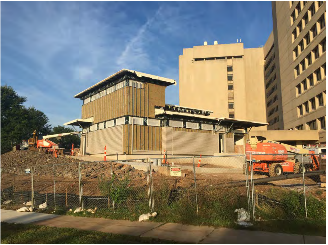
Installation of building metal skin exterior walls is in progress
