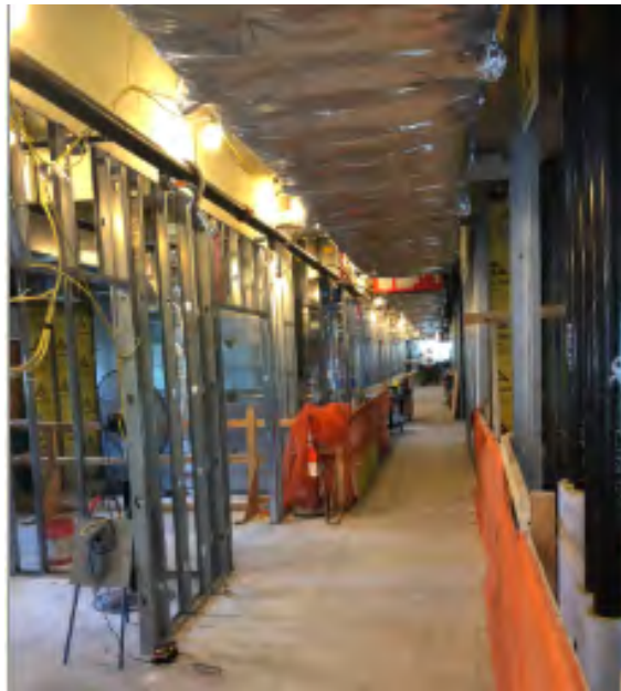
Fourth Floor Framing and MEP Rough-in
