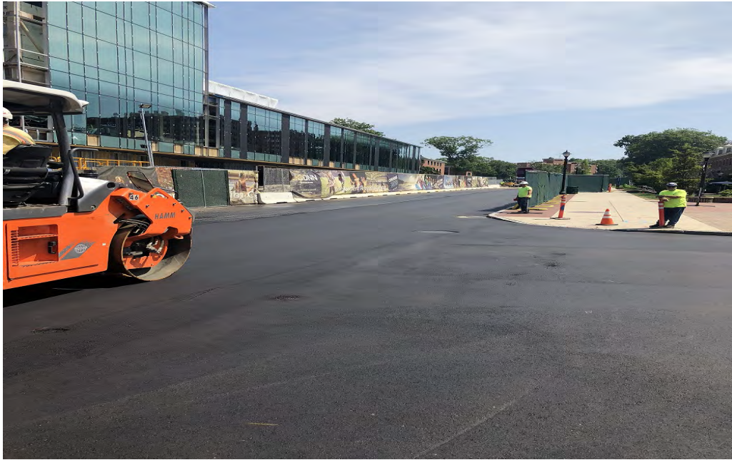
View of final paved Hillside/Jim Calhoun Way intersection
