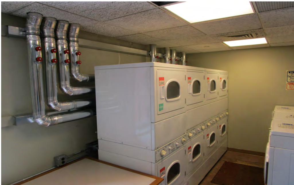
New Code Compliant Venting on Dryers
