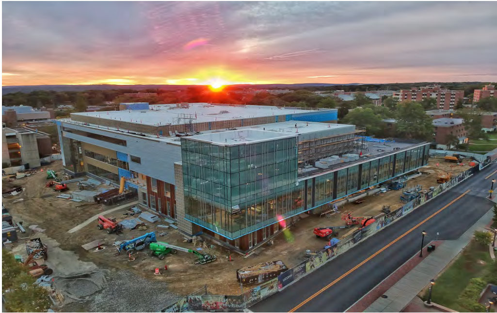
View of Hillside Elevation
