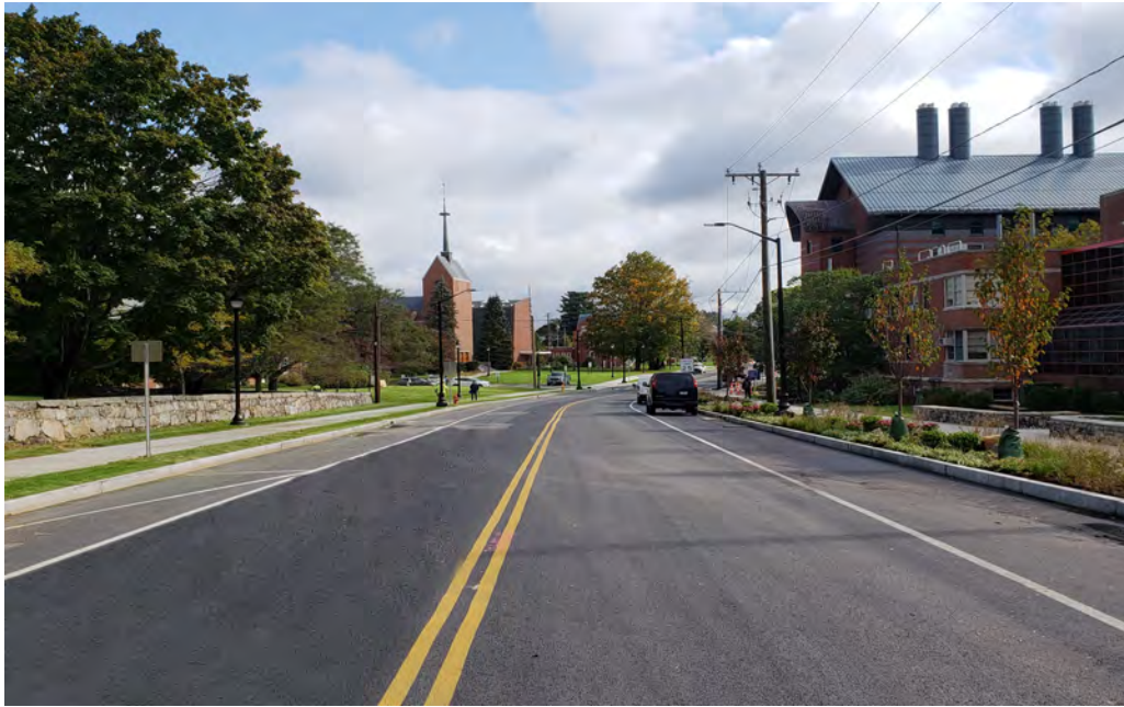
#1 NER 3B - Binder complete and landscaping is in progress.
