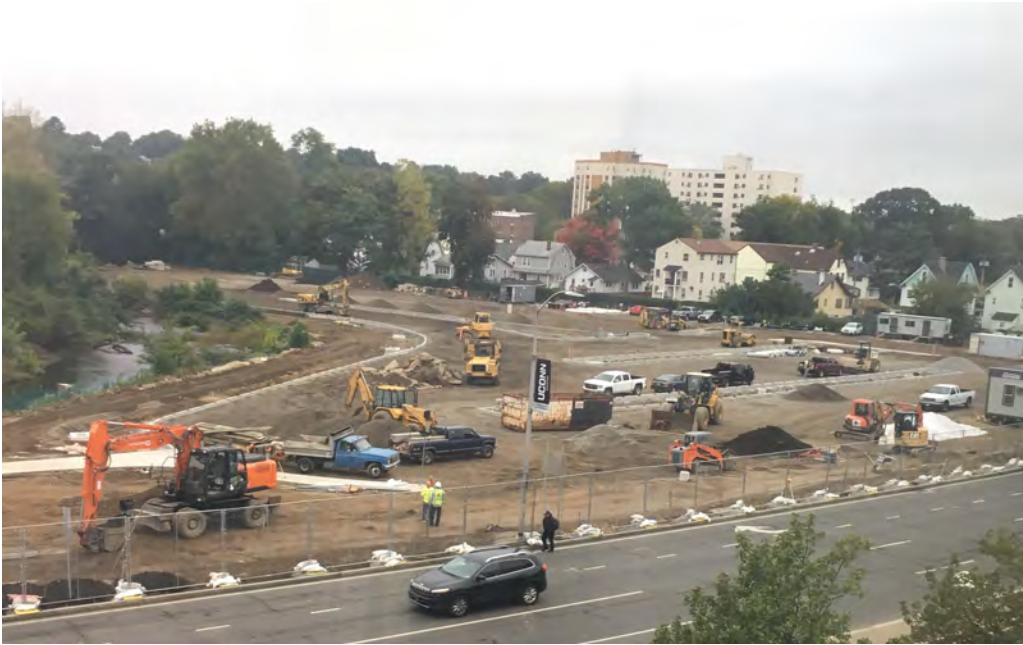
Site Progress Through October 10, 2018
