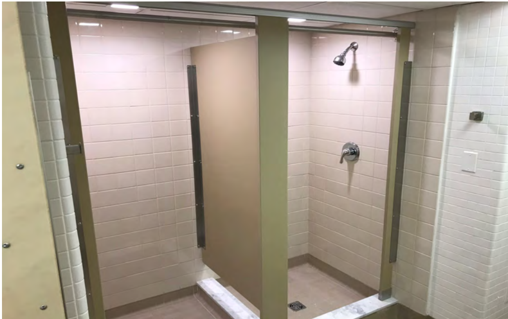
Shower Compartment Completed
