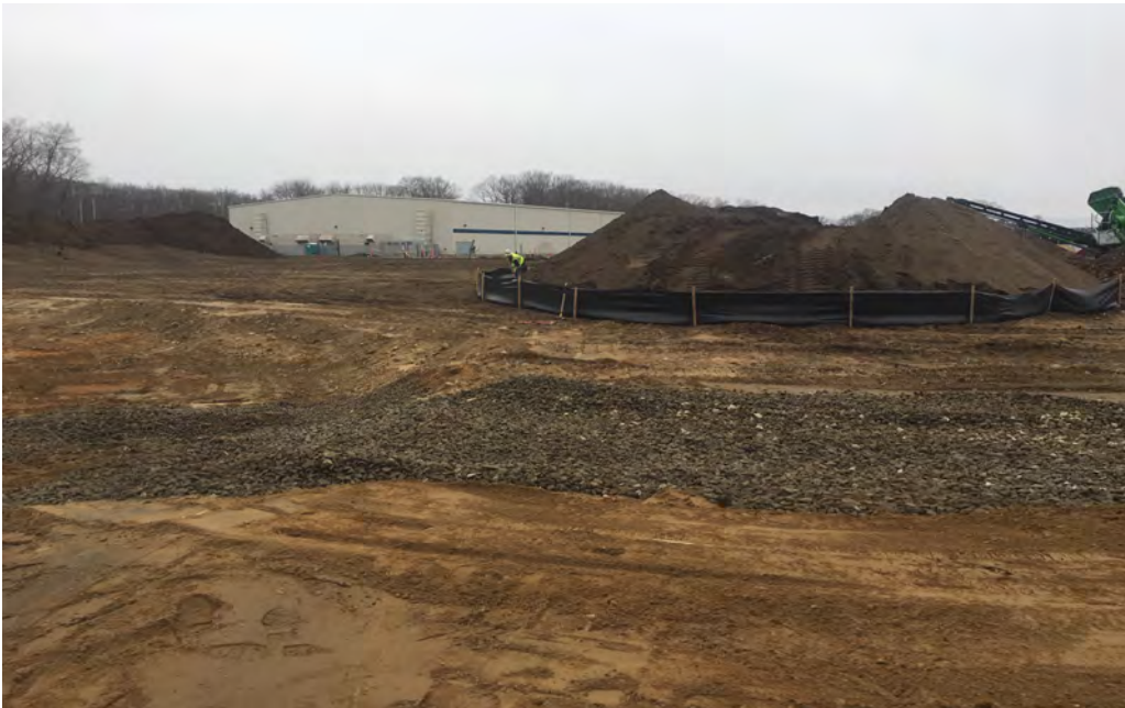
Top soil with silt fencing
