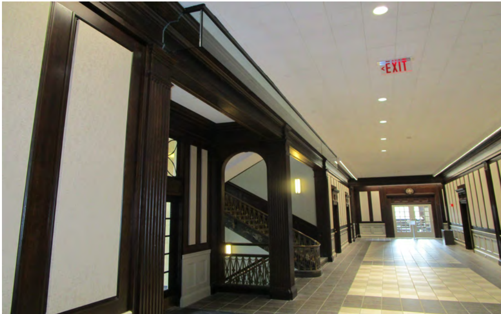
Completed Smoke Curtain
