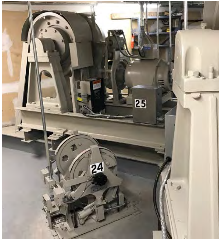
New motor, clutch and Safety brake assemblies in the elevator machine room
