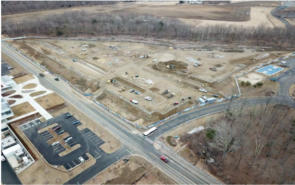
Parking Lot progress looking to the Northwest (March 2019)
