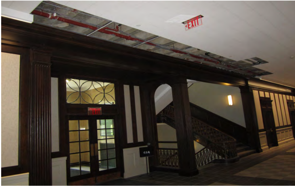
Installation of Smoke Curtain and Sprinklers
