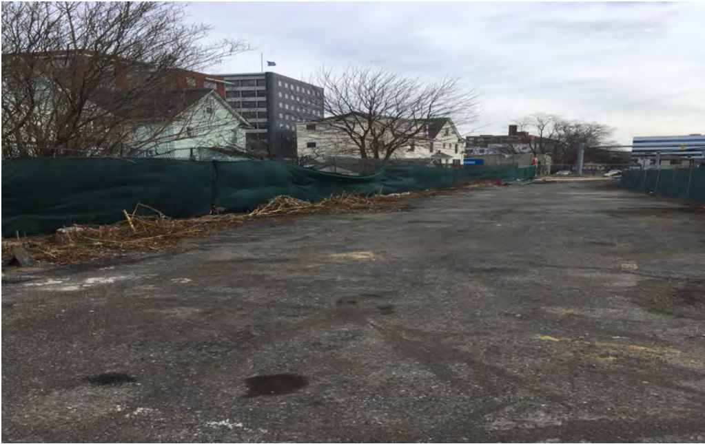
Pending-Phase 2 Site Area Looking East
