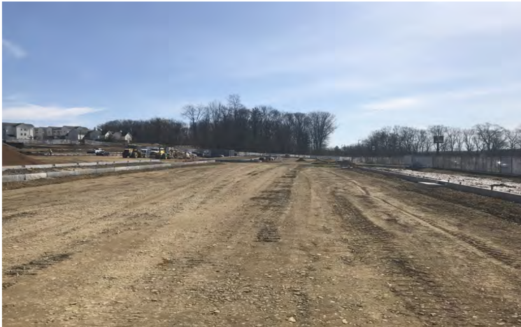
Western parking bay ready for pavement base (April 2019)
