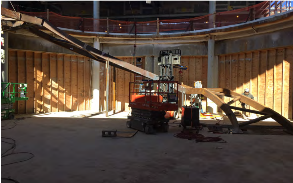
New steel frame work for Plaza Building light court stairs.
