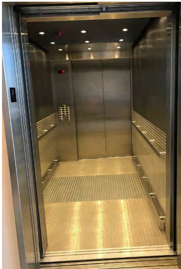
New completed elevator cab
