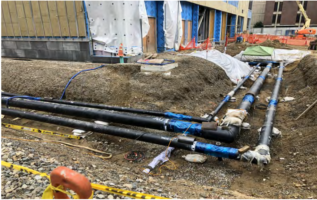
CCIU Steam looking north
