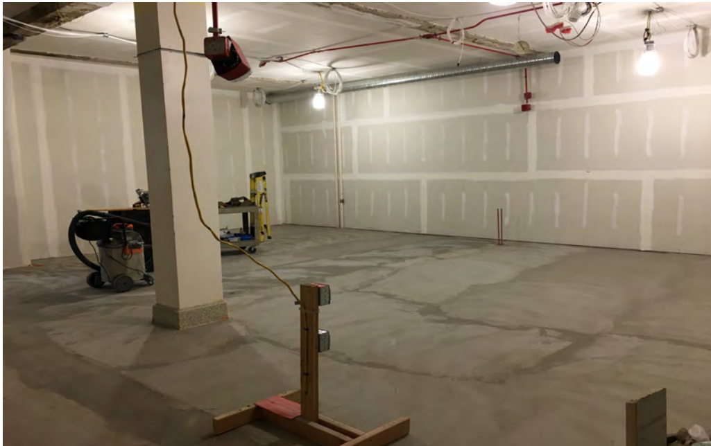
Clean room shell space, awaiting panel system
