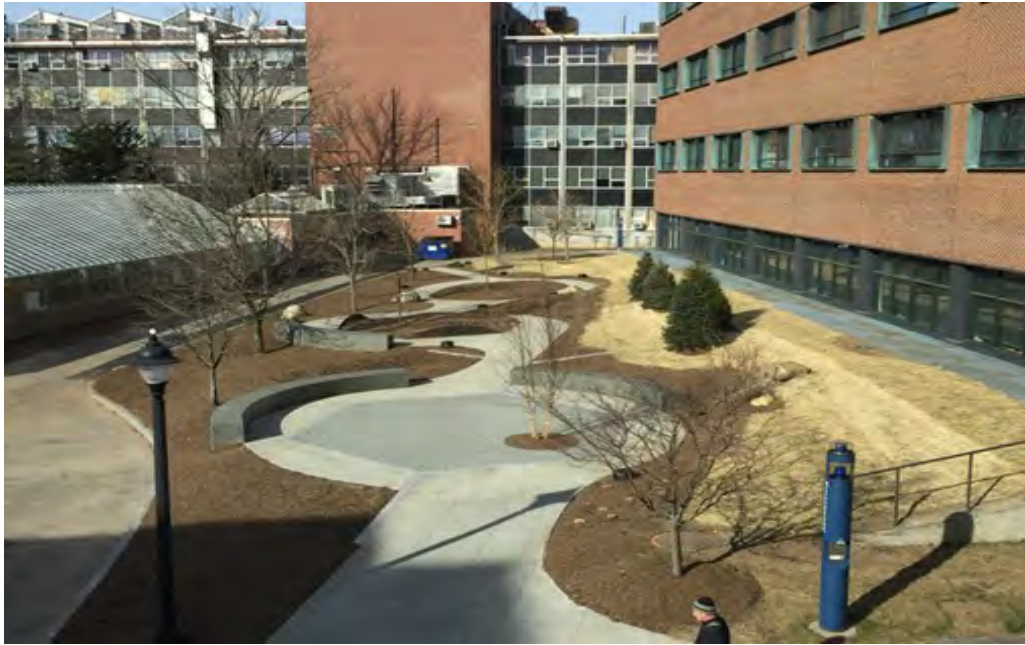
Medicinal Garden Substantially Complete
