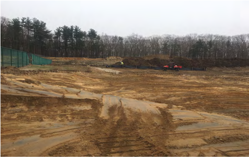
Installation of construction / Silt fencing
