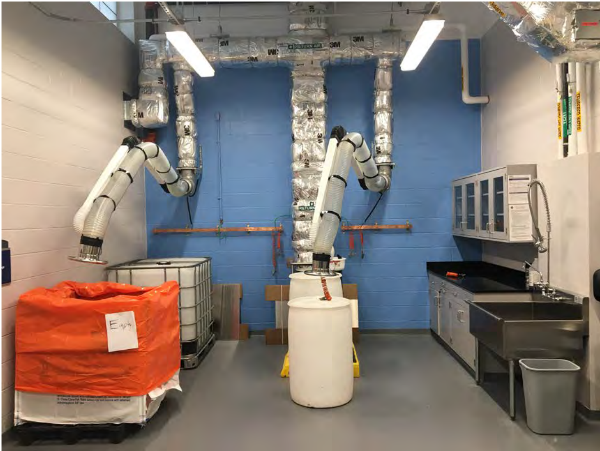
Chemical Processing Room
