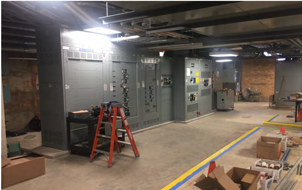
New switchgear in place
