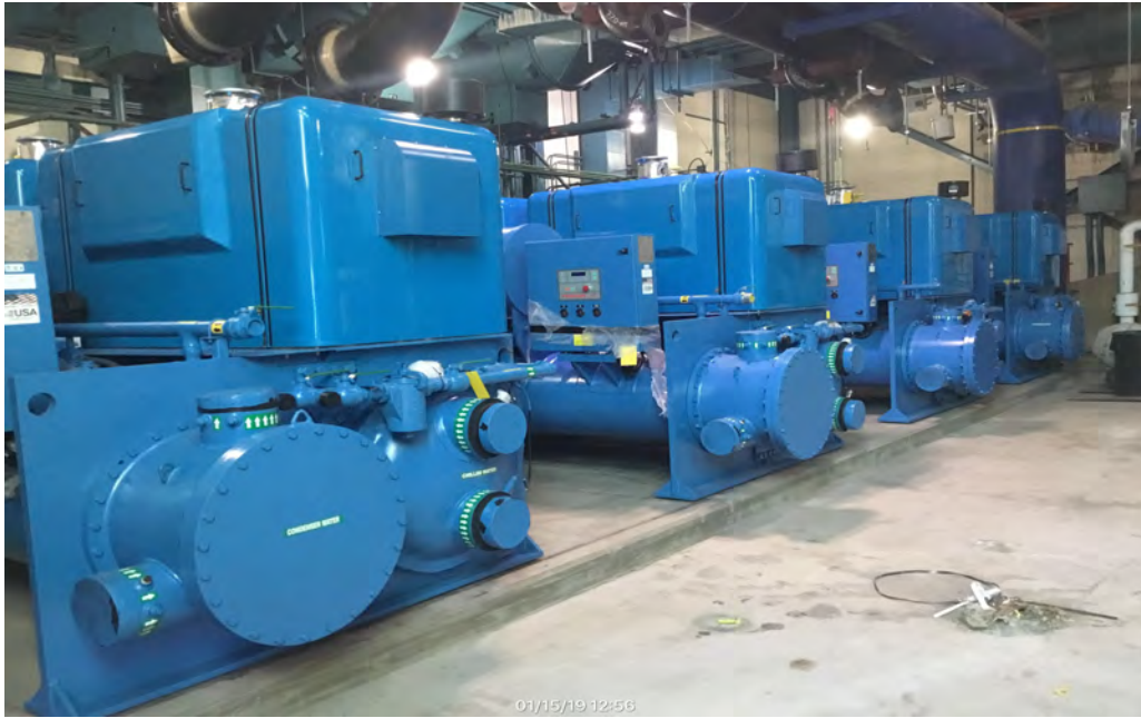
New Chillers Set in Place
