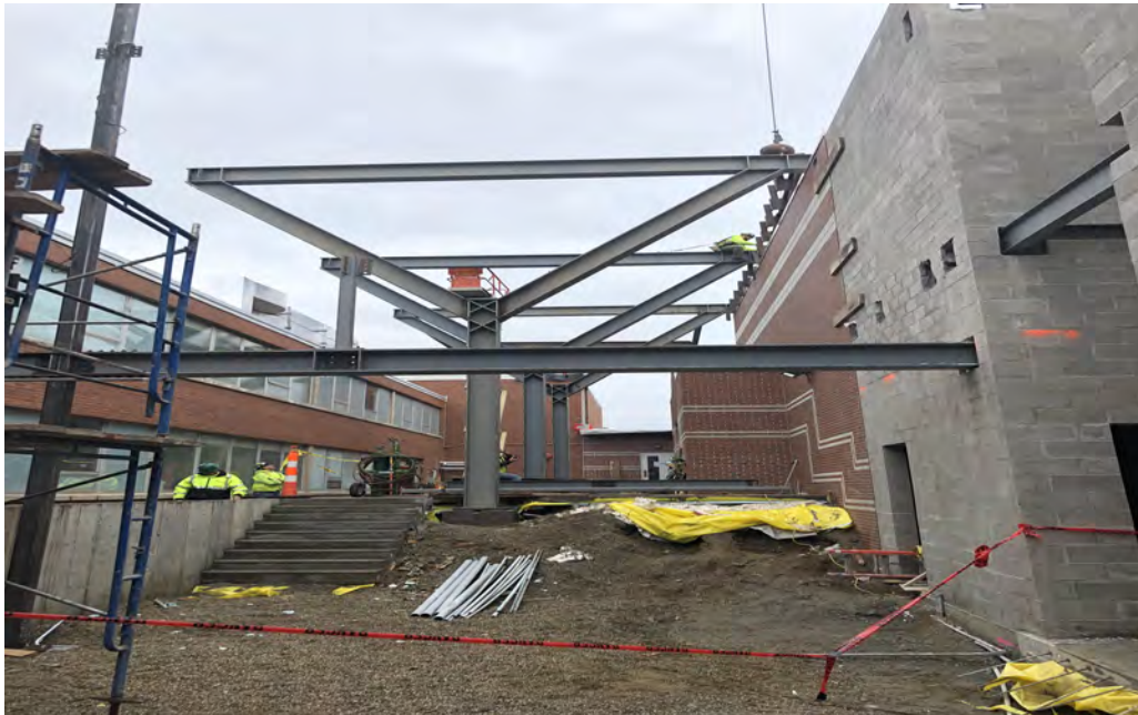
Fine Arts Production Facility - Courtyard Y-columns
