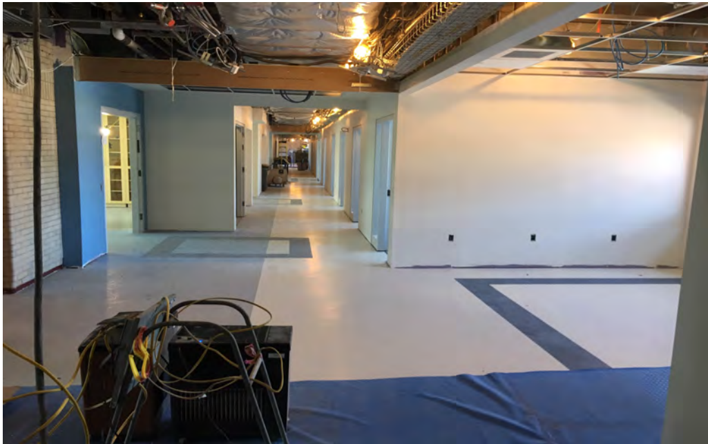
South tower 4th floor drywall and vinyl enhanced tile (VET).
