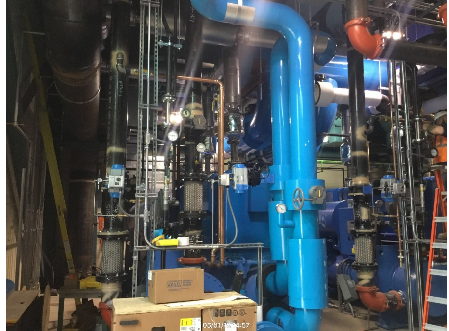
Chiller piped and connected to Chilled Water distribution system
