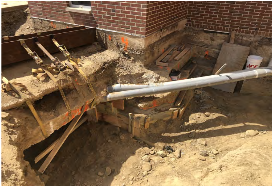
Underpinning Existing Nafe Katter Theater Foundation
