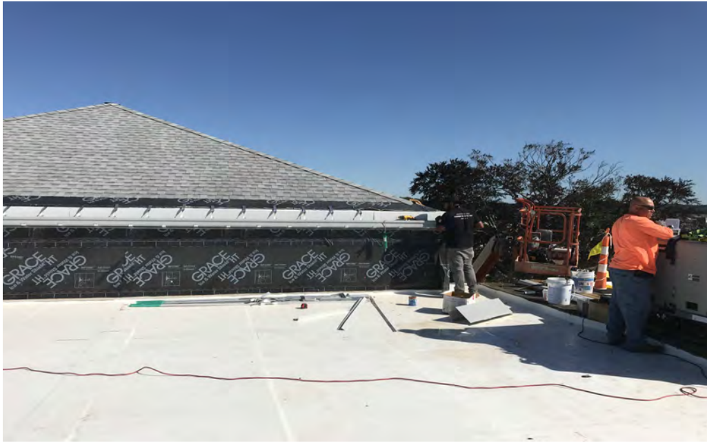
New PVC roof, asphalt shingle roof, and aluminum gutters
