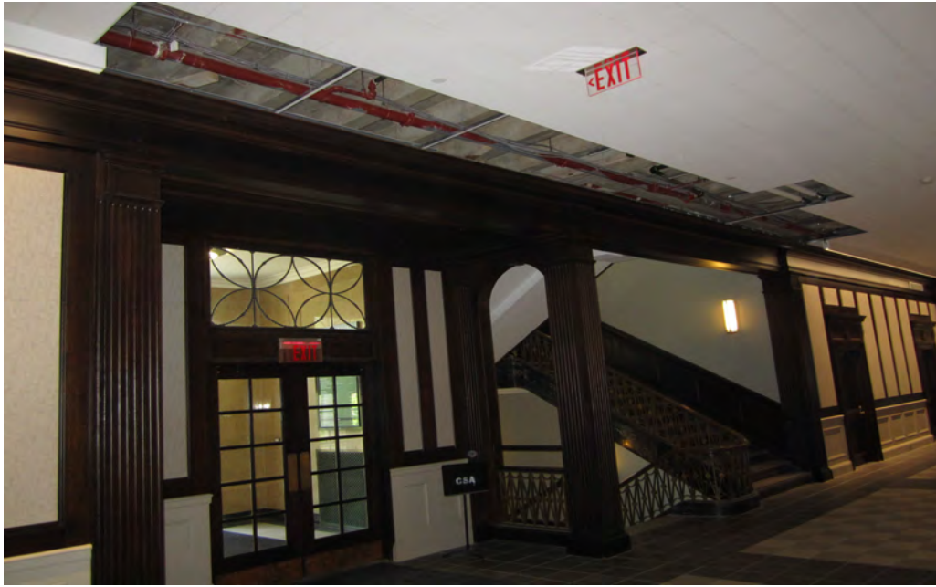
Installation of Smoke Curtain and Sprinklers
