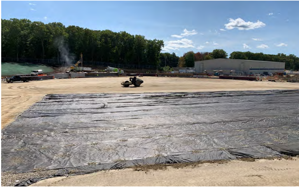
Baseball Underground Drainage System - Complete
