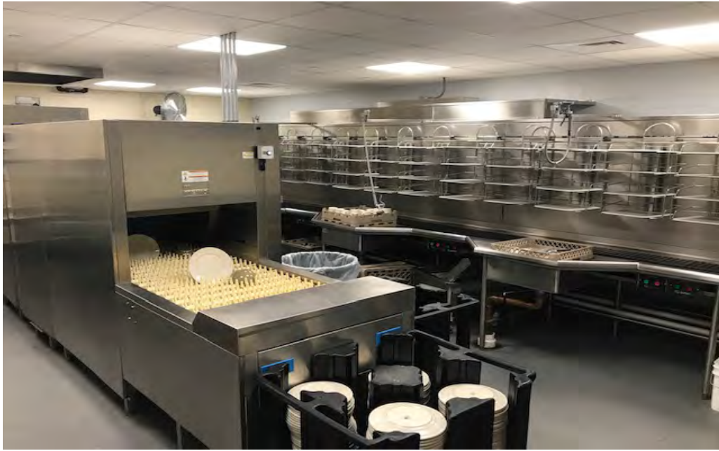
New Dish Washing Equipment and Accumulator
