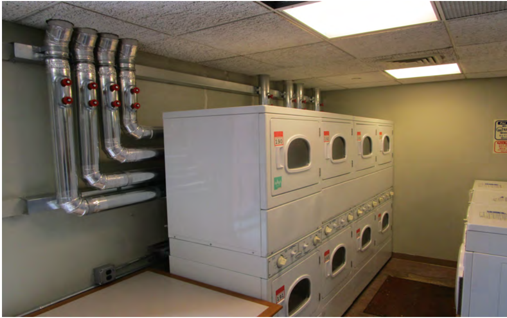
New Dryer Exhaust Venting
