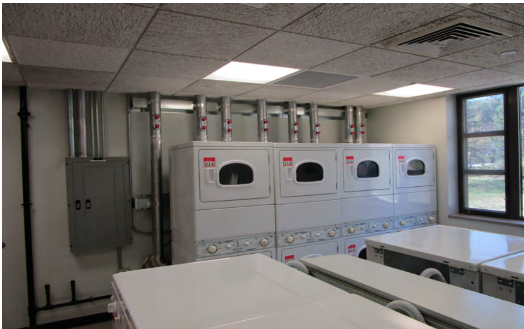
Upgraded Exhaust Clean-Outs
