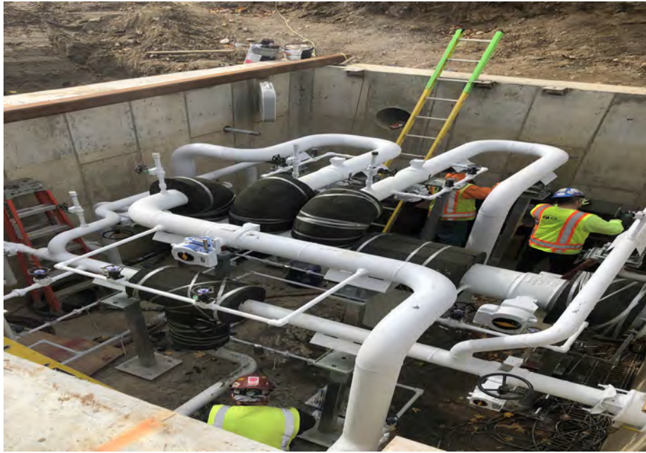
Vault F8 Steam pipe being insulated
