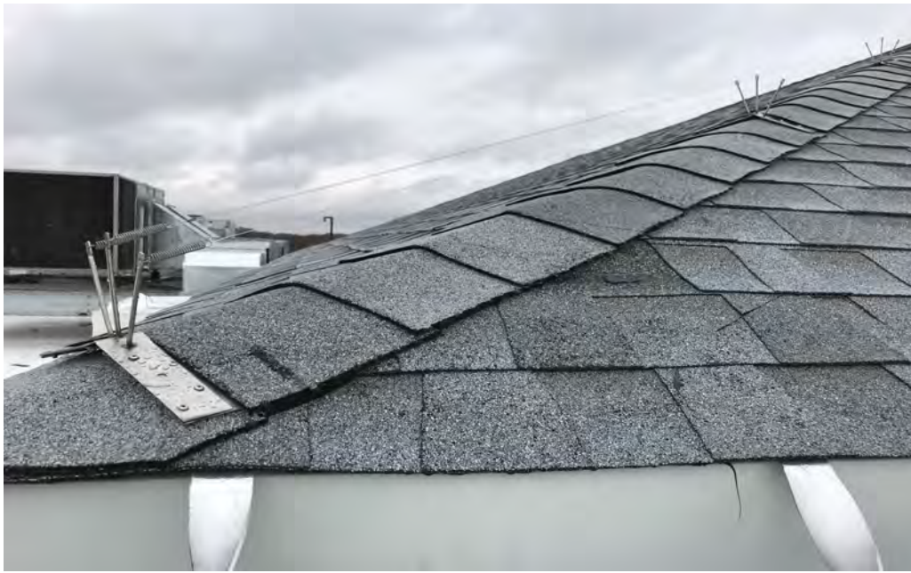
Asphalt shingle roof with wire bird deterrent system
