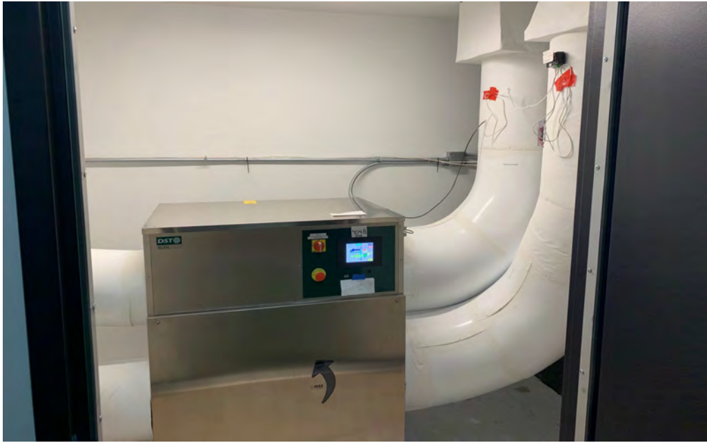
Desiccant Dehumidifier Unit (1 of 2 installed)
