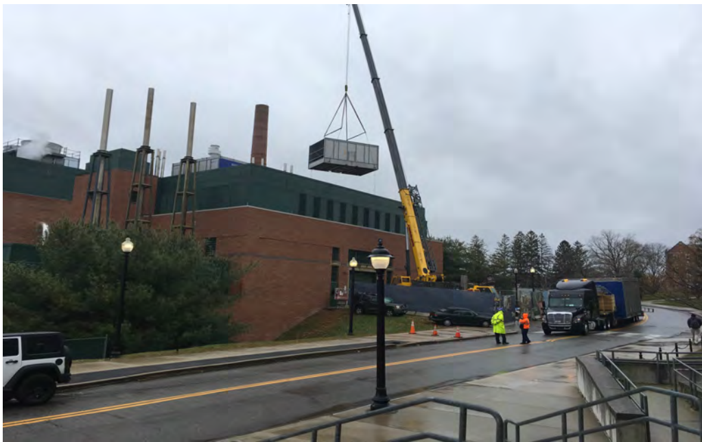
Cooling Tower Crane Lift to Roof of CUP
