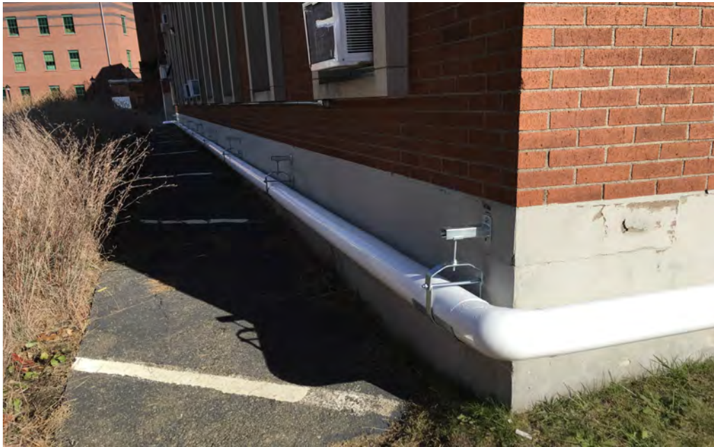
Temporary Steam Pipe to Infirmary
