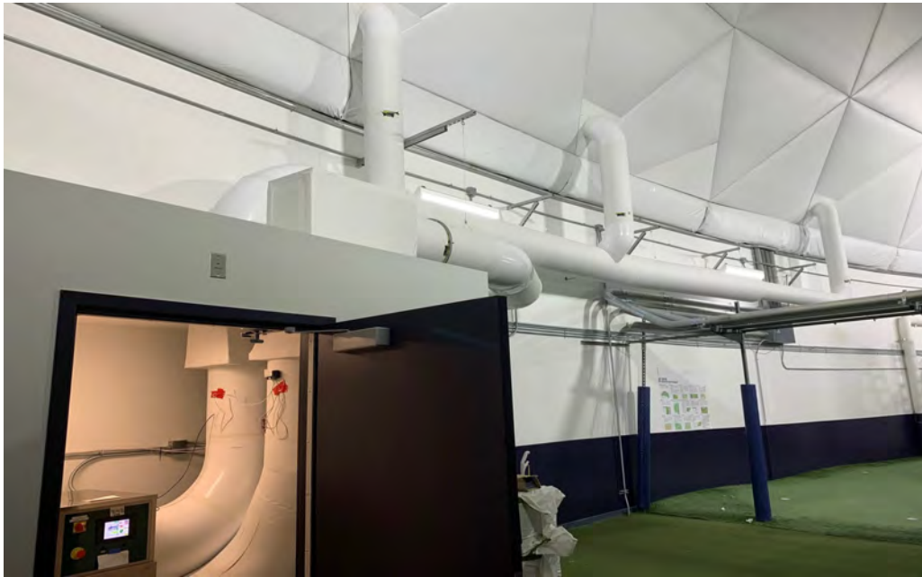
Desiccant Dehumidifier Units connected to ceiling panels
