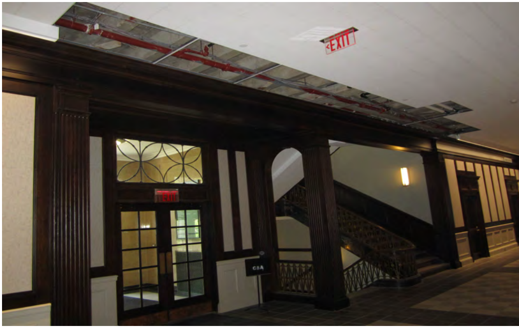
Installation of Smoke Partition and Sprinklers
