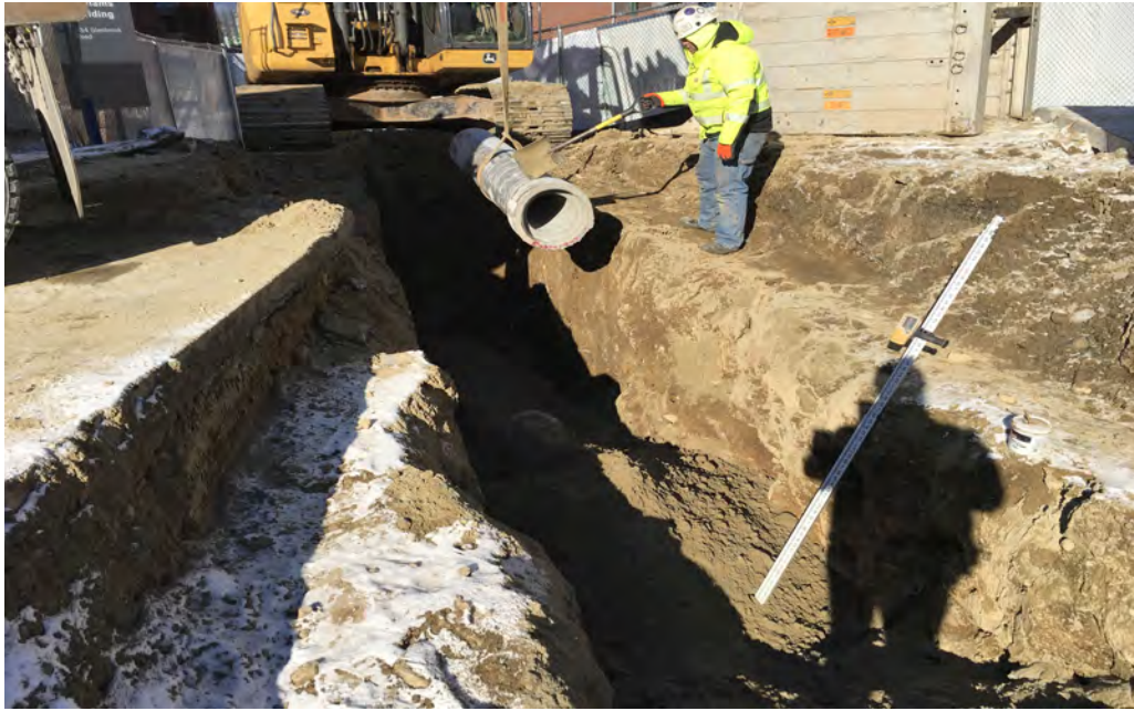
Tunnel Ventilation Pipe Being Installed
