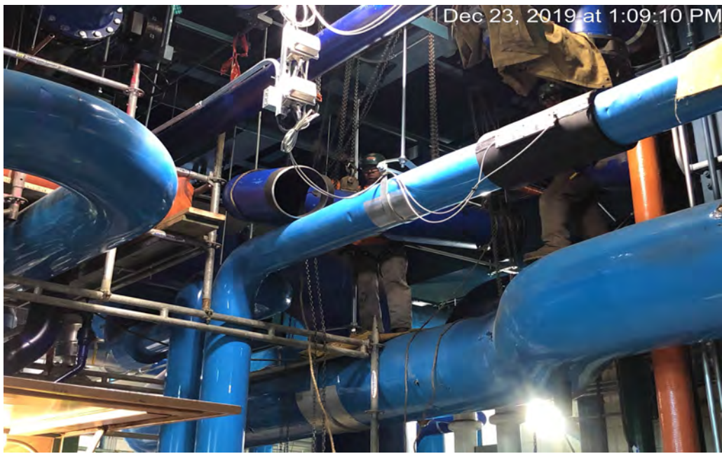
Cooling Tower Condenser Water Pipe Installation
