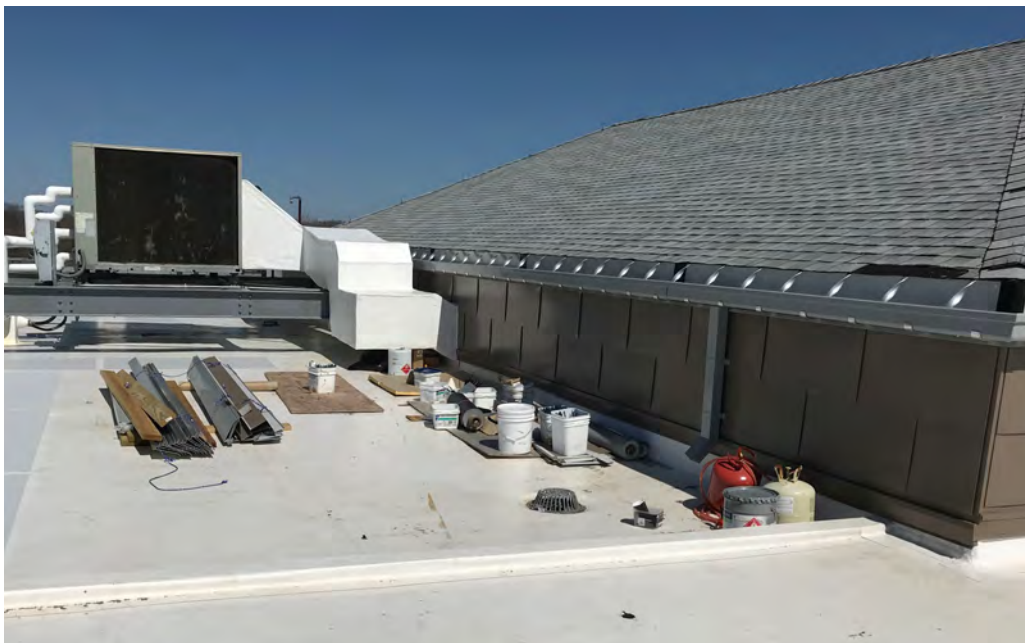
Metal wall cladding and duct insulation
