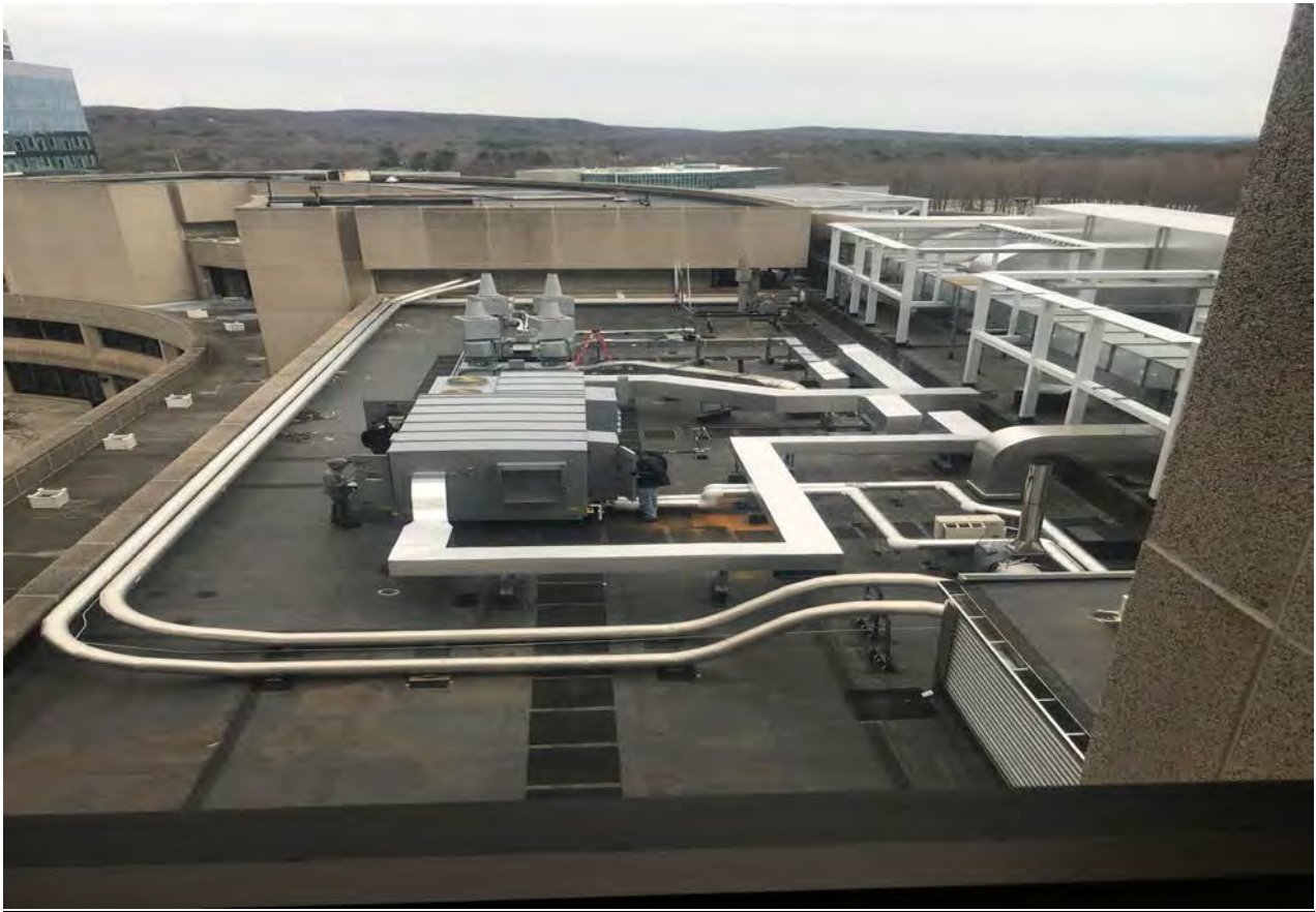
Inpatient Pharmacy New AHU and Exhausters
