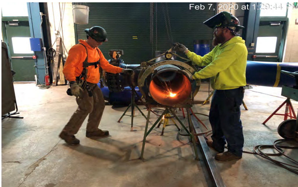
Cutting Condenser Water Pipe
