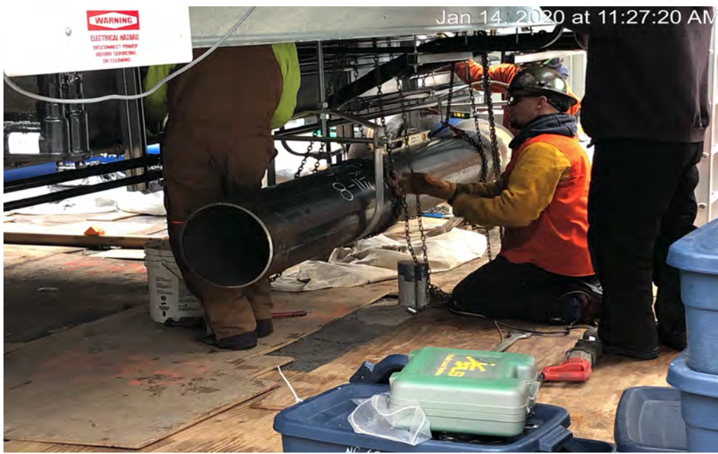
Condenser Water Pipe Installation Under Cooling Tower
