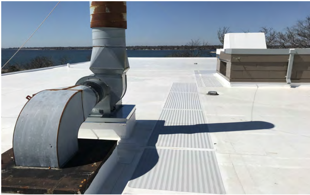
New roof, flashing, and walkpads
