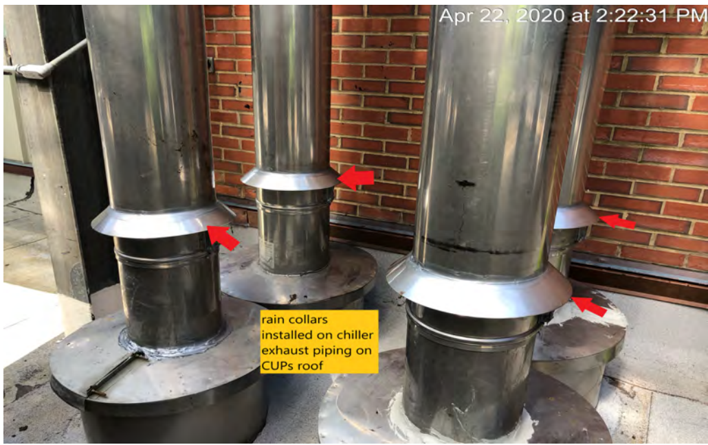
Chiller Exhaust Rain Collar Installation
