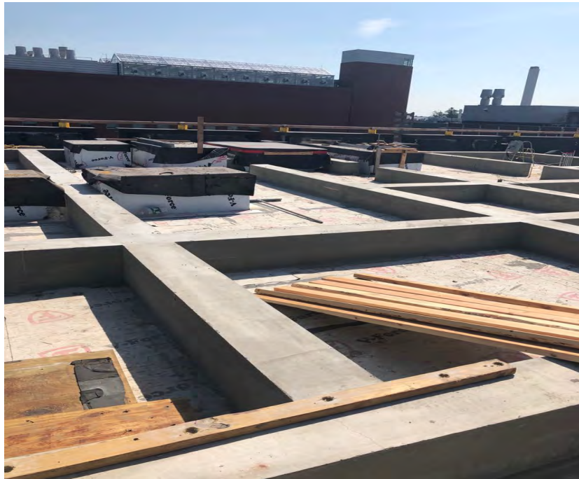
Gant West Roof - Concrete curbs for mechanical equipment
