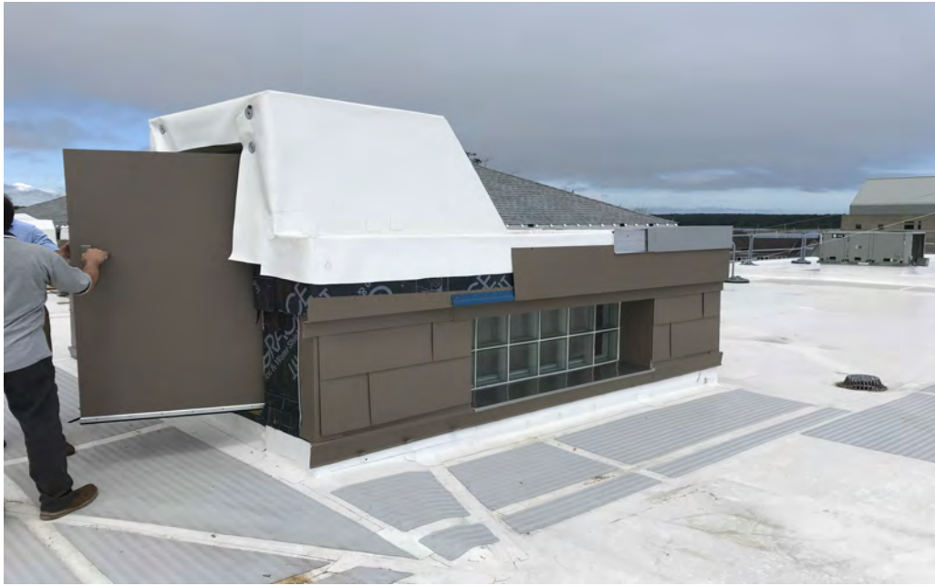
New door and flashing
