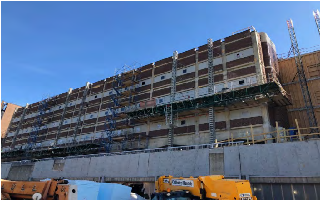
Gant West - Masons working on scaffold, repairing brick
