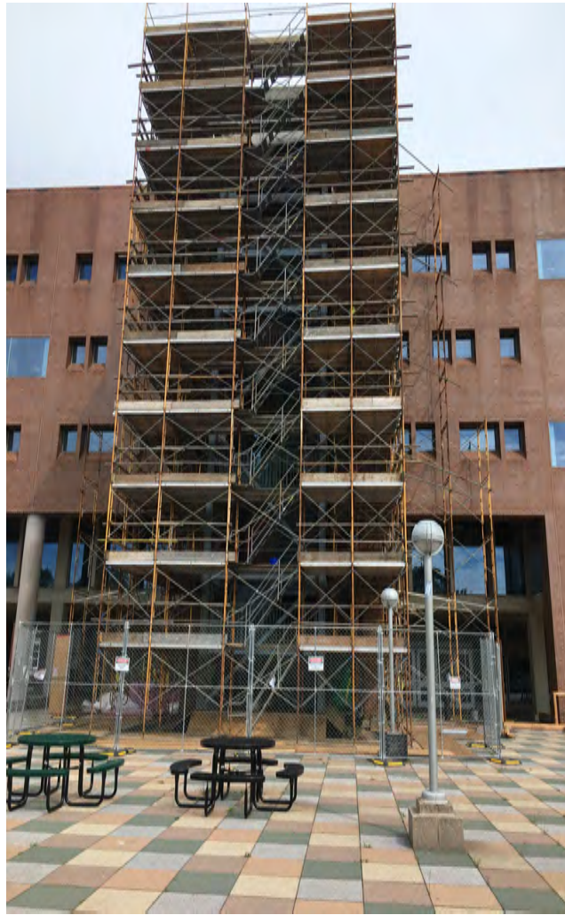
Stair tower installed (between scaffolding towers)
