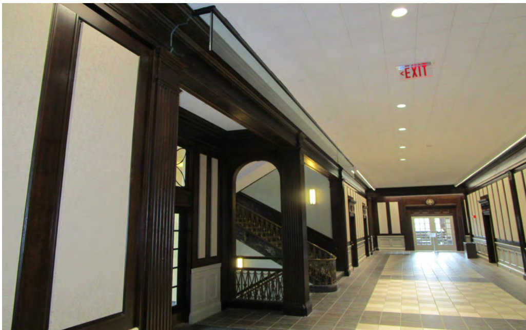
Completed Smoke Partition/Barrier
