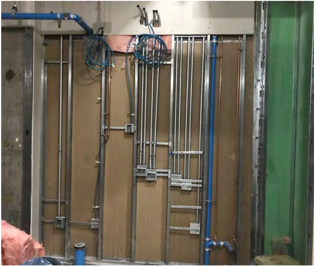
In-wall rough-in and drywall
