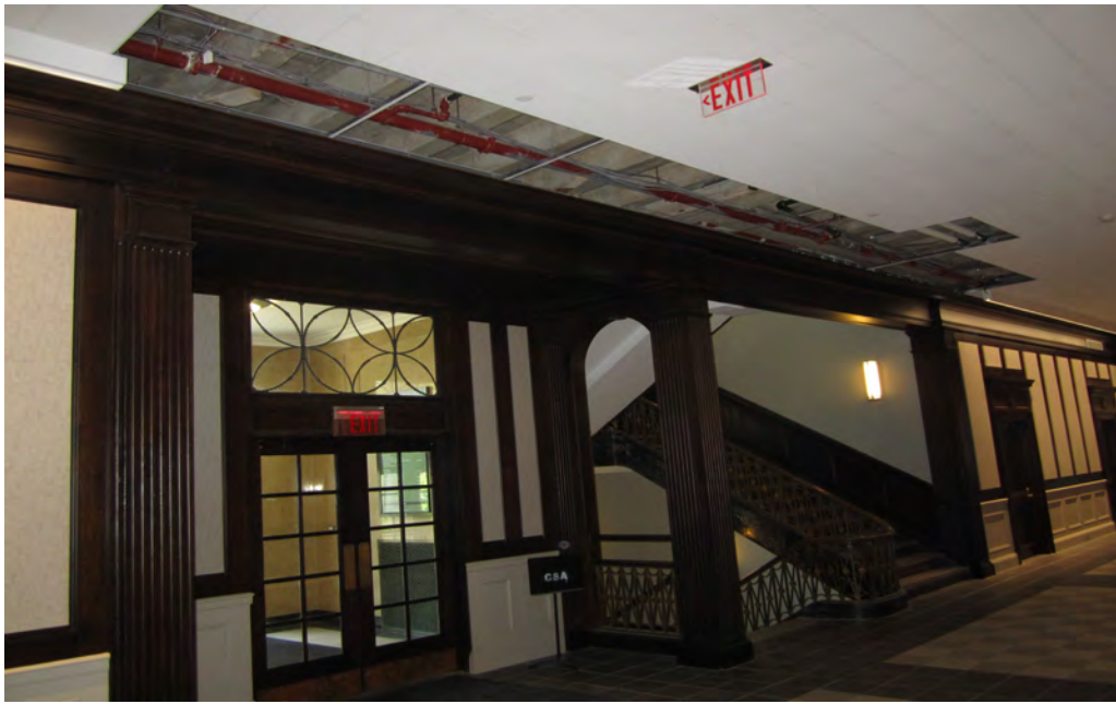
Installation of Smoke Partition and Sprinklers
