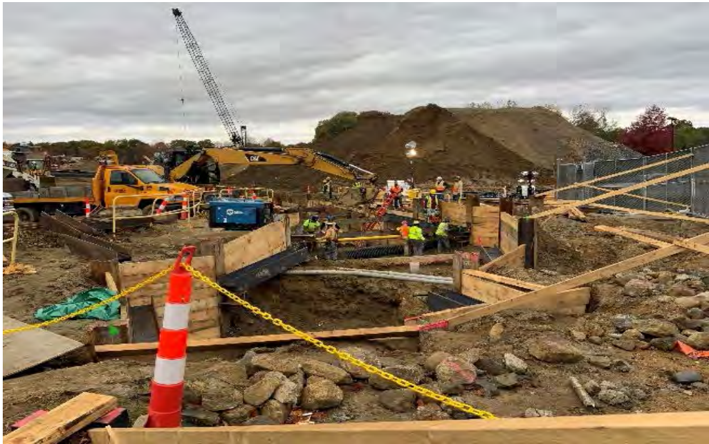
Tunnel Lagging Installation at the far East end of the site
