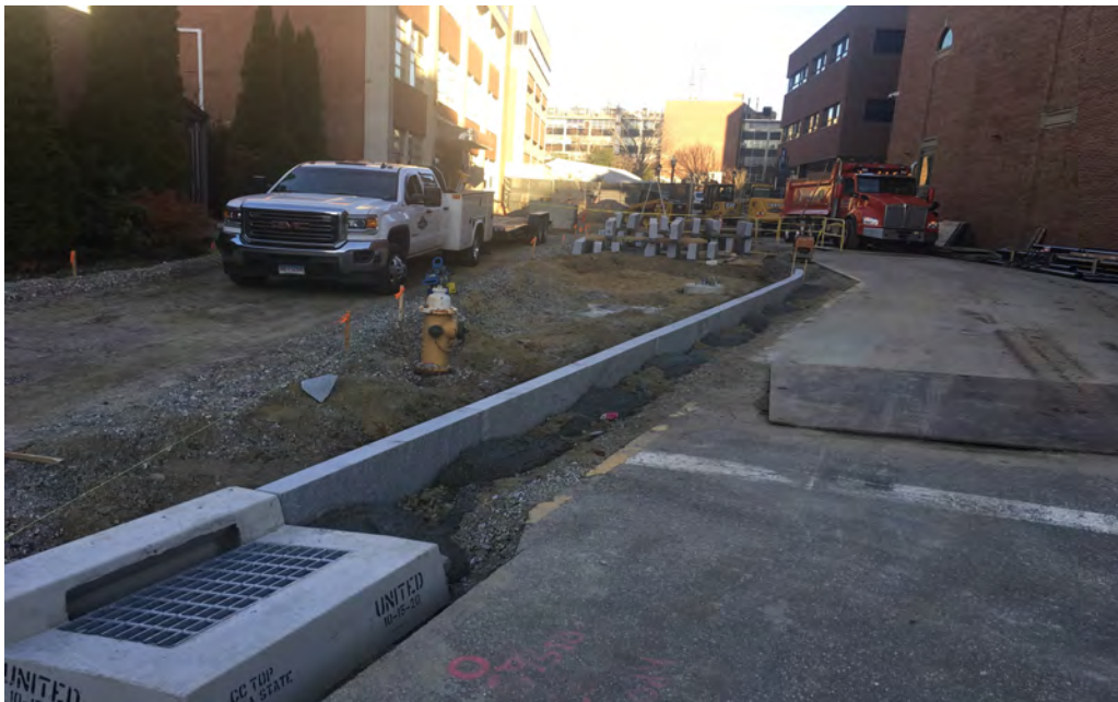
Granite curb installation west of Cogen looking North
