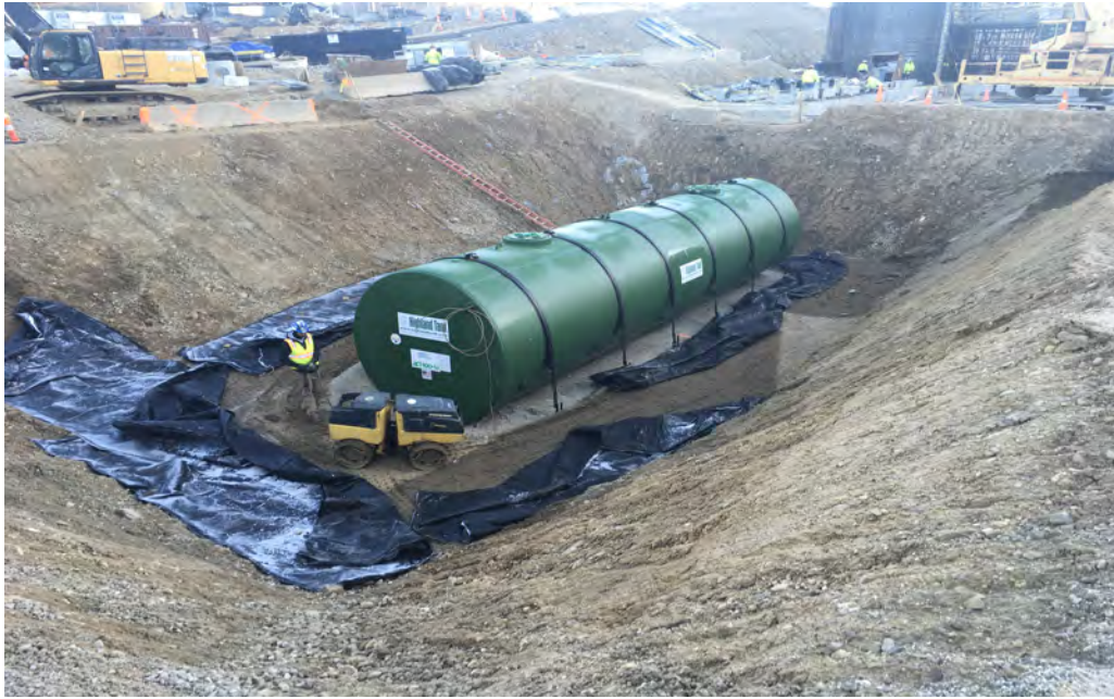
Oil tank installation looking northeast
