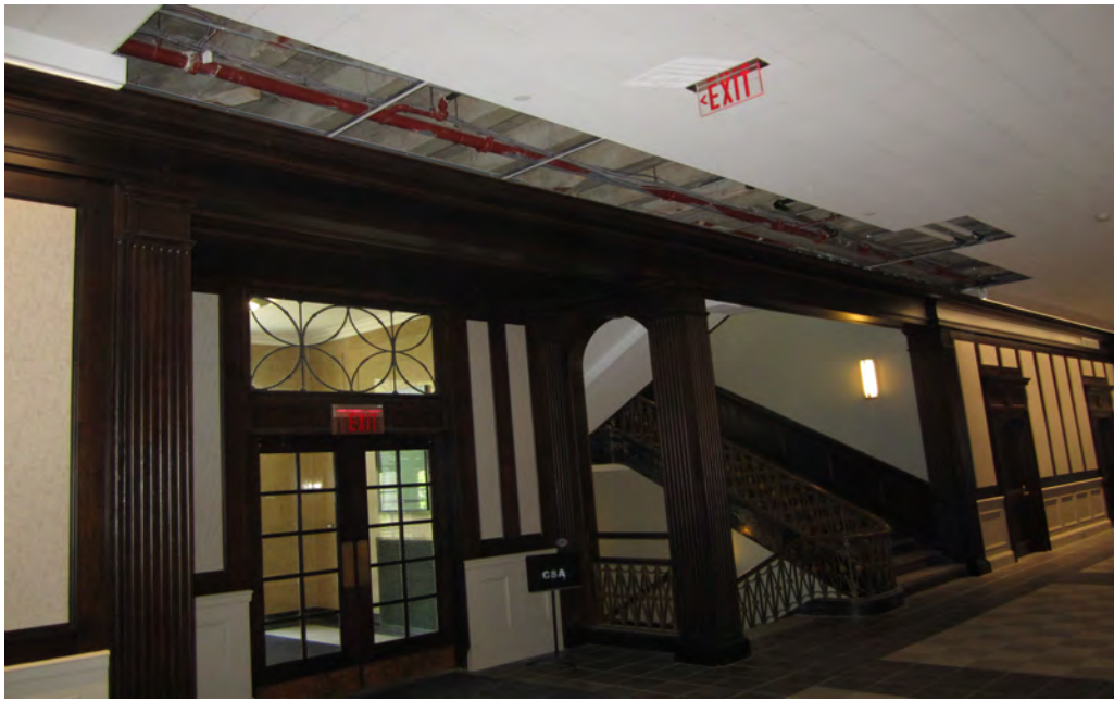
Installation of Smoke Partition and Sprinklers
