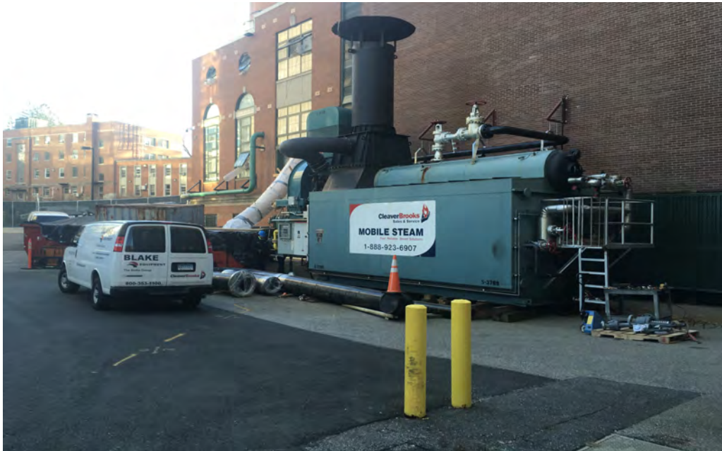
Temporary boiler in place North of boiler plant
