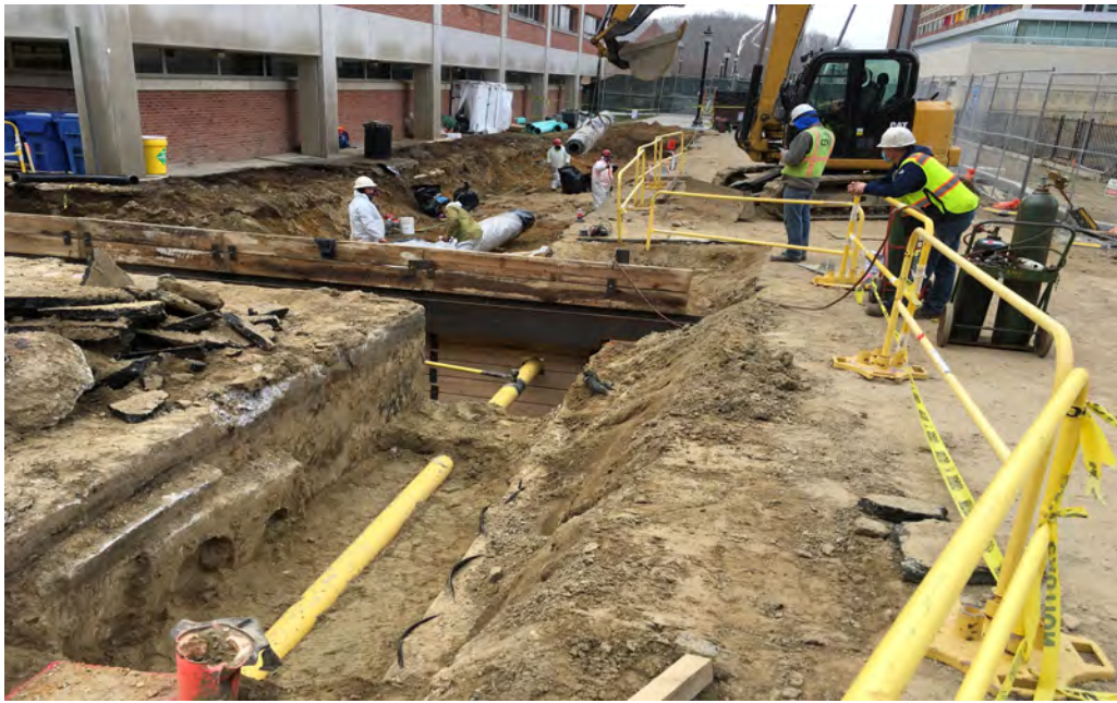
Existing steam pipe removal north of UTEB, looking west
