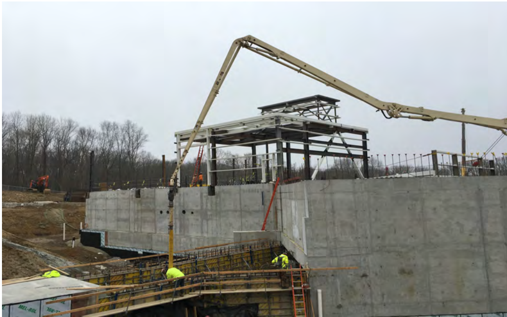
Concrete pumping west end of tunnel walls looking southwest
