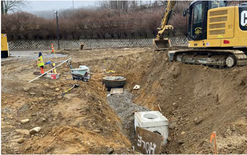
Storm Water Drain Installation
