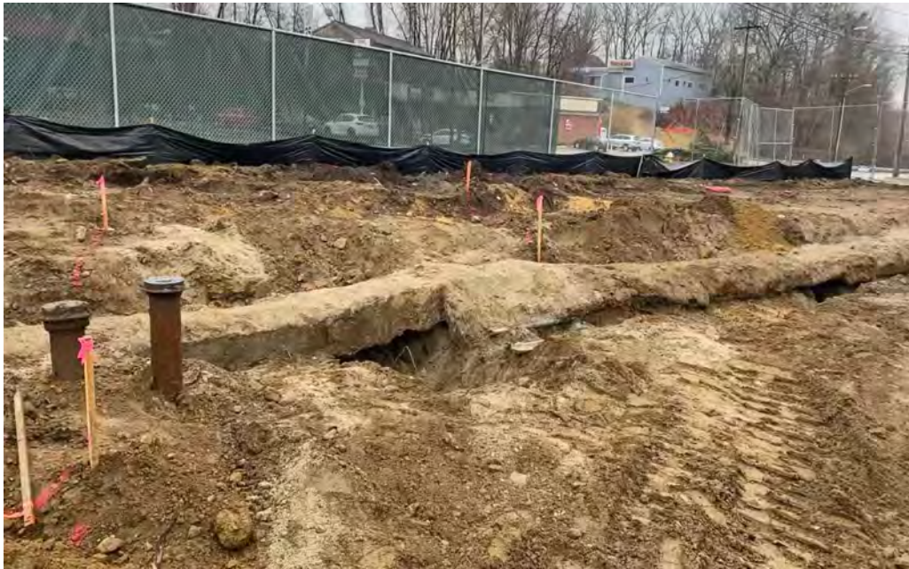
Uncovered Duct Bank and Gate Valve
