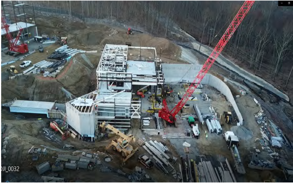
Boiler hall steel erection looking south
