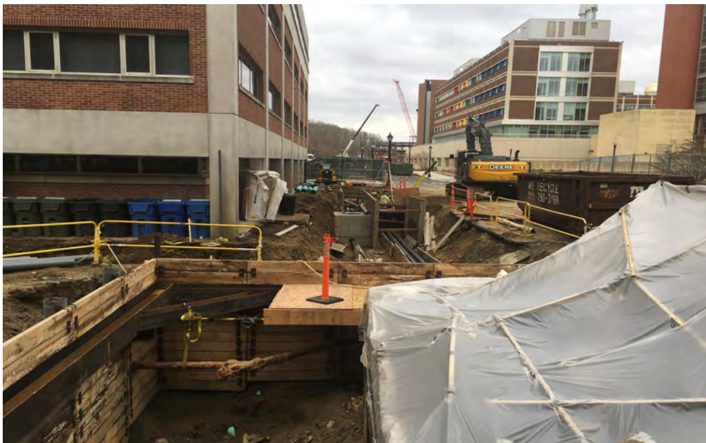
Electrical conduits in duct bank north of UTEB, looking west
