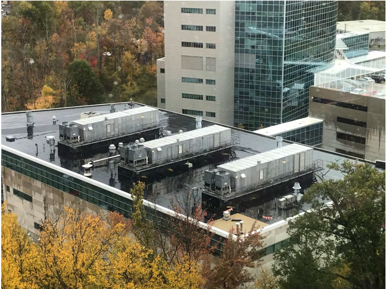
View of existing MSI Roof Top units #1, #2 & #3
