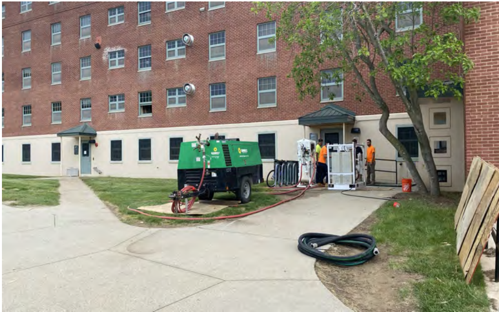
Equipment Used to Remove Asbestos Containing Skim Coat
