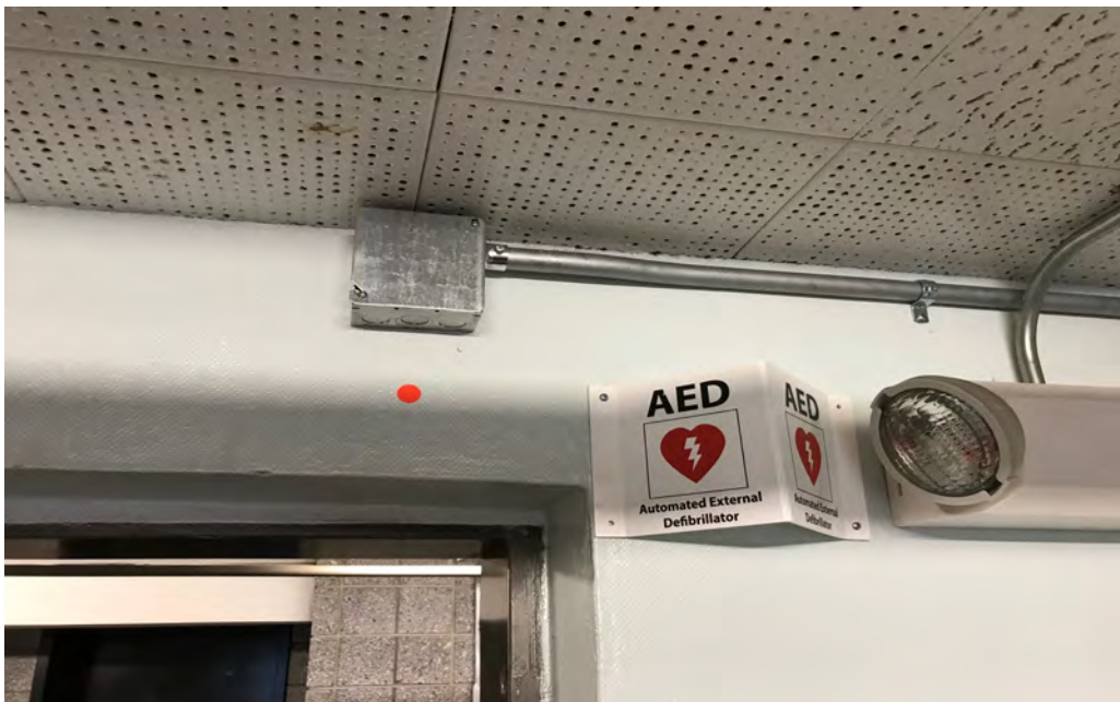
New conduit at North Campus
