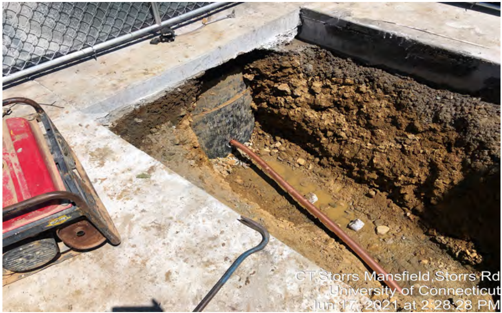
Force Main Installation into Sanitary Manhole
