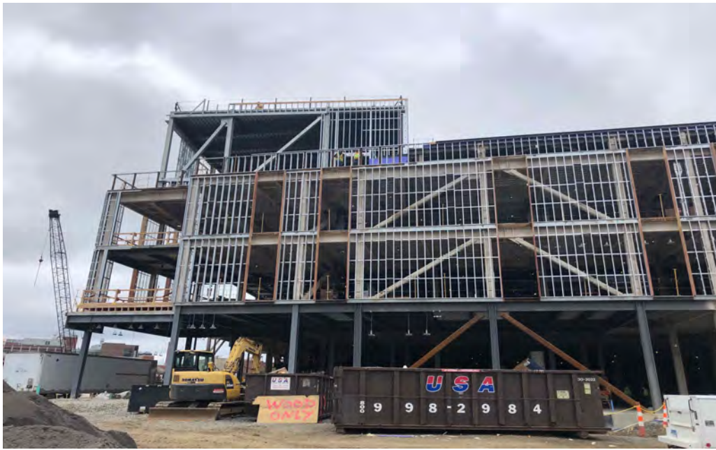
West Elevation Framing
