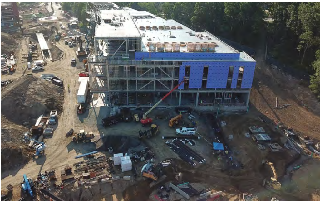
Utility work along West side of Science 1
