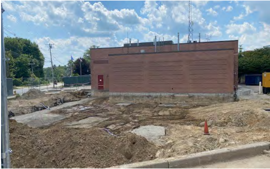
Site Ready for Footings
