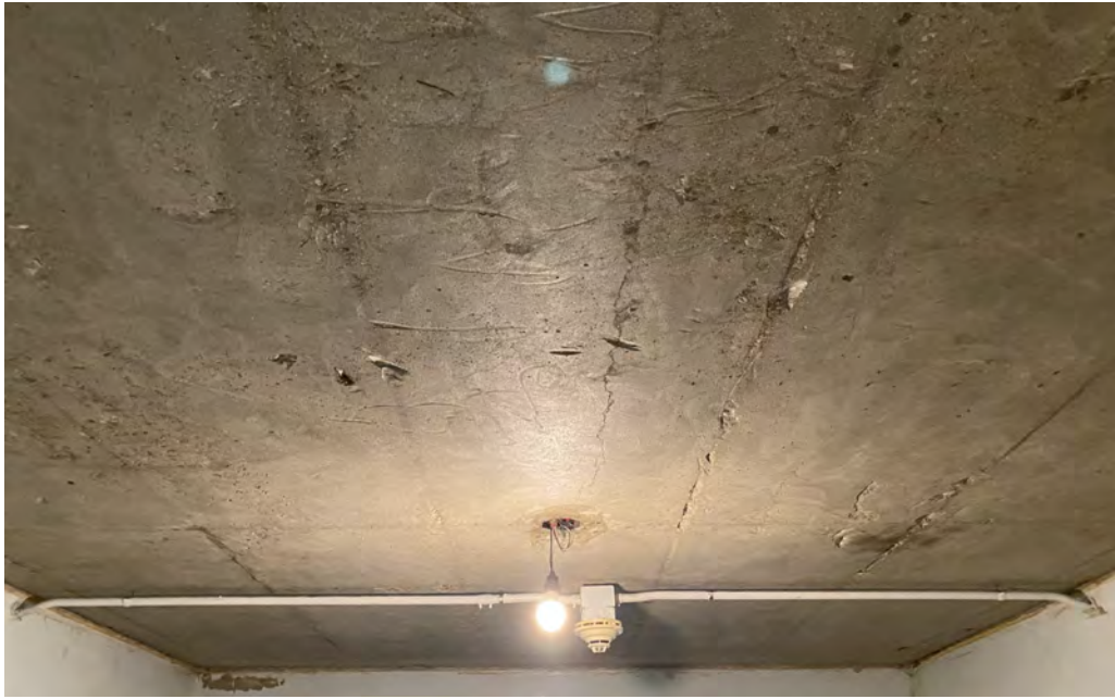
Student Room Ceiling with Asbestos Removed
