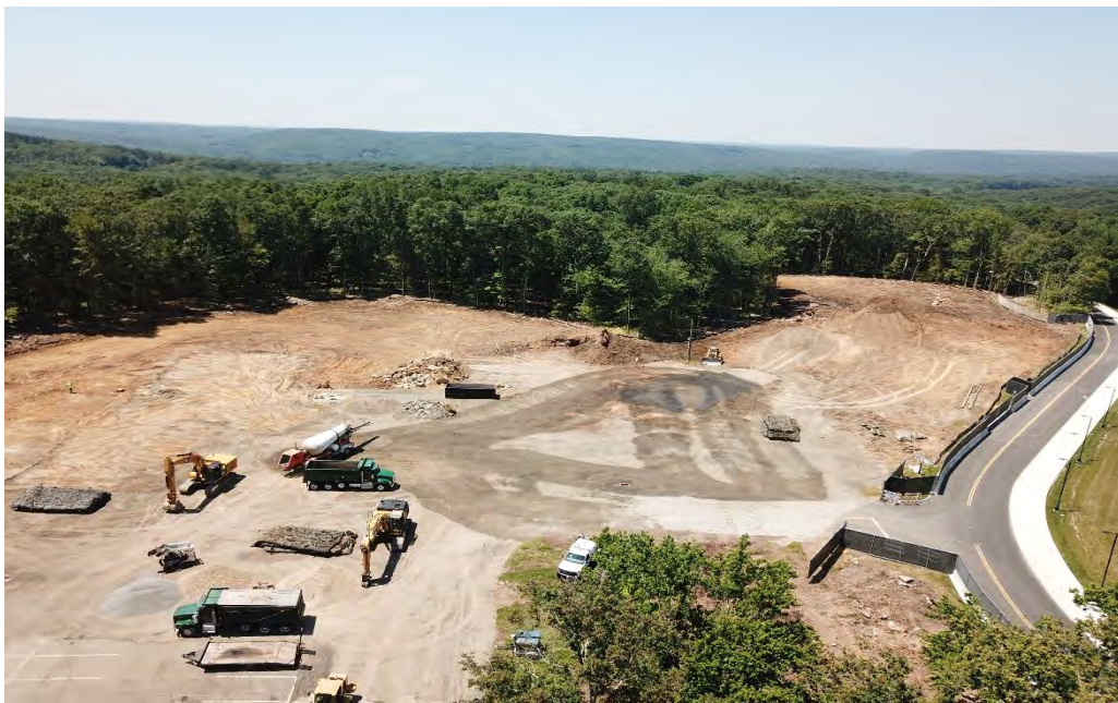
Trees cleared, top soil removed, blasting ledge started
