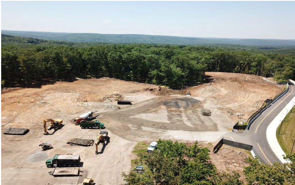
Trees cleared and topsoil stripped
