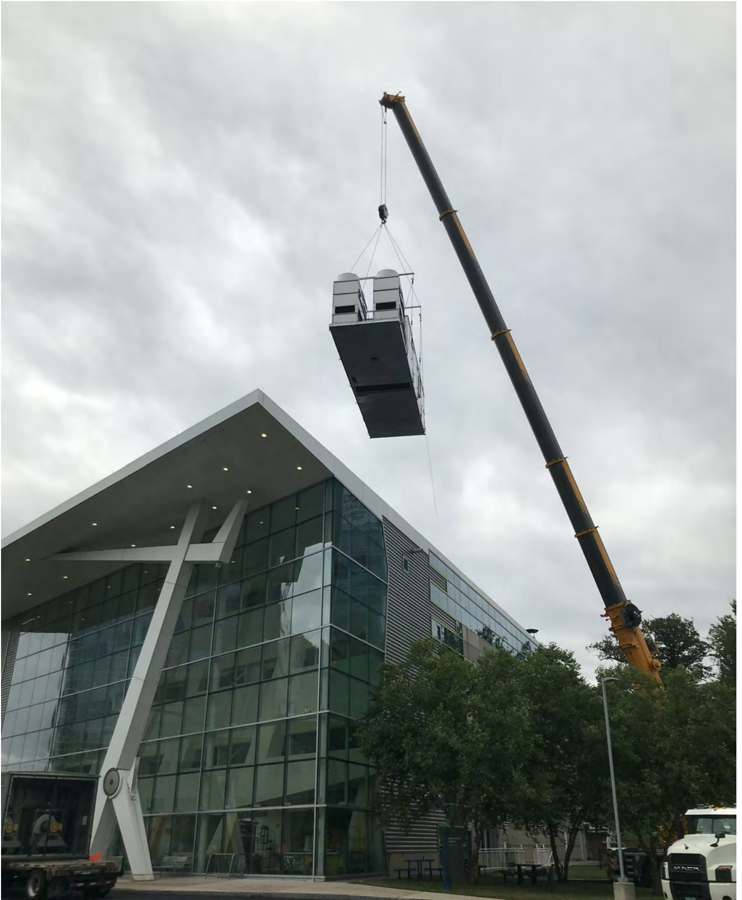
Rigging of the Roof Top Unit RTU-2
