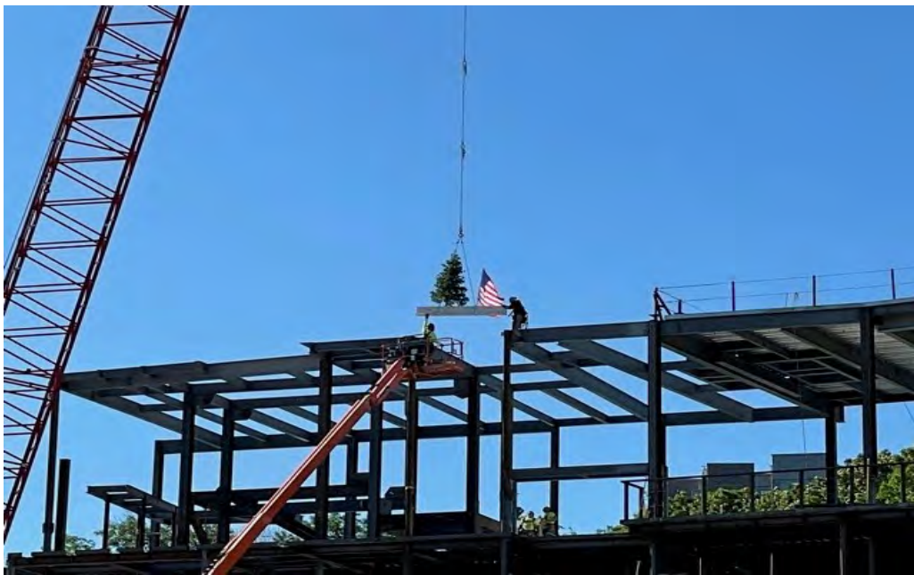
Structural Steel Topping Off
