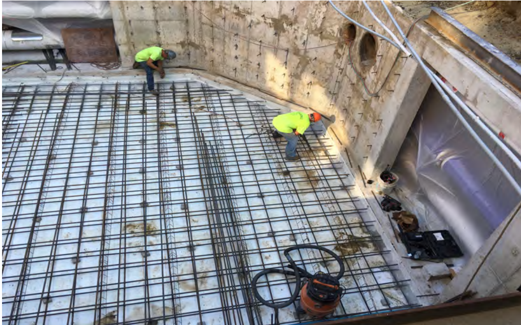
Tunnel bump out slab rebar installation west of Pharmacy
