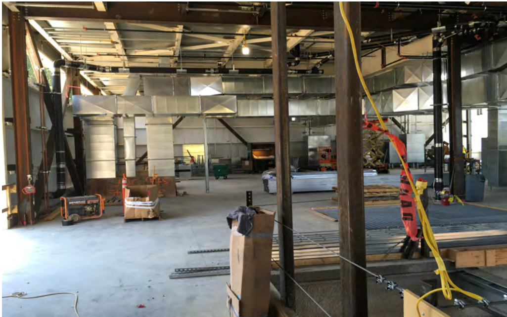
Ductwork installation 2nd floor looking south
