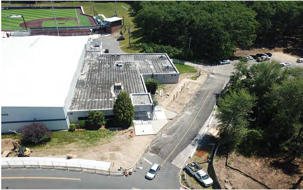
Sidewalks, parking & two-way traffic lanes established.
