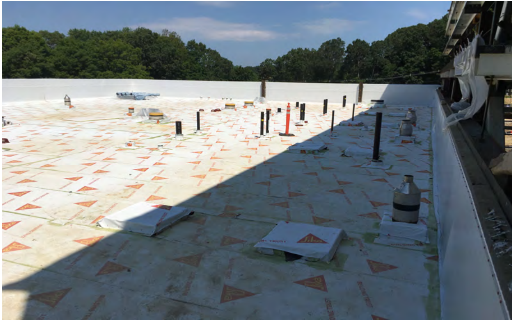
Cooling tower roof awaiting support steel looking north
