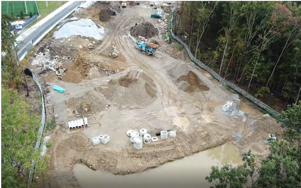
West Lot - Unsuitable soils to be removed to progress work
