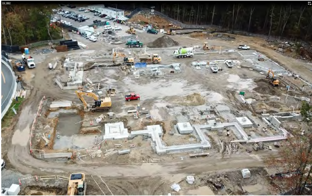
Installation of footings and foundations
