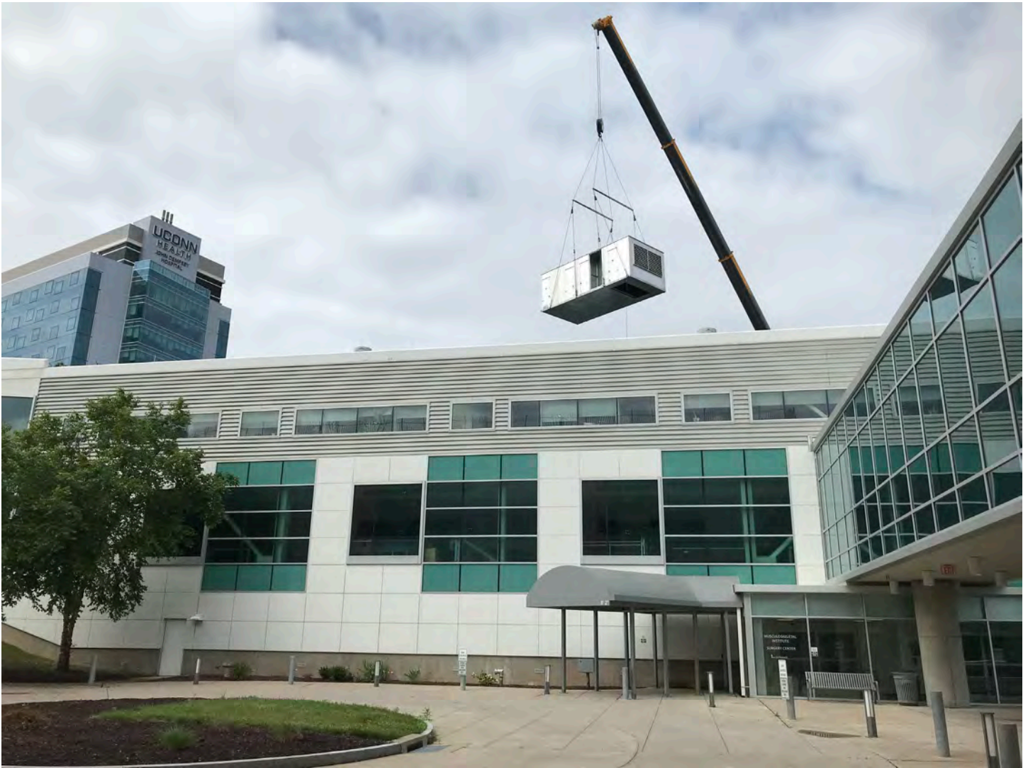
Rigging the Final Roof Top Unit RTU-3
