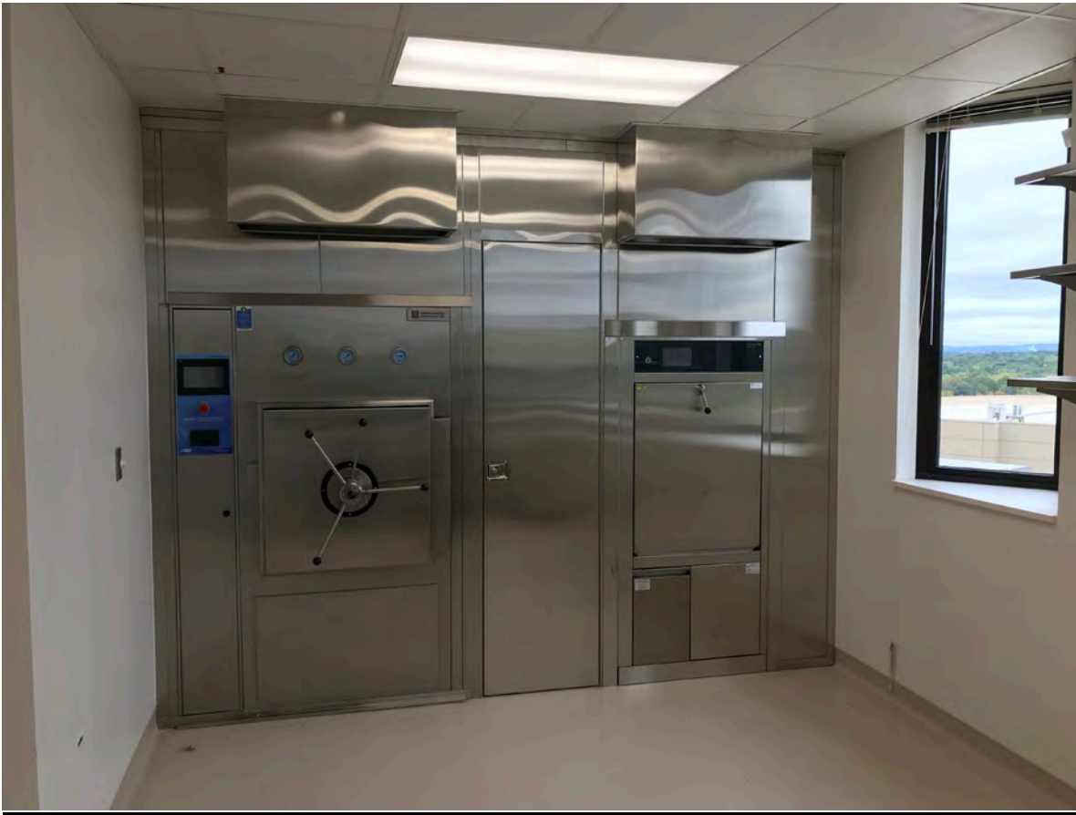
Autoclave & Glass washer
