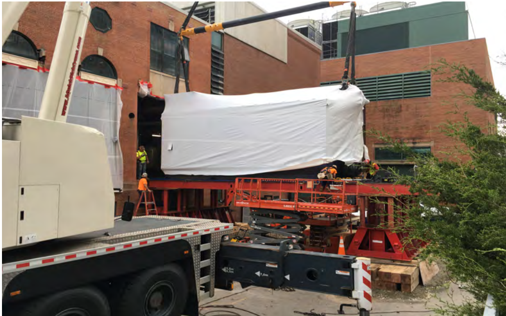
Boiler #2 being rigged into boiler plant
