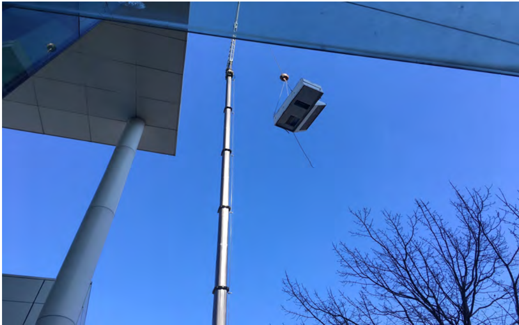
Placement of Roof Top Unit
