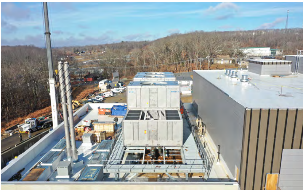
Chiller hall roof, cooling tower and generator stacks
