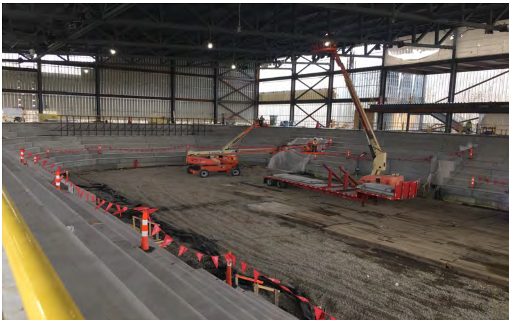
Stadia precast is near completion
