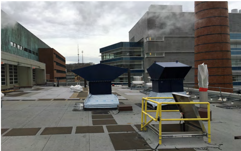
Boiler air intakes at roof
