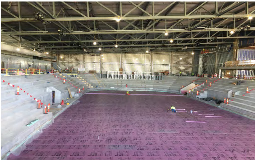
Pre-cast seating is complete and rink is ready to be poured
