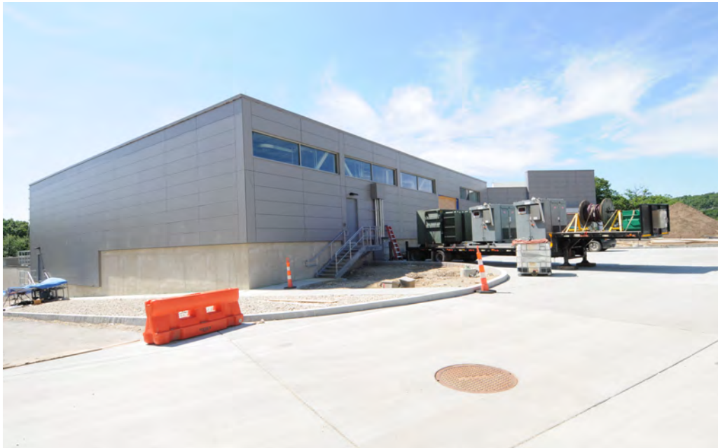
Load bank trailer for emergency generator test looking northwest
