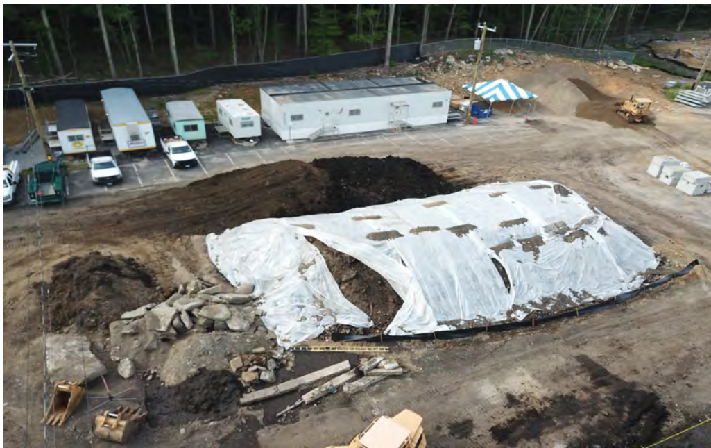
East Lot - Retaining Wall excavation - Unsuitable soils
