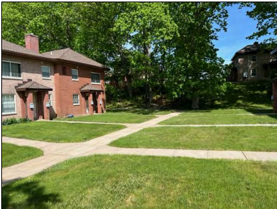
Photo 4. Overview photo from west-central portion of the project area facing southeast with Building 4 in view.
