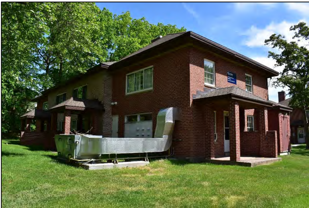
Photo 13. Building 13 rear elevation, facing north.
