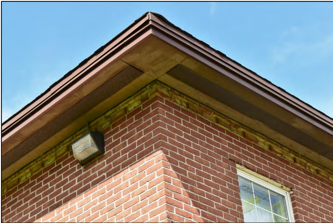
Photo 17. Detail of cornice on Building 3, facing west.
