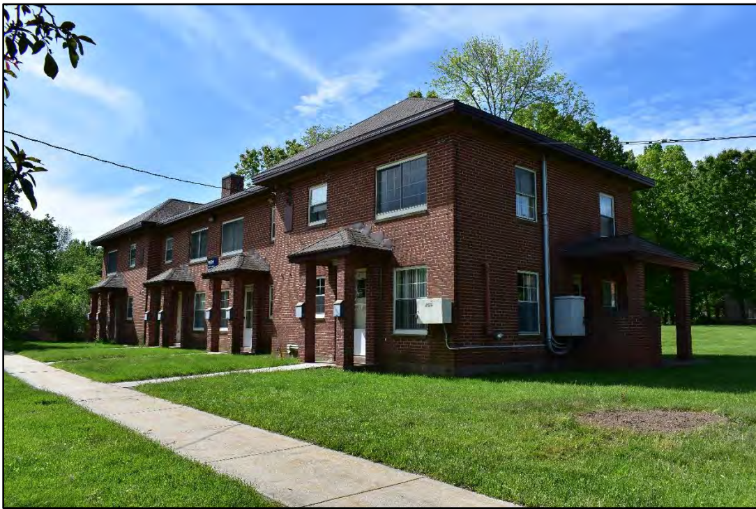
Photo 8. Building 2 façade, facing south.
