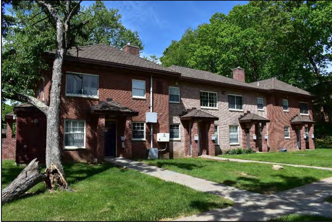
Photo 12. Building 13 façade, facing west.
