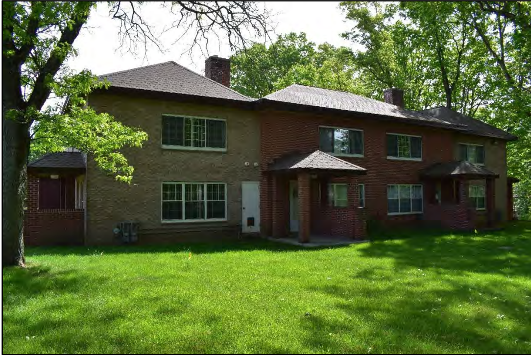
Photo 11. Building 5 rear elevation, facing northeast.
