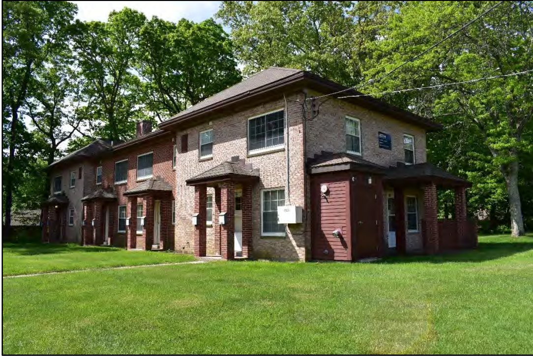
Photo 10. Building 5 façade, facing south.
