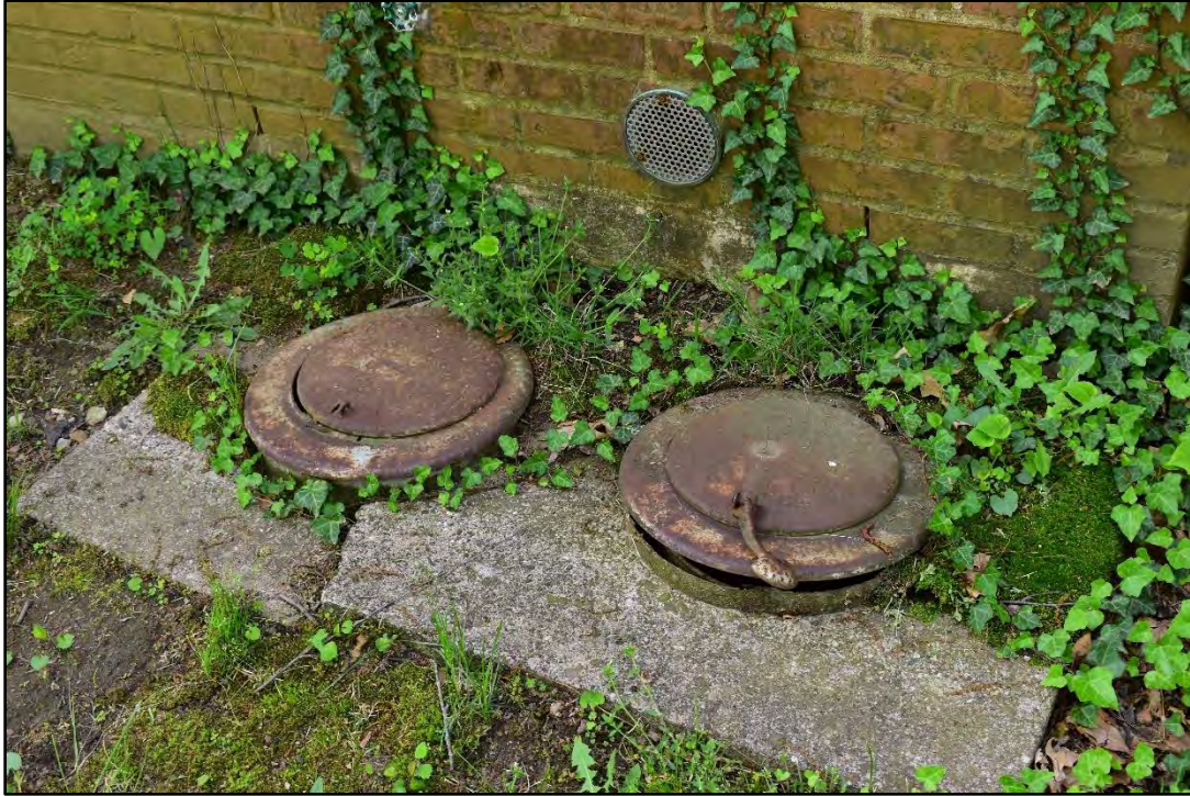
Photo 18. Detail of coal holes outside Building 7, facing south.
