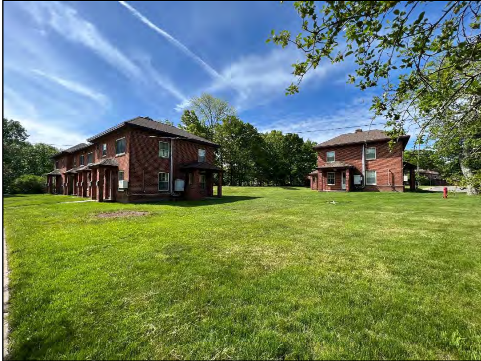
Photo 1. Overview photo from northern corner of project area facing south with Buildings 2 and 3 in view.
