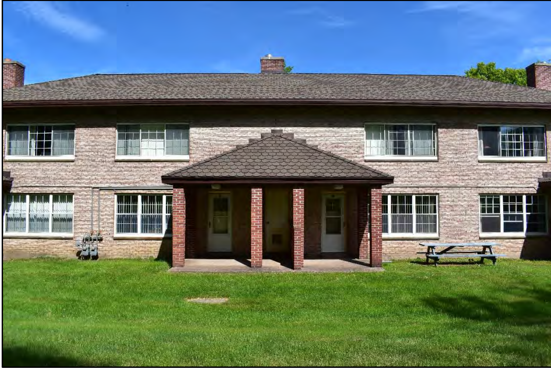
Photo 16. Detail of double portico on Building 3 rear elevation, facing west.
