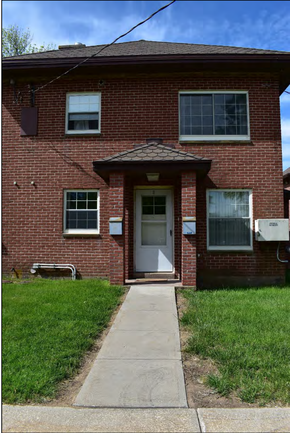
Photo 9. Detail of a single unit of Building 2, facing south.
