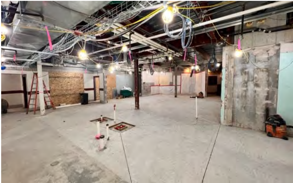
Men's Locker Room After Under Slab Plumbing Completed
