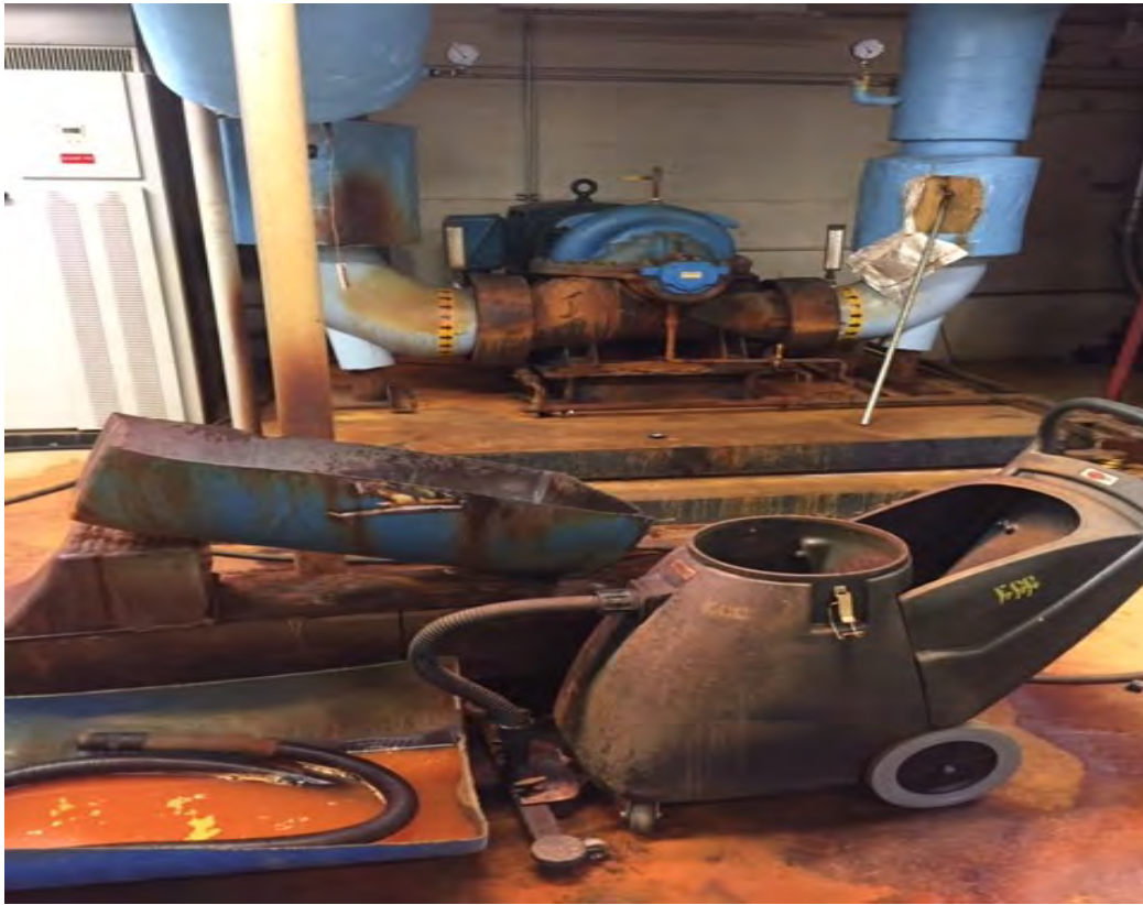
Mechanical Room with existing Chilled Water Pump #4
