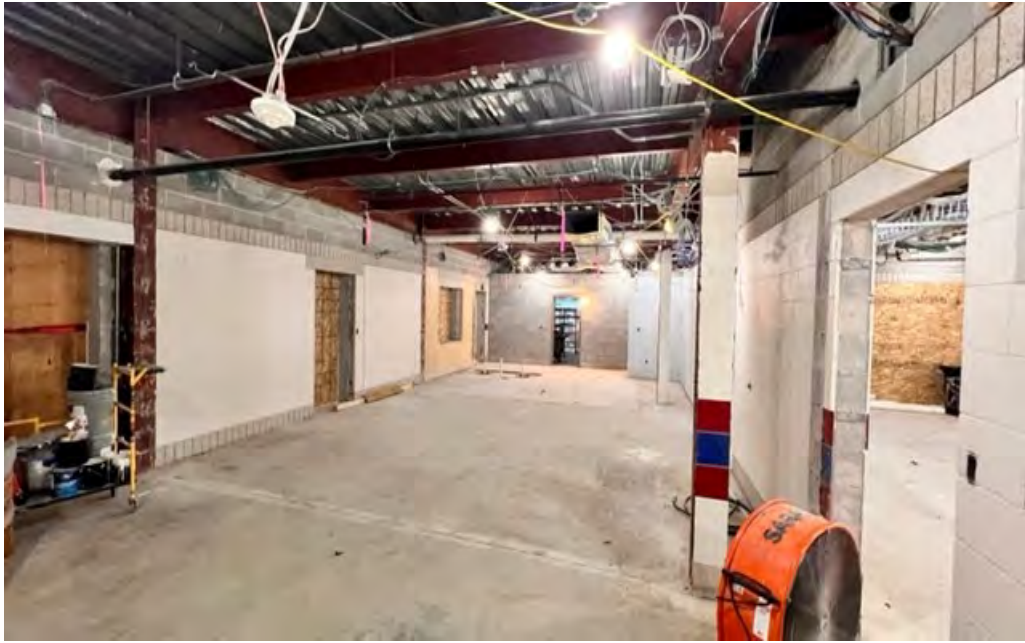
Women's Locker Room After Under Slab Plumbing Completed
