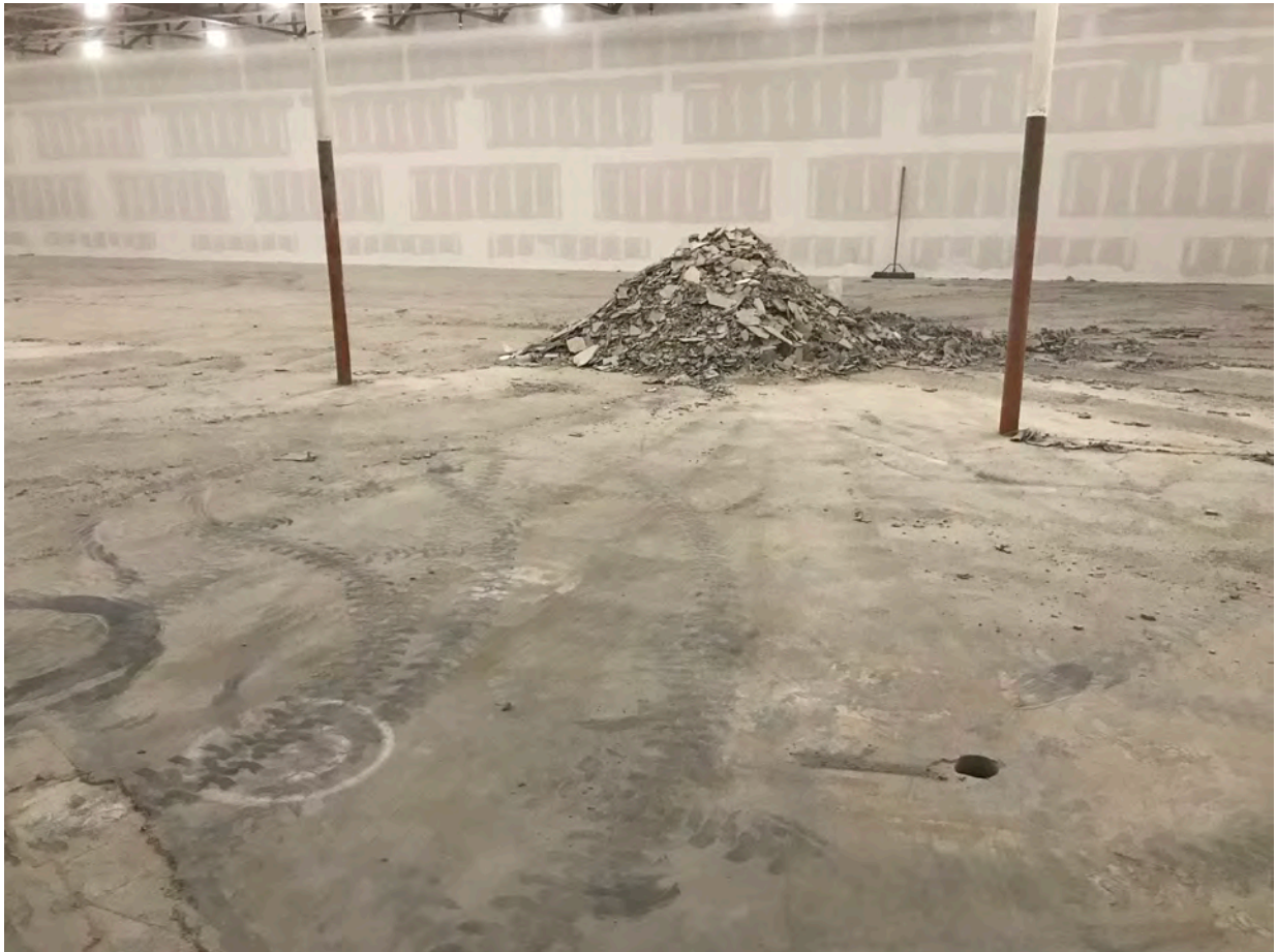
Removal of improper floor underlayment installation
