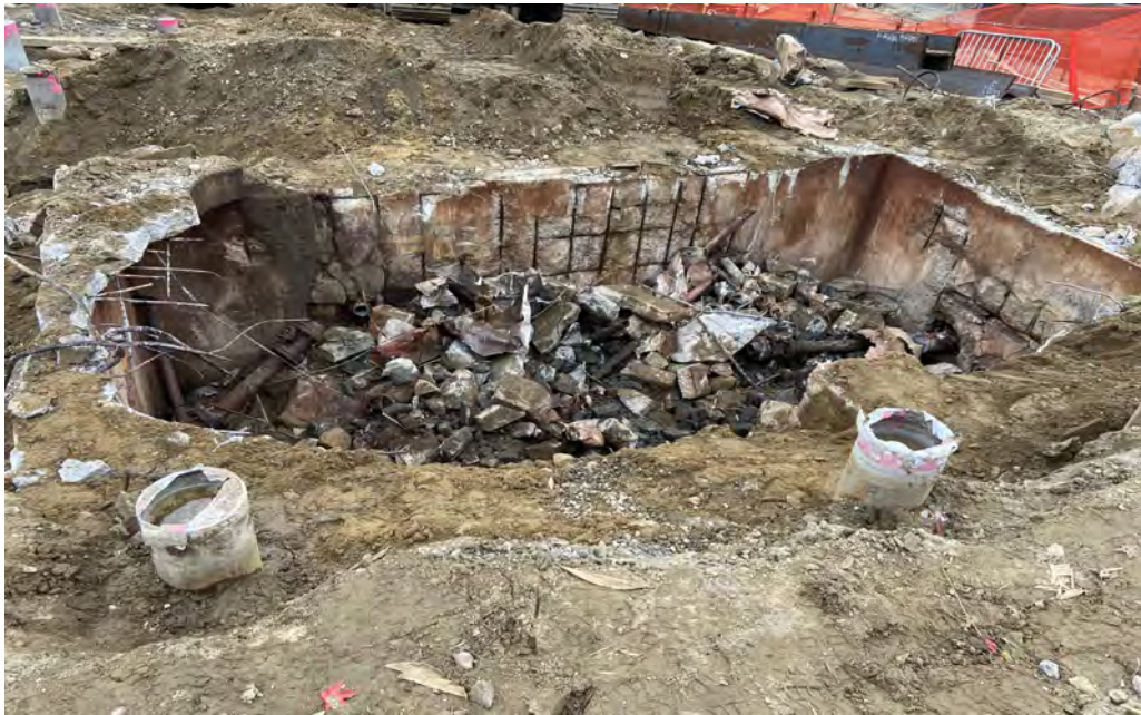
Demolition of the existing steam vault B4
