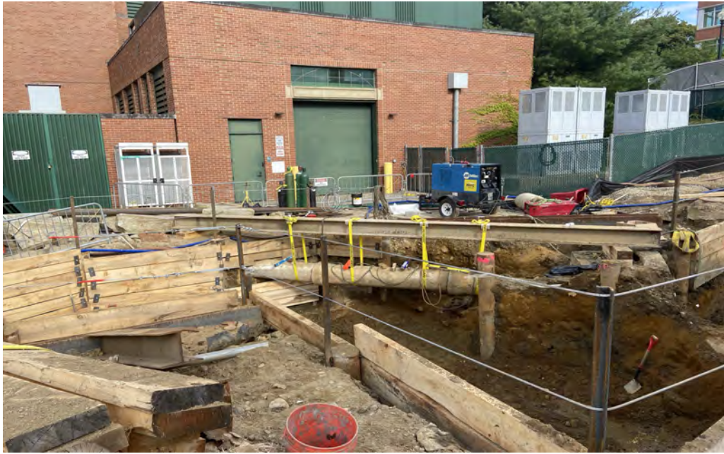
Steam excavation, piles and lagging, support existing piping
