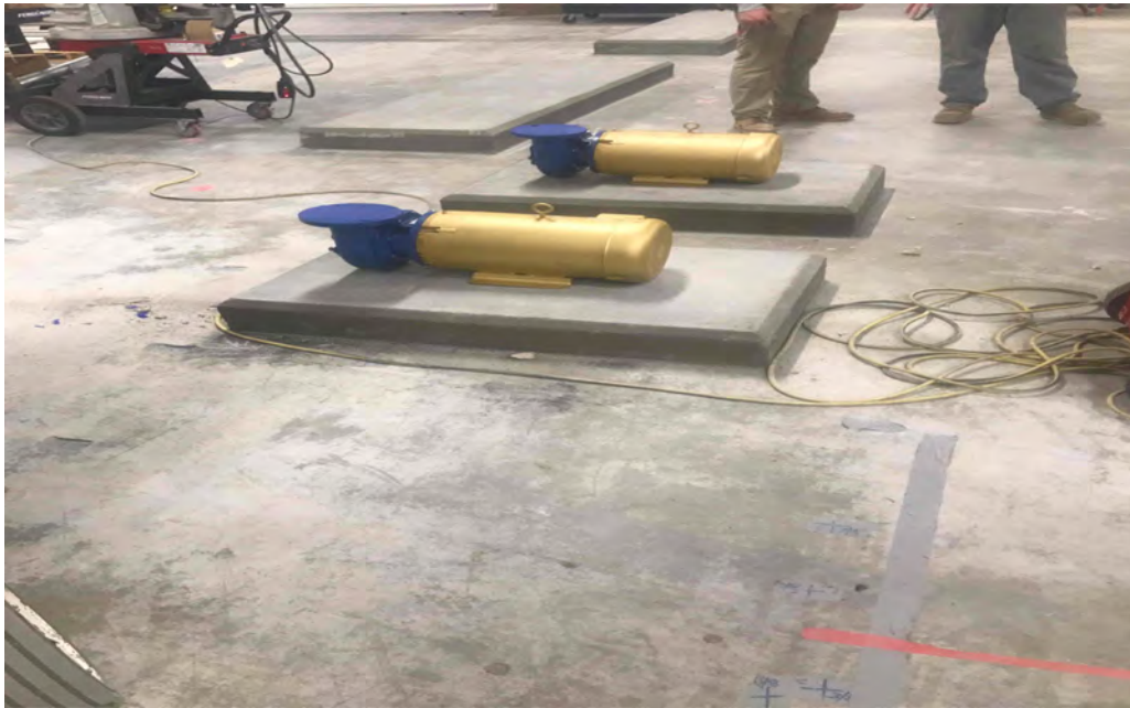
Condensate pumps set in place
