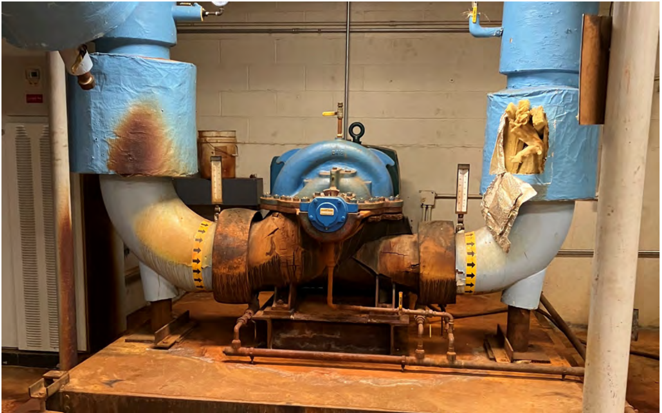
Existing Chilled Water Pump #4
