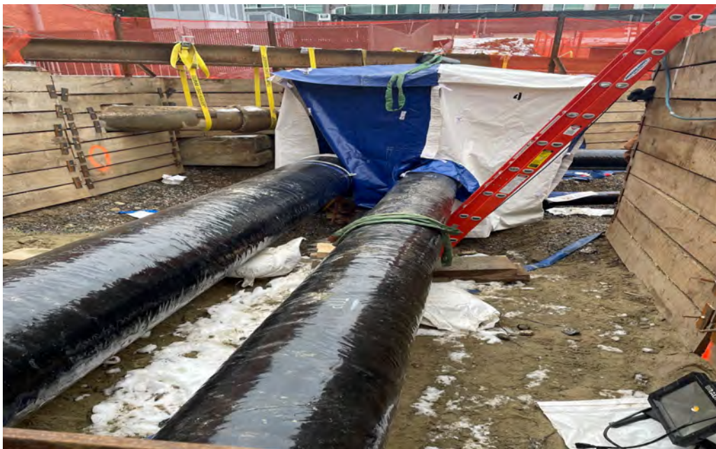
Perma-Pipe prefabricated steam & condensate pipe install
