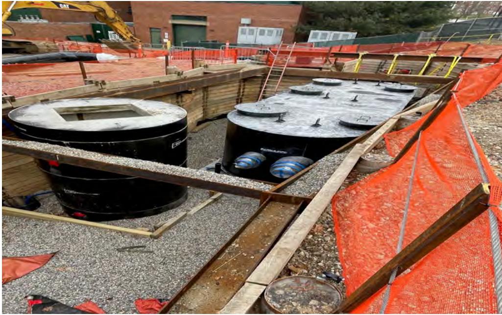
B4 vault steam vault in place ready for connections
