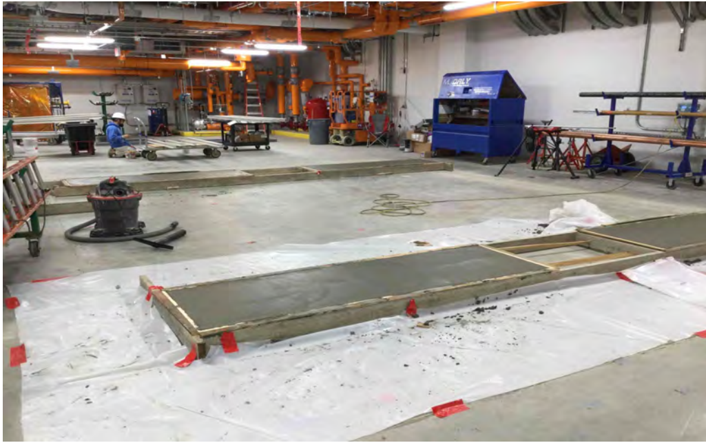
Condensate tank housekeeping pad placement at SUP
