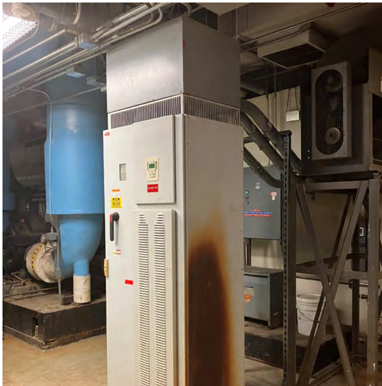
Relocated VFD from CWP#4 to CWP#1
