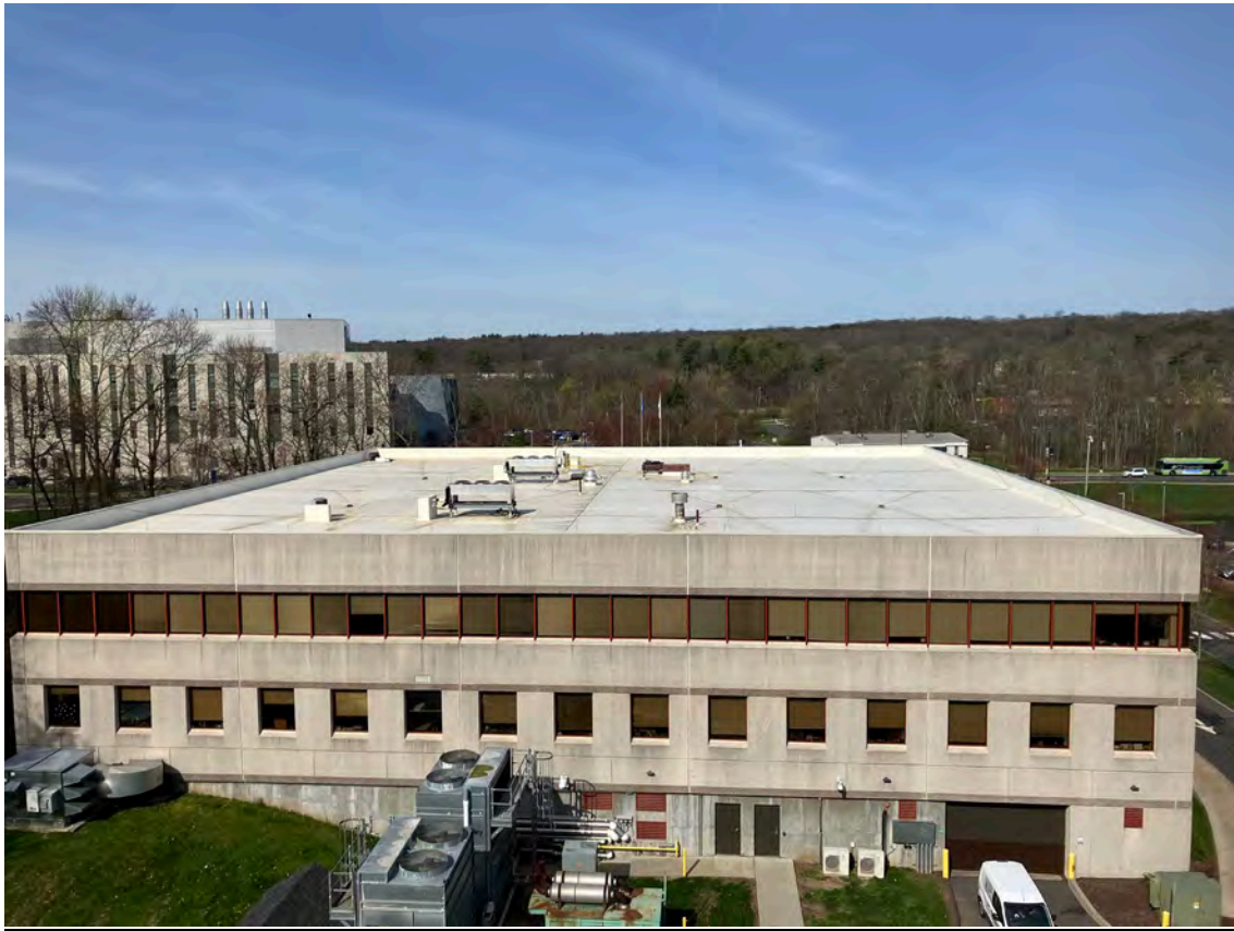
Substantially Complete Roof – Building D
