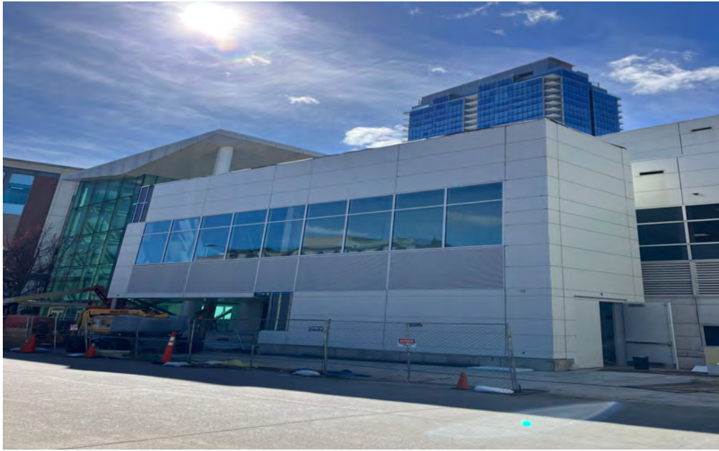
Progress photo of the new Southeast Emergency Egress Stair
