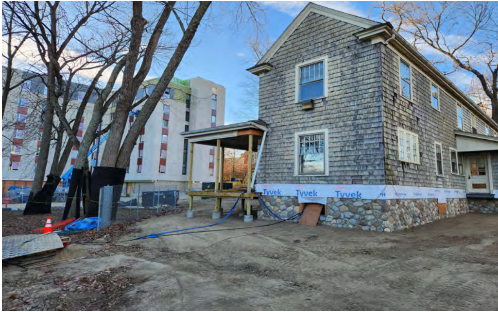
House stone veneer, foundation and backfill complete.
