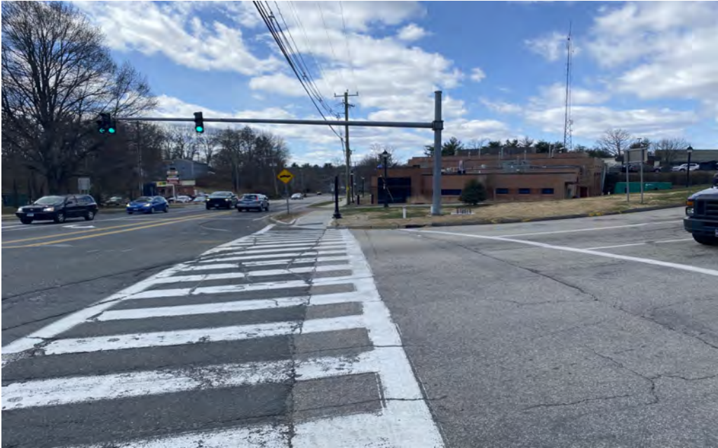
NW corner of NER and Discovery Dr - New Accessible Ramp
