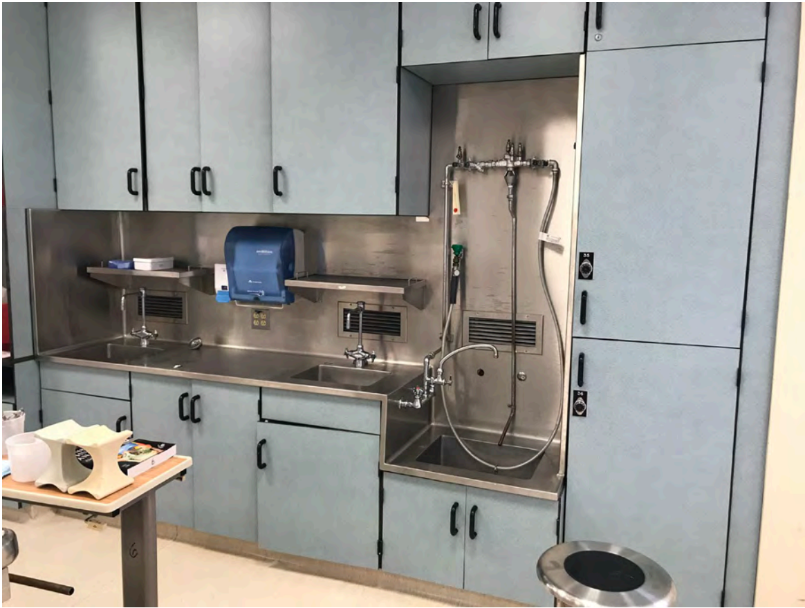
View of Existing Conditions in Lab
