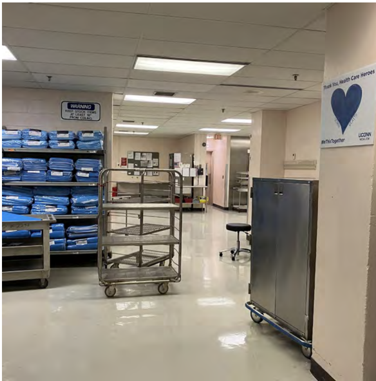
CB011D – Phase 2 Central Sterile before Demolition
