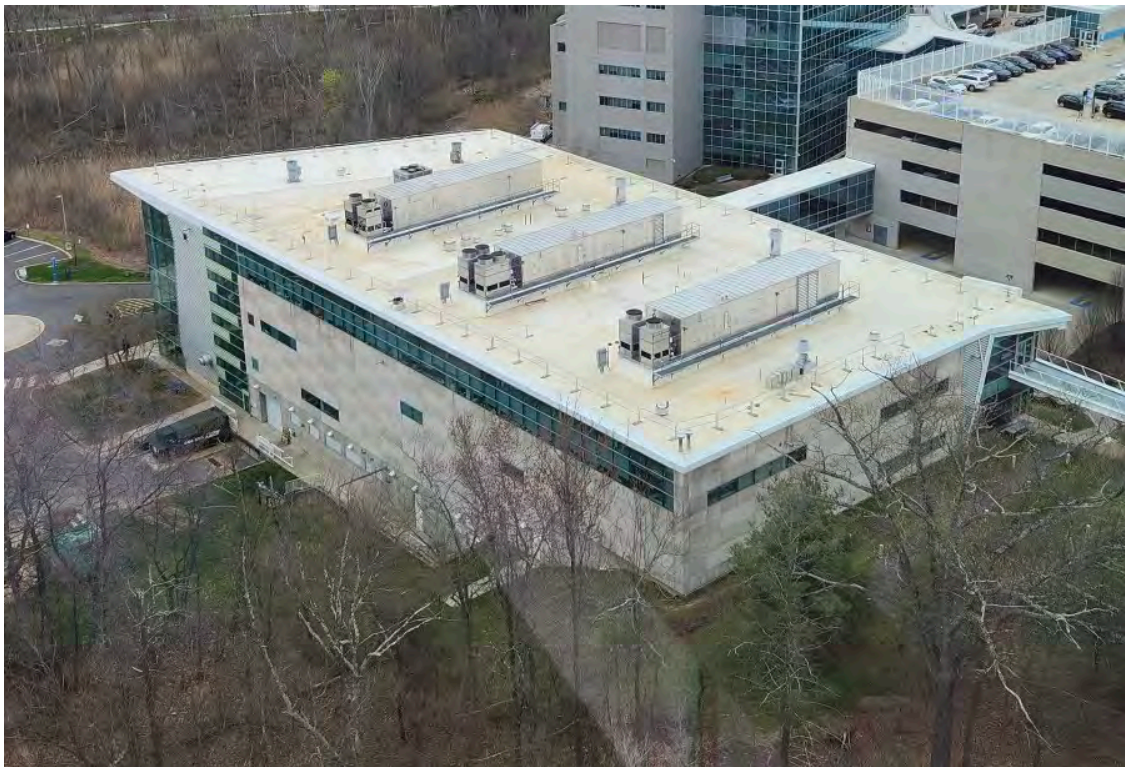
Substantially Complete Roof – Building N
