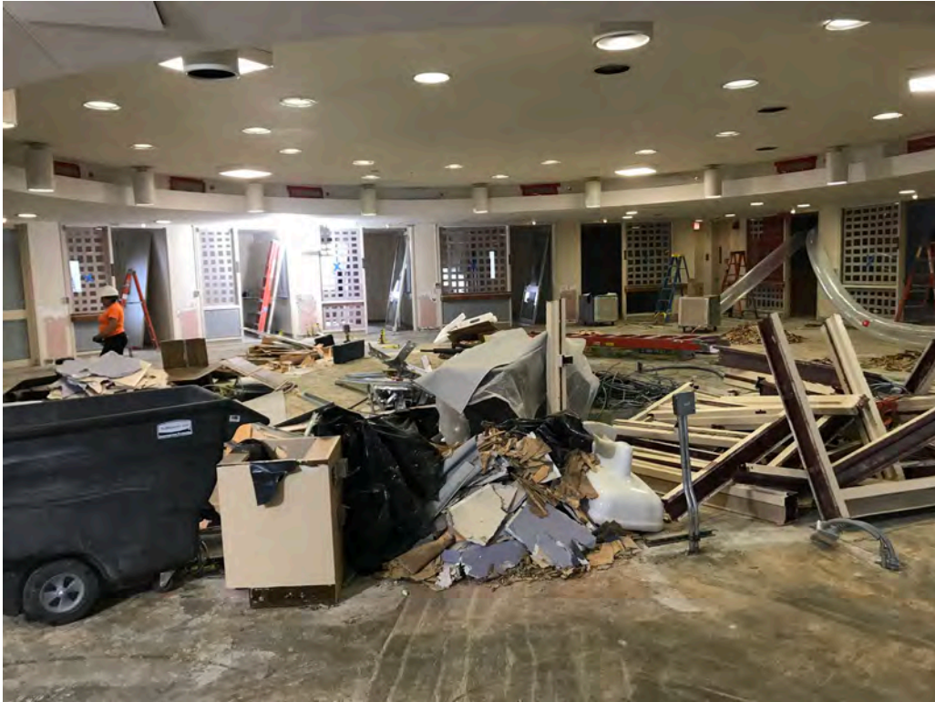
Demolition Work in progress
