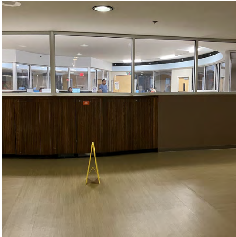
Nurse Station Enclosure – Window Frame to be modified for mesh along the top
