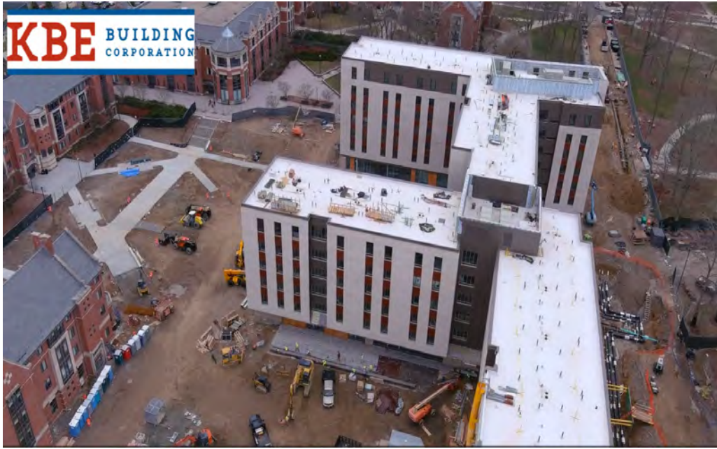
New Residence Hall - Area E and F - looking West
