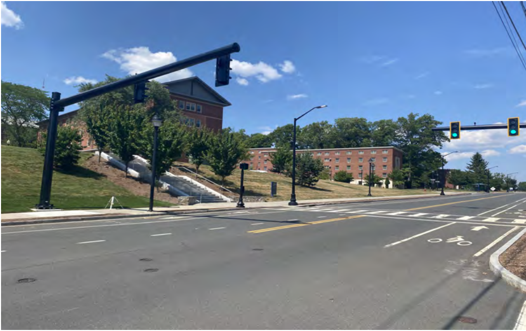
NER and Auditorium Dr - New Signals in Operation
