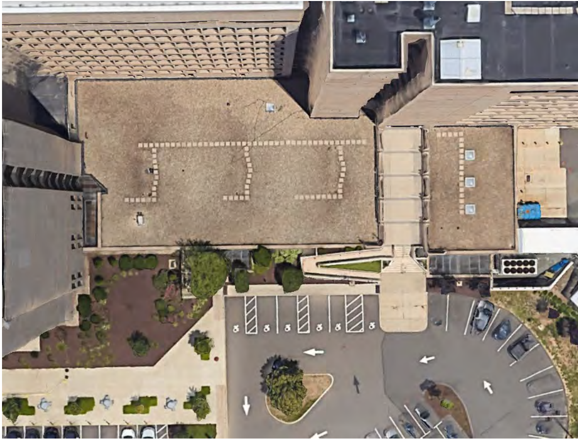
Existing Building K Roof
