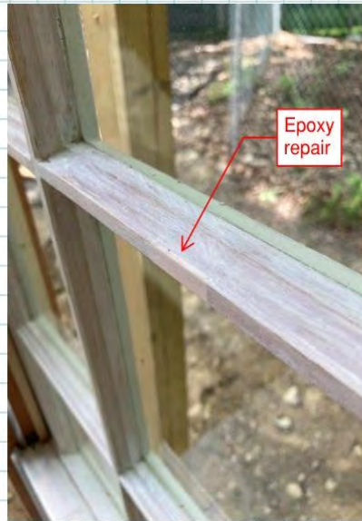
04 View of epoxy wood repair
