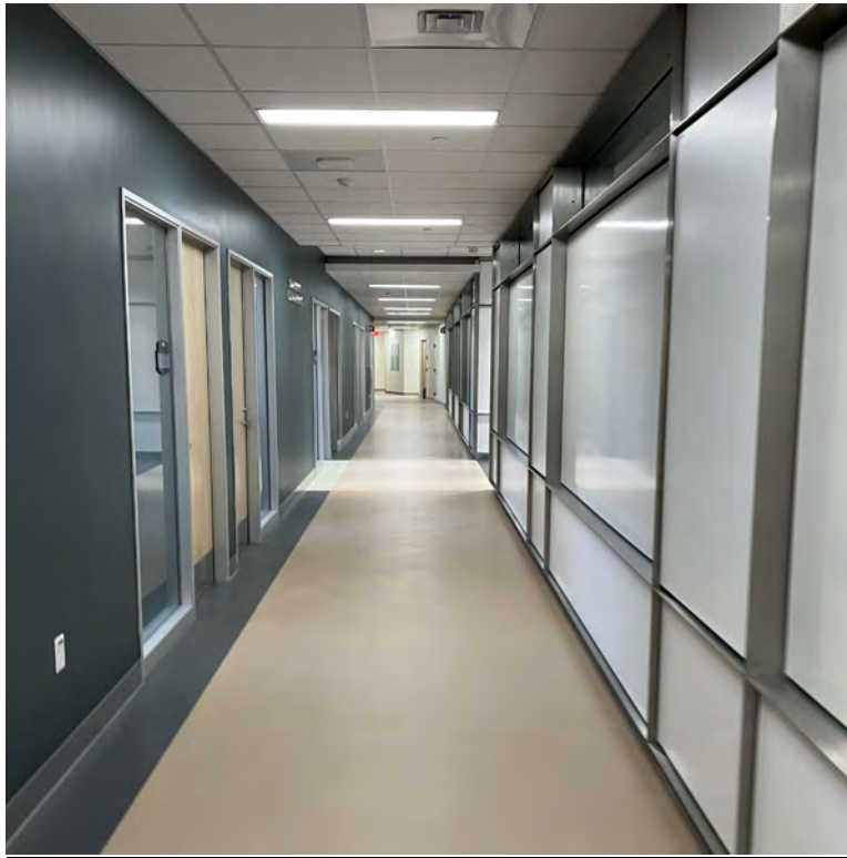
Completed Main Corridor
