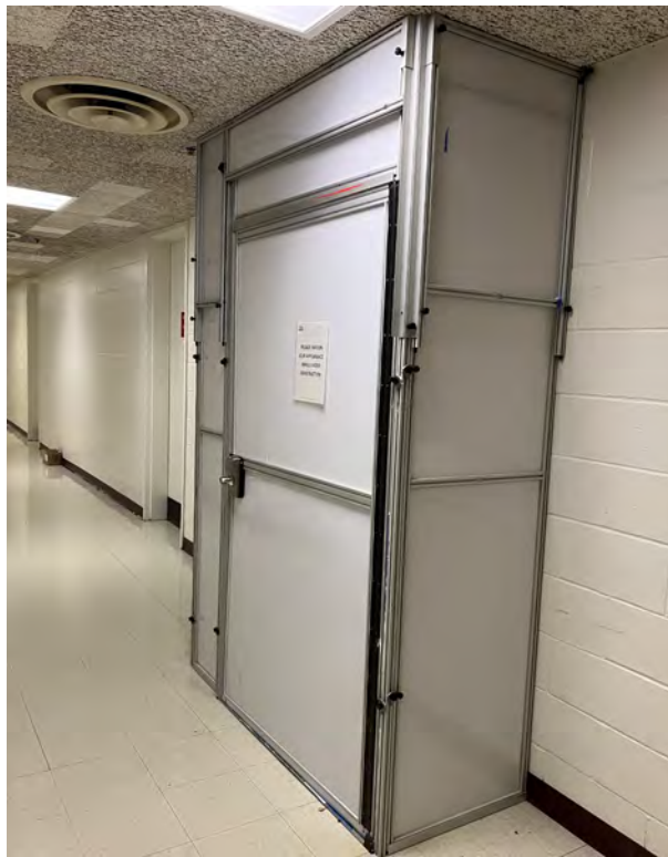
Phase 1 CG054 – Containment setup
