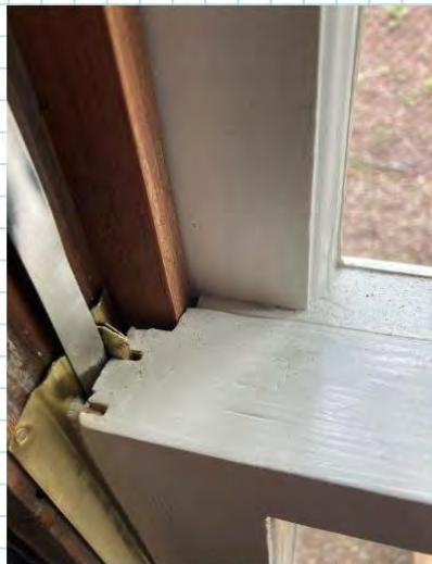
05 Metal weatherstripping in recommended location
