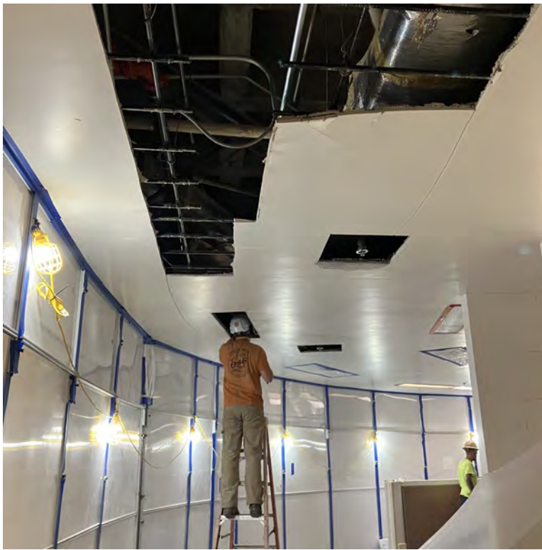
HB044 – Phase 1 Plaster Ceiling and Lighting Demolition
