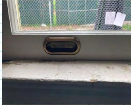
03 view of refurbished sash lift
