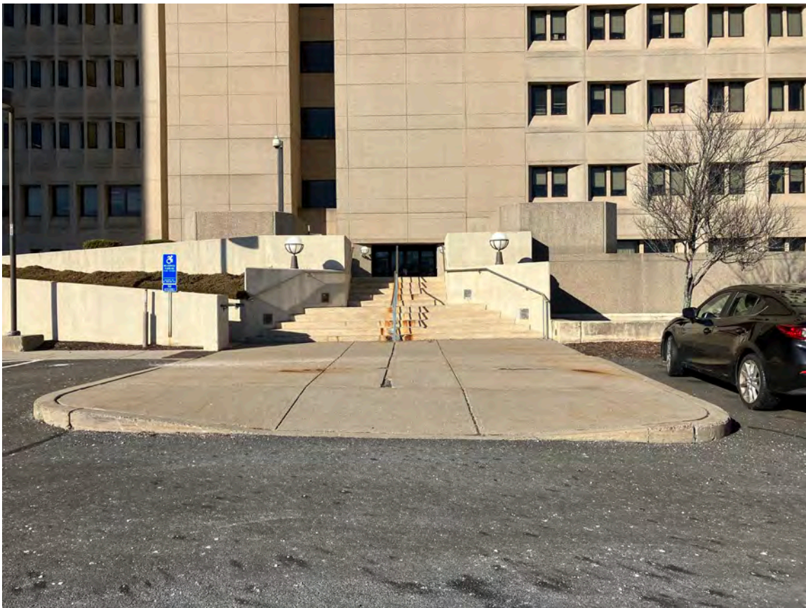
Existing Building E Entrance Walkway over Building K Roof
