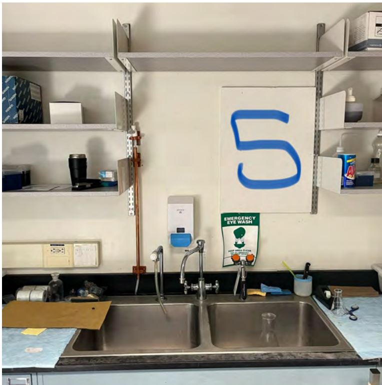
E5009 Millipore Install Location.
