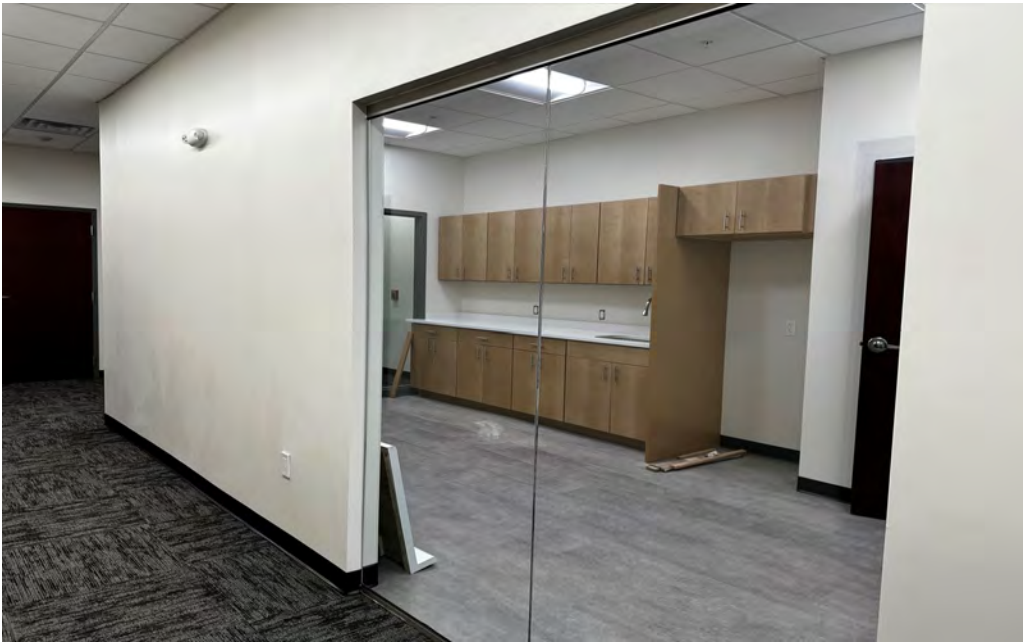
Waterbury progress photo kitchenette.
