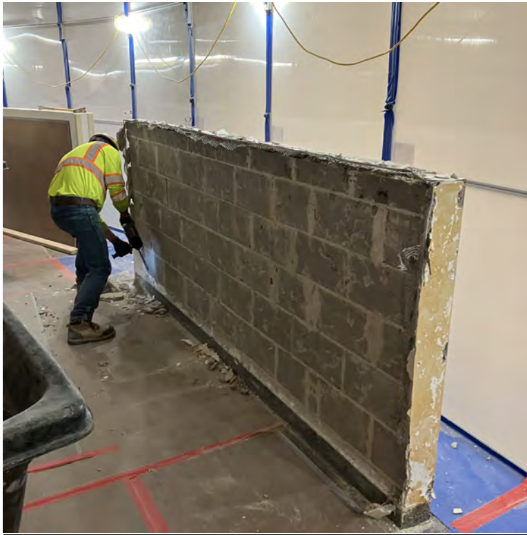
HB044 – Phase 1 Demolition of half walls
