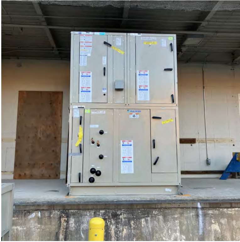
New CRAC Unit on the Loading Dock
