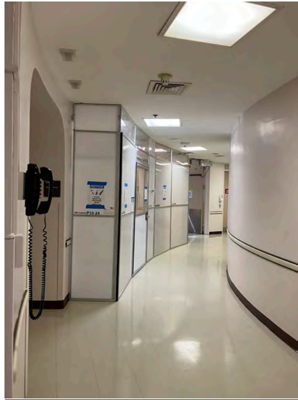
Infection Control Containment at Fluoroscopy Room
