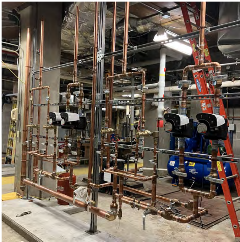
New Circulation Pump Station
