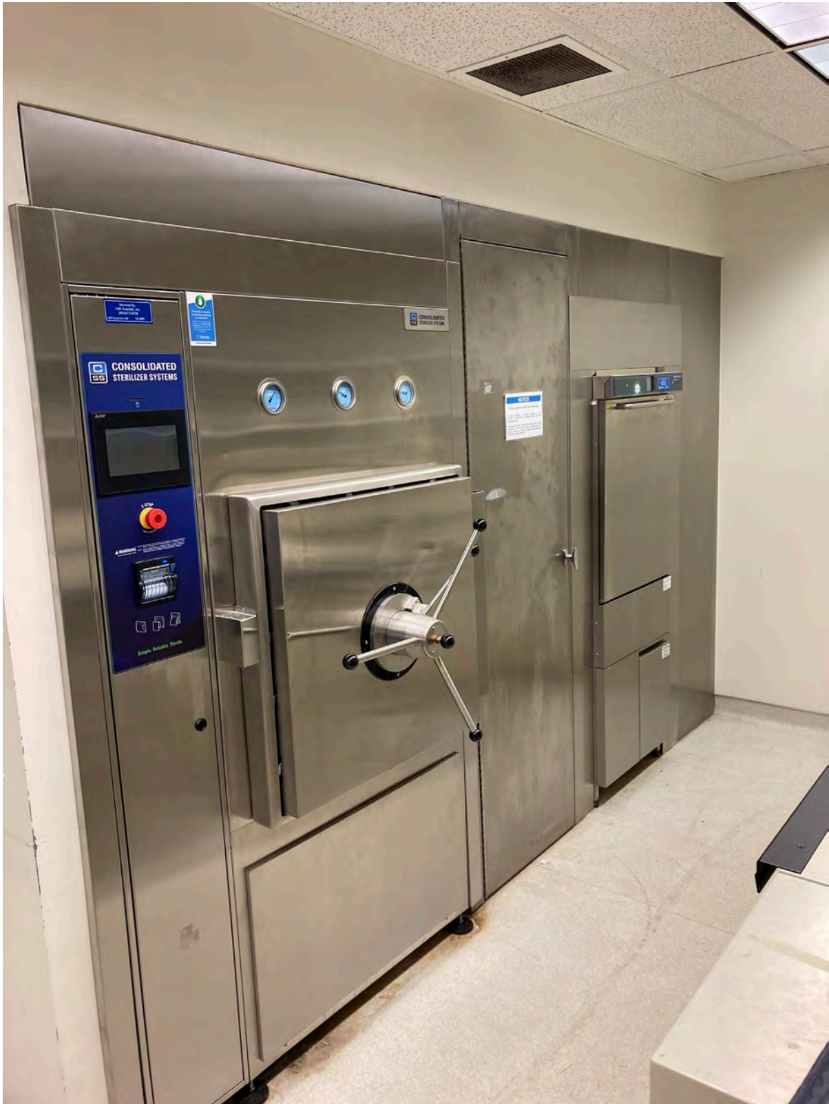
Typical ARB Consolidated Sterilizer & Lancer Glasswasher Installation
