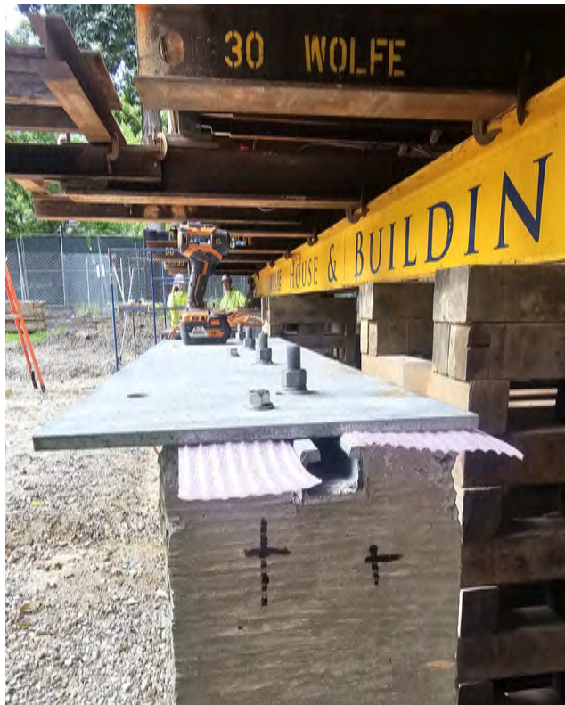
Foundation and metal plate to support the house sill.
