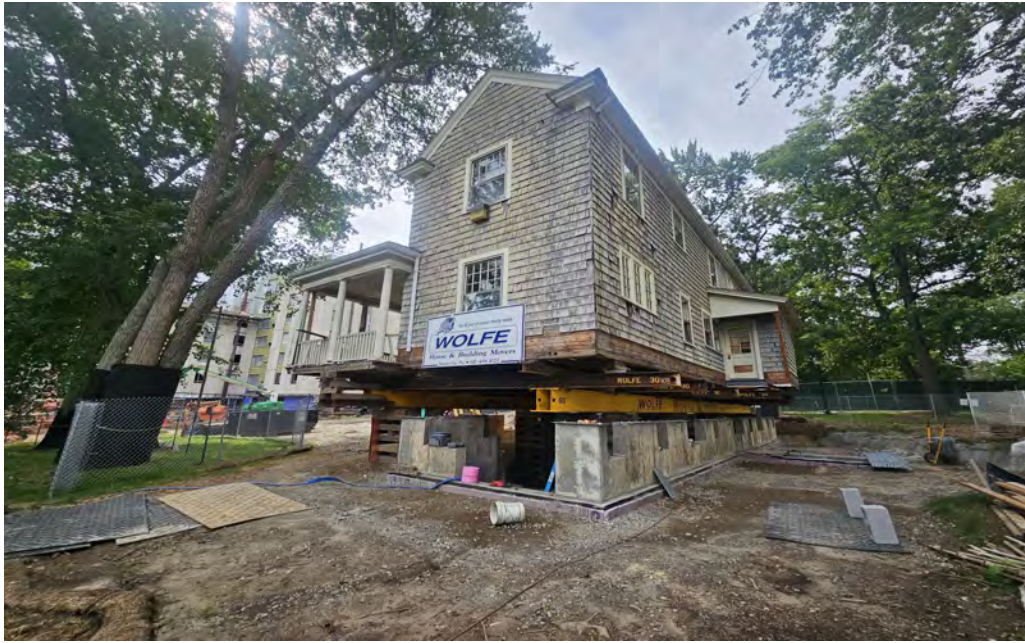
House at permanent site hovering over foundations.
