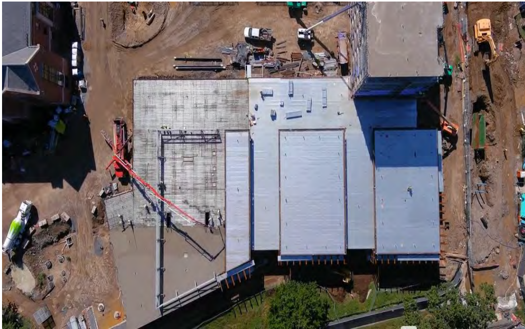
Top view Area G (Dining Hall)-Concrete roof pour in progress
