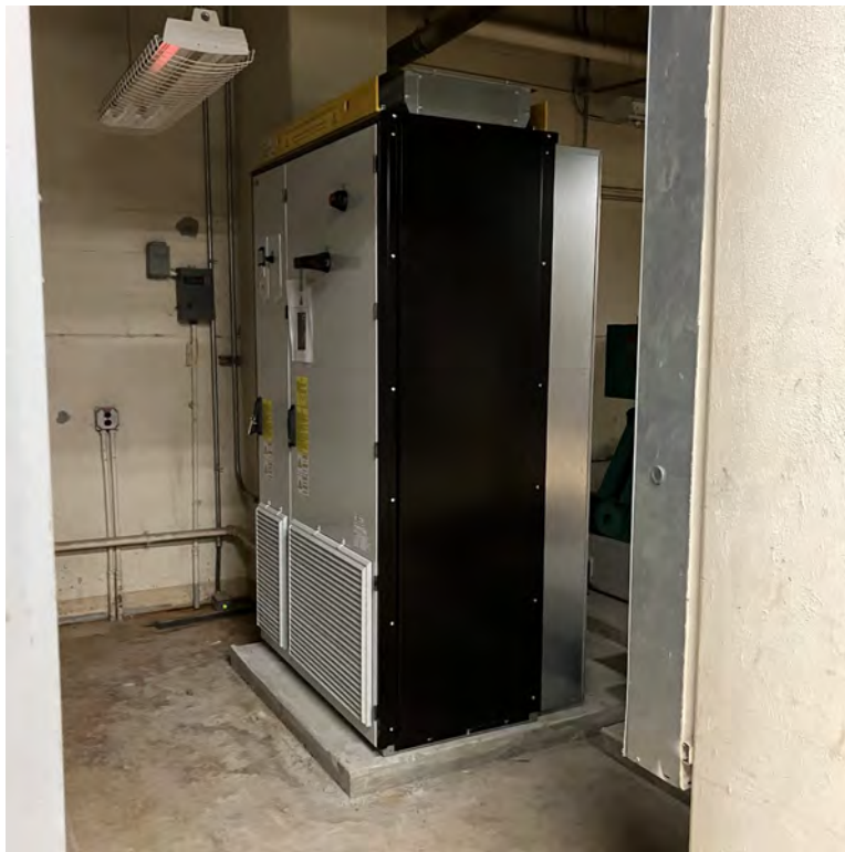
New VFD for Chilled Water Pump #4
