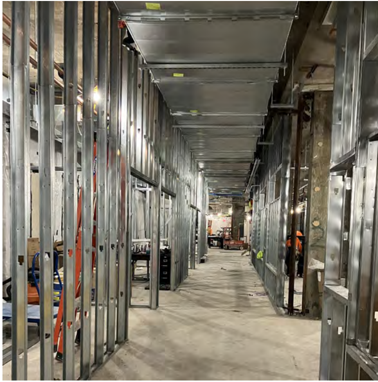
New Ductwork and Framing
