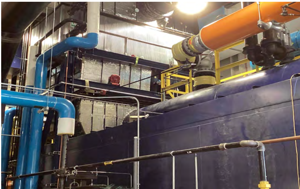
Boiler economizer insulation installation
