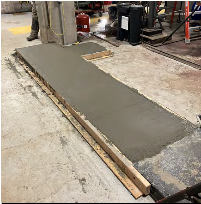
New Circulation Pump Station Equipment Pad
