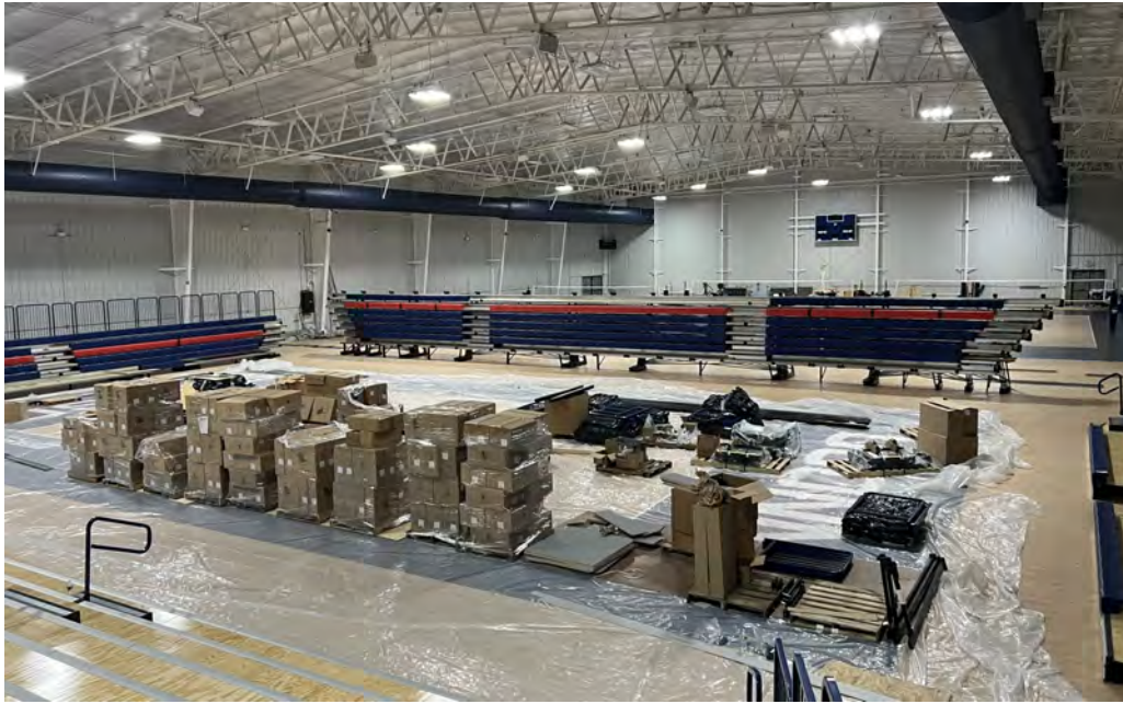
Volleyball Arena - Bleacher Installation
