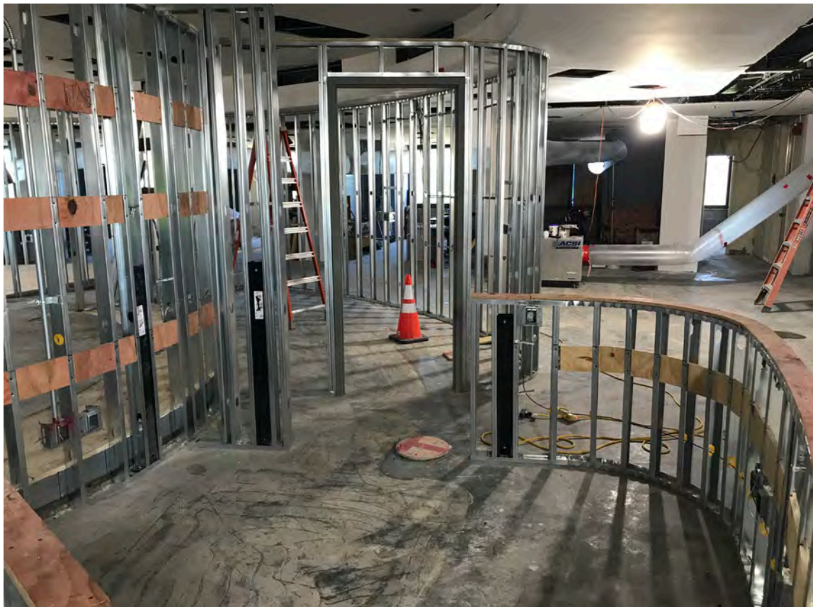
New Metal Framing at Low Wall Nurse Station Area
