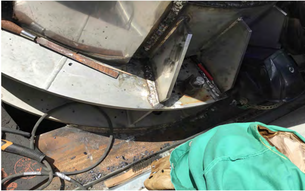
SUP boiler stack support modifications
