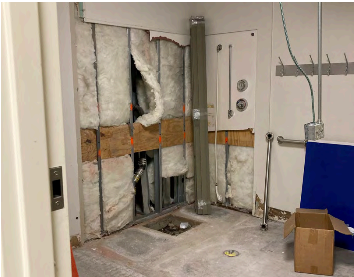
N1016 Existing Shower has been demolished
