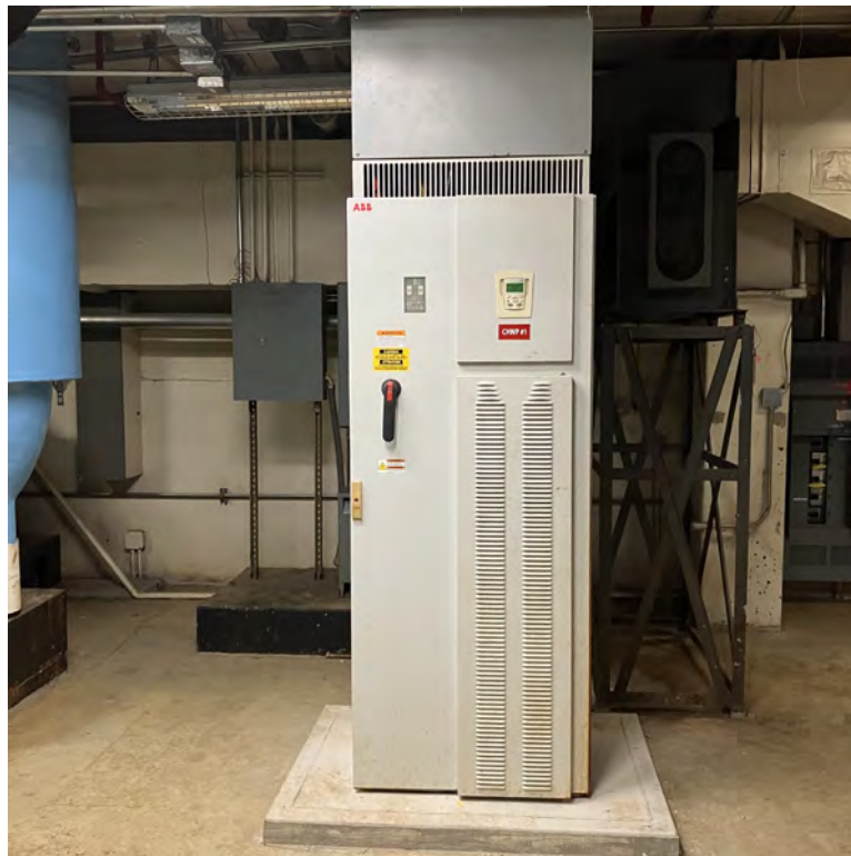
Relocated VFD from CWP#4 to CWP#1
