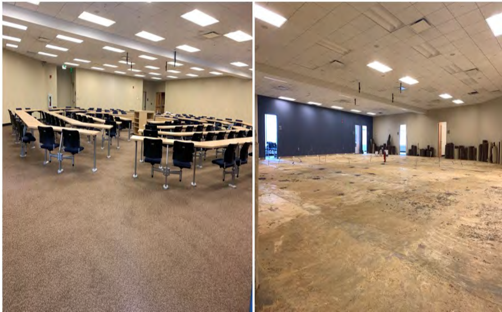
Room 302 existing Lecture Hall before and after demo
