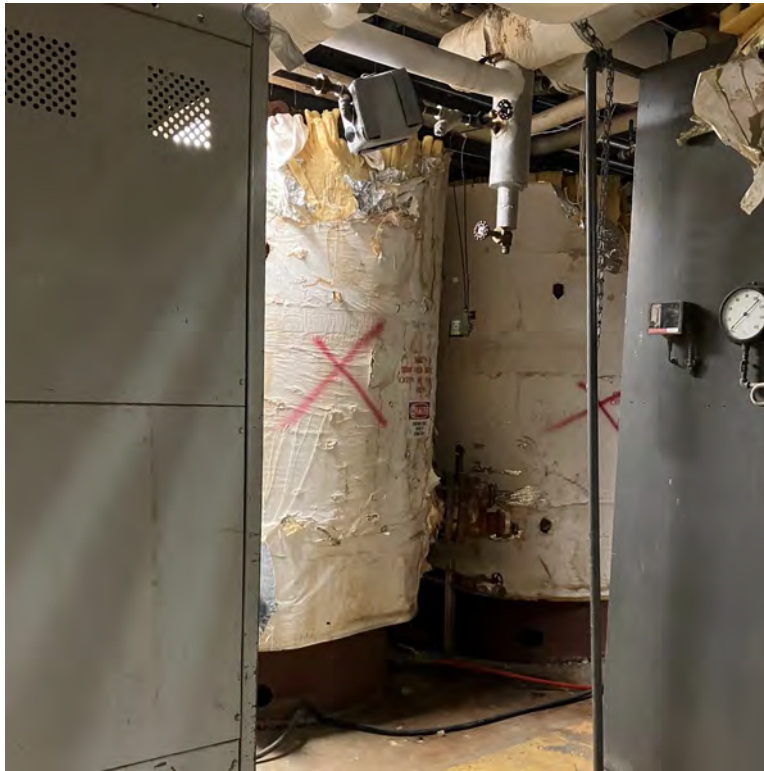
Existing Hot Water Storage Tanks to be Removed
