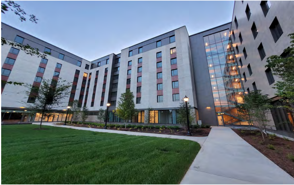
Connecticut Residence Hall - Courtyard
