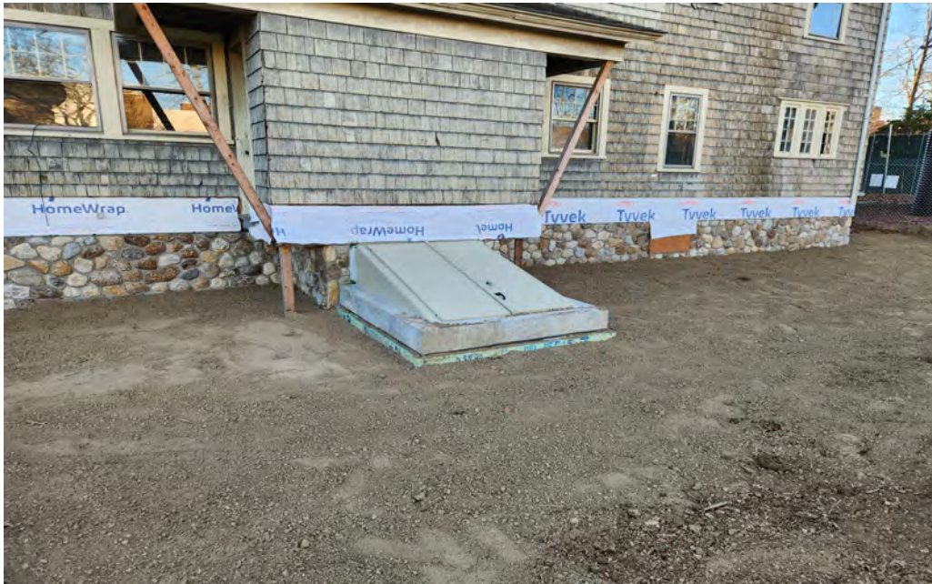
House stone veneer, foundation and backfill complete.
