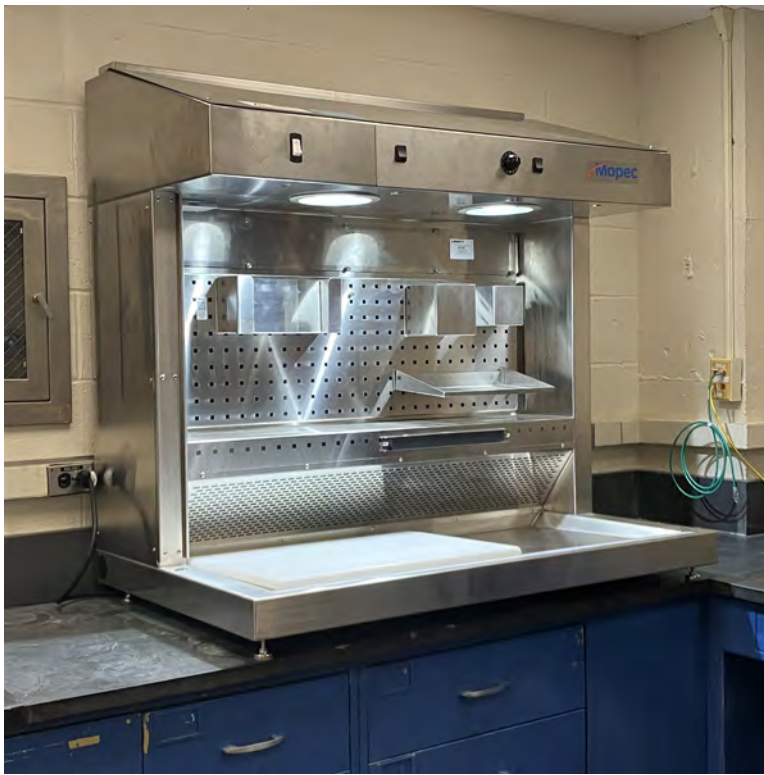
CG047 – Installed New Countertop Grossing Station
