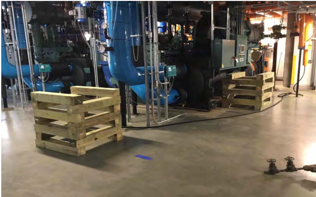
Cribbing being assembled for July steam blow
