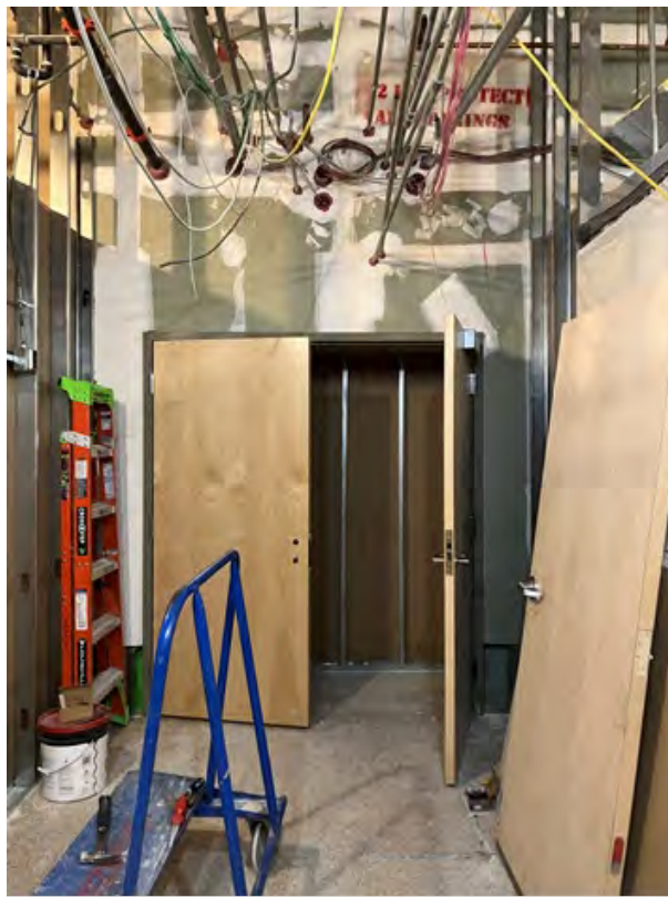
HM003A – Construction of Temporary Bathroom and Corridor
