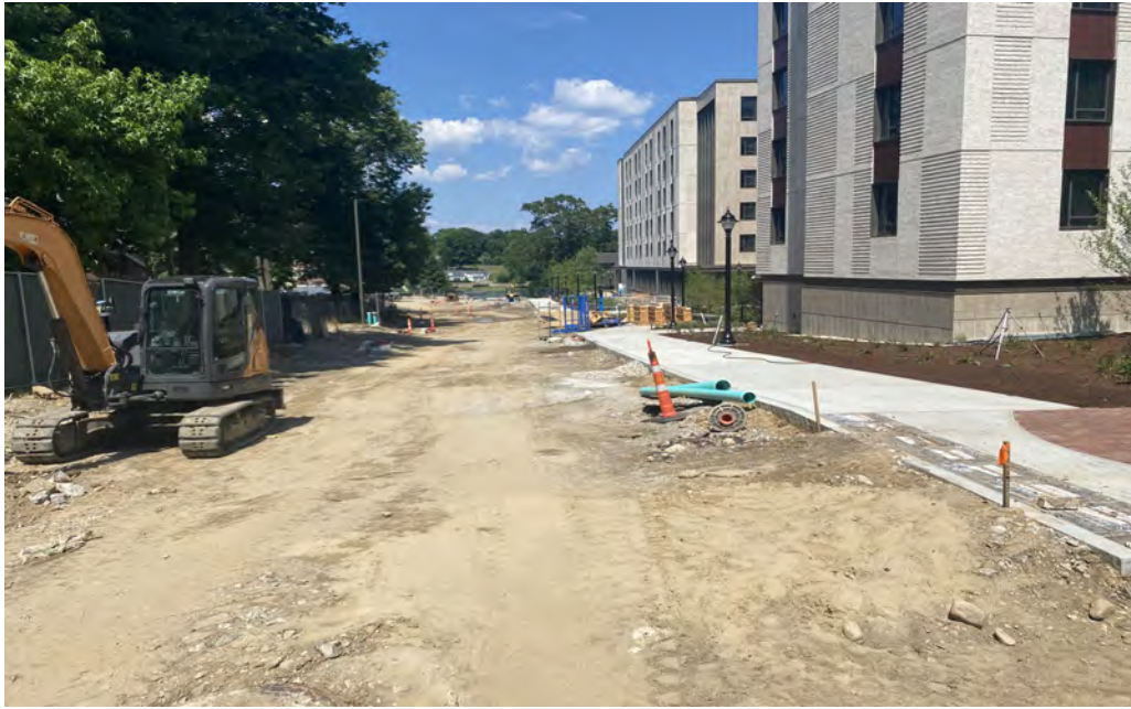
Gilbert Road Looking East - Finishes starting (Package 1)
