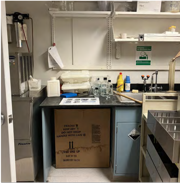
EG047 DI Water Connection Needed
