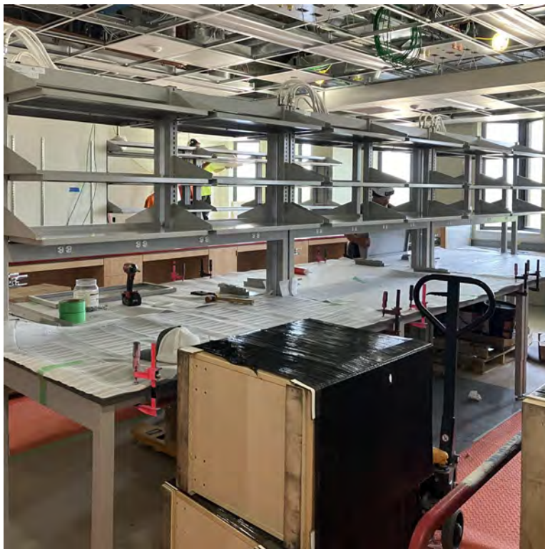
Installation of Lab Casework in Open Lab L2078
