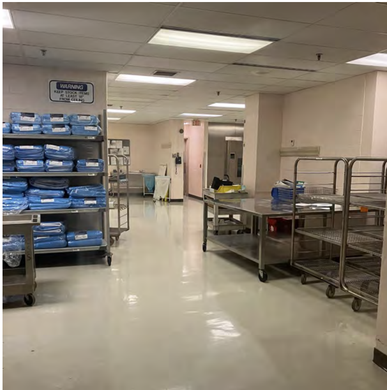
CB011D – Phase 2 Central Sterile before Demolition
