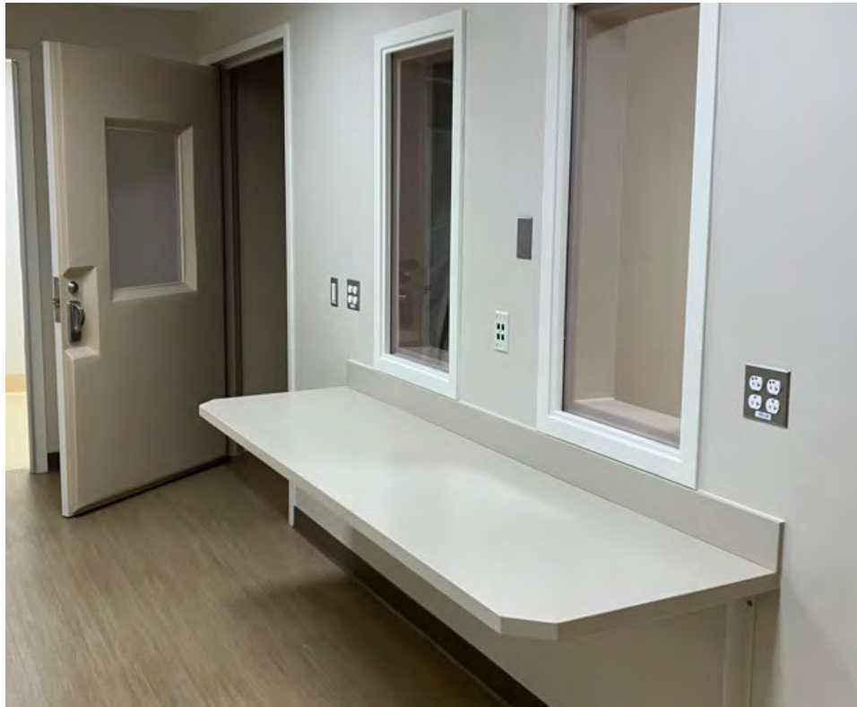
Nurse Station Enclosure – Window Frame with Mesh Installed
