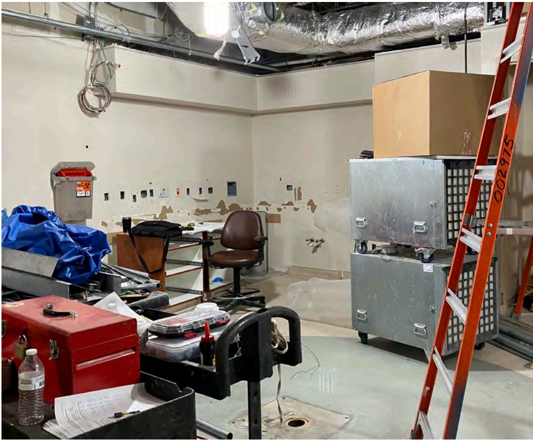
Cath Lab 1 - Demolition
