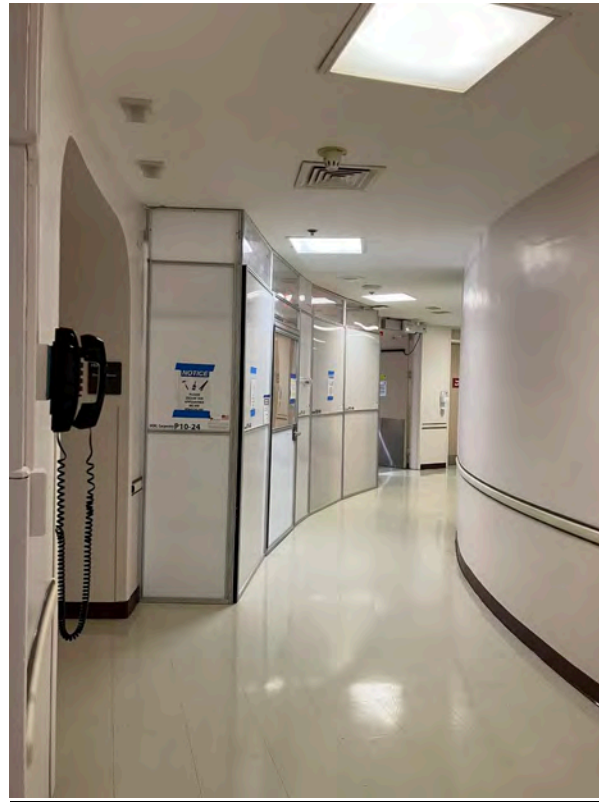
HM043 – ICRA Containment at Fluoroscopy Room
