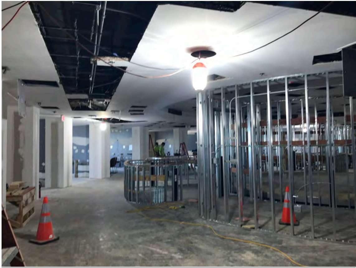
New Metal Framing at Nurse Station area
