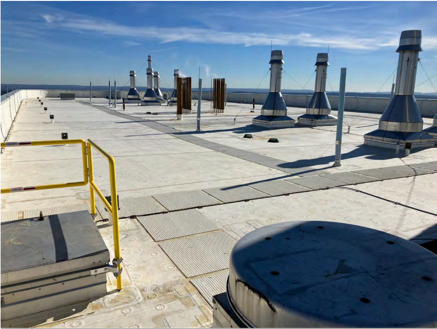
Completed Roof – Building E
